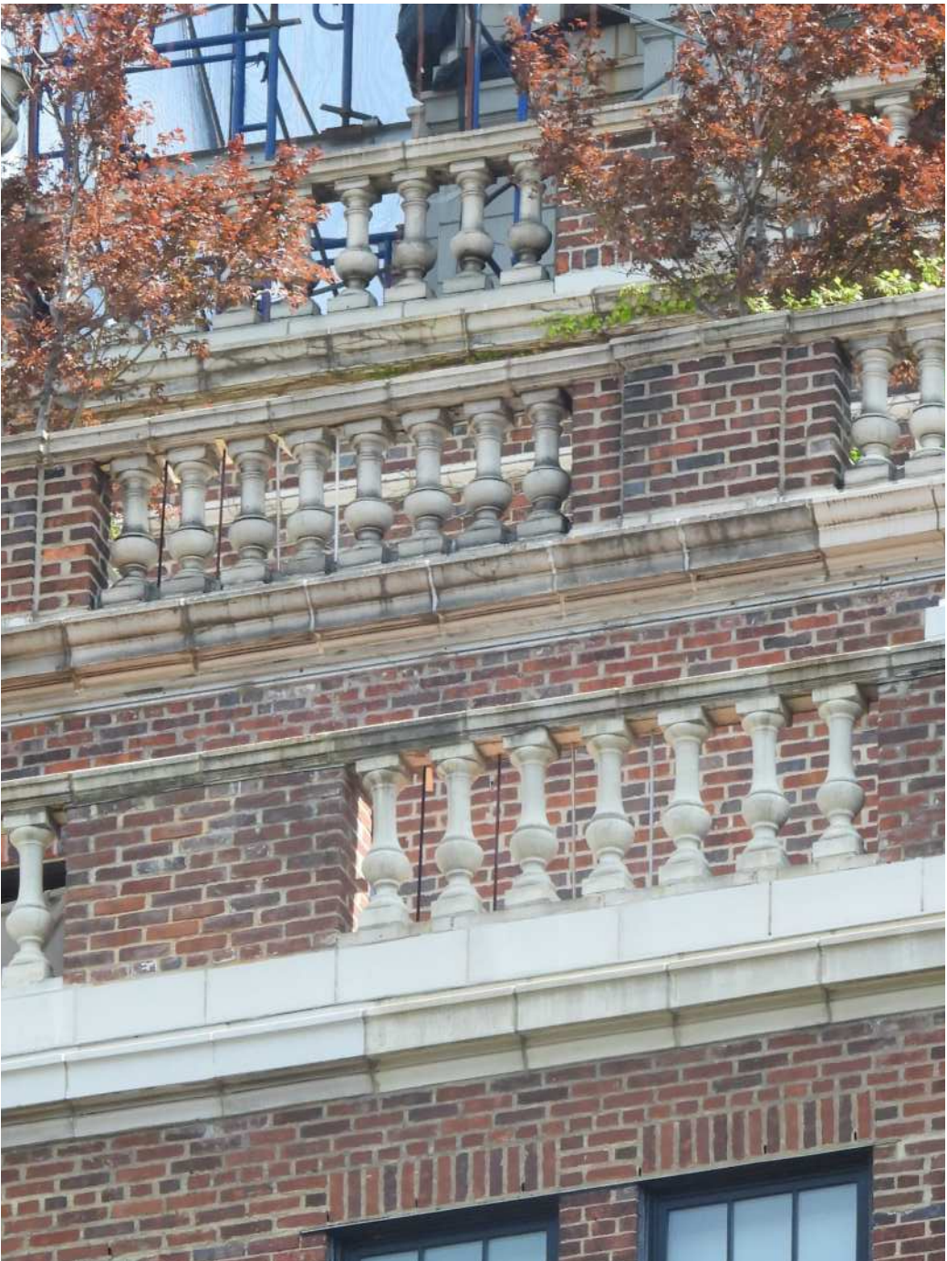
VISUAL MOCK-UP OF PROPOSED METAL ROD BETWEEN BALUSTERS AT PENTHOUSE PARAPET UPPER & LOWER LEVELS
