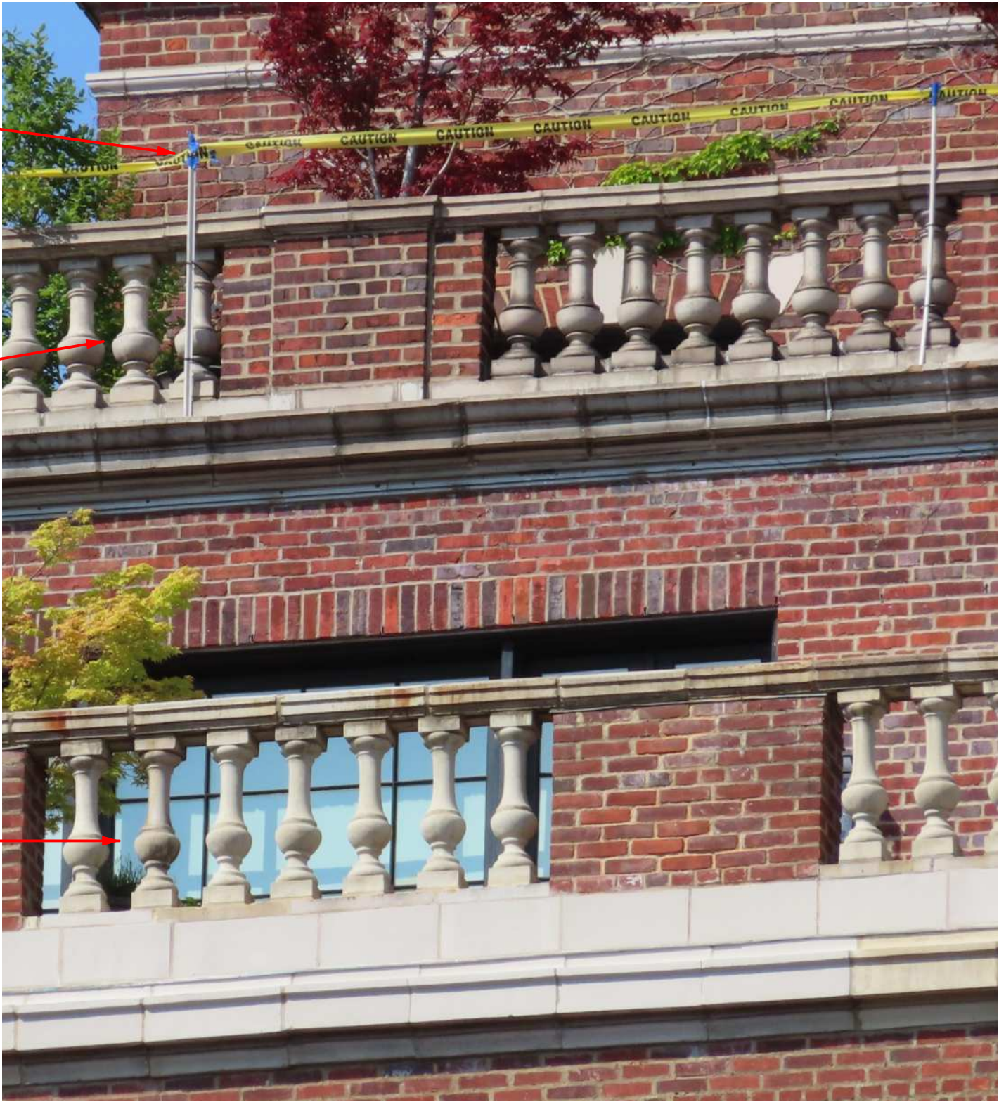
CLOSE-UP PHOTOGRAPHS OF EXISTING BALUSTERS, BASE UNITS AND WATER TABLES AT THE UPPER AND LOWER TERRACES FOR REFERENCE
