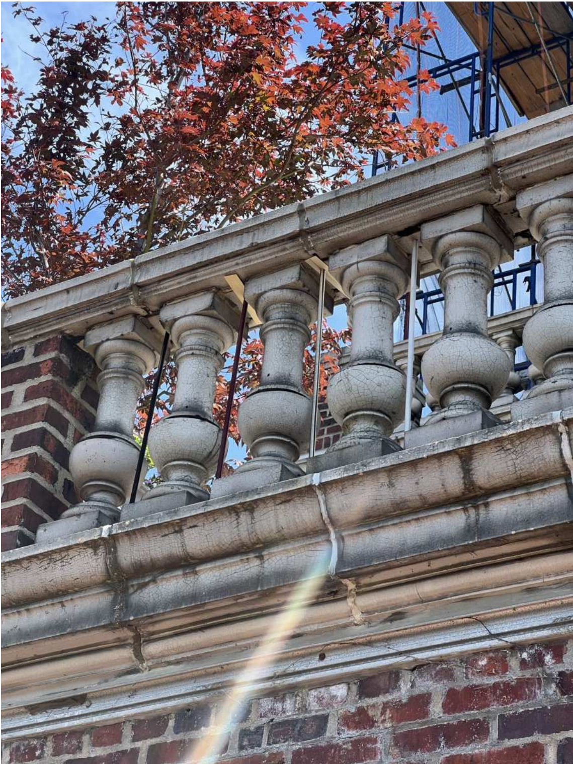
VISUAL MOCK-UP OF PROPOSED METAL ROD BETWEEN BALUSTERS AT PENTHOUSE PARAPET UPPER LEVEL EXTERIOR
