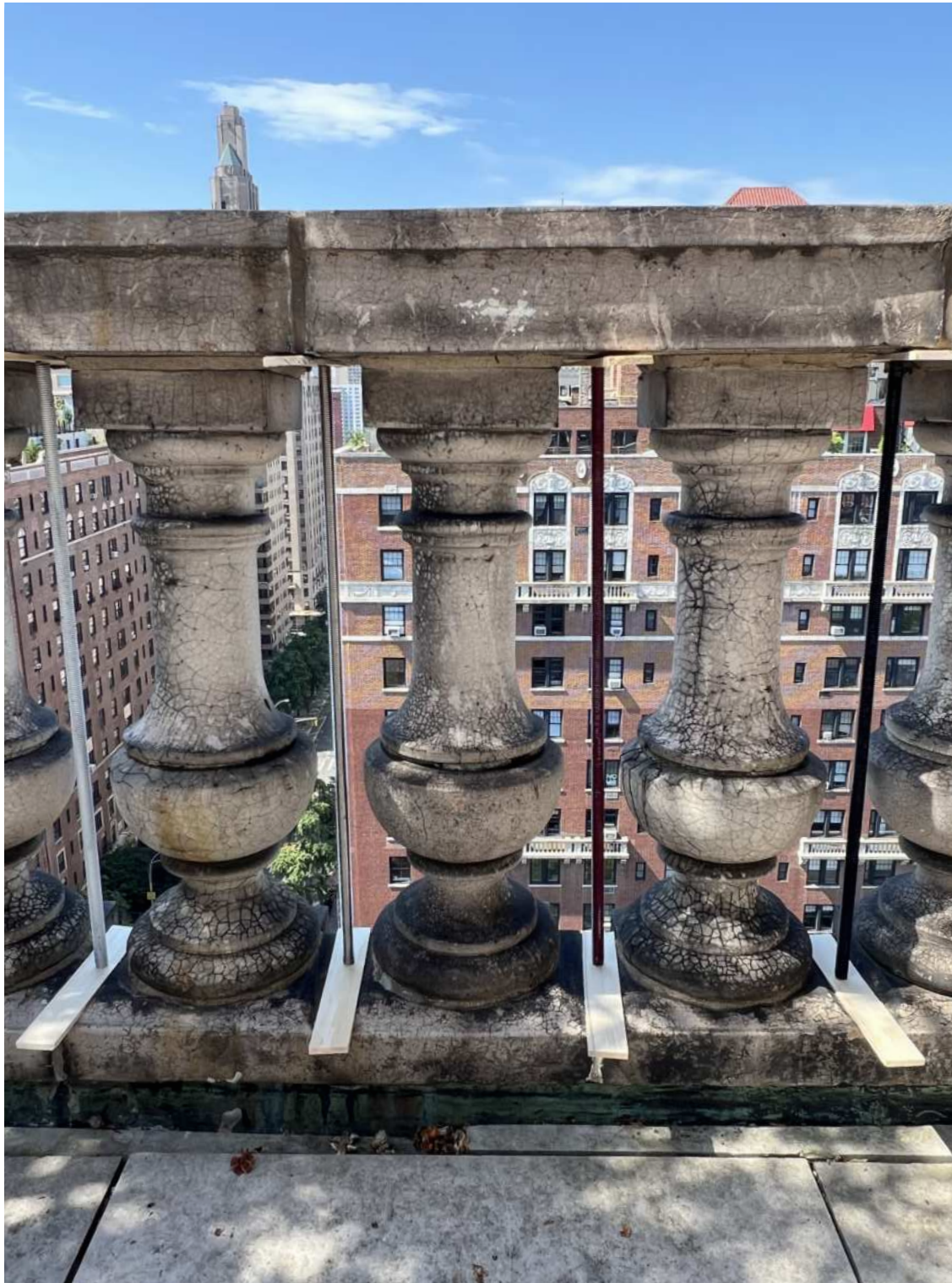
VISUAL MOCK-UP OF PROPOSED METAL ROD BETWEEN BALUSTERS AT PENTHOUSE PARAPET UPPER LEVEL INTERIOR
