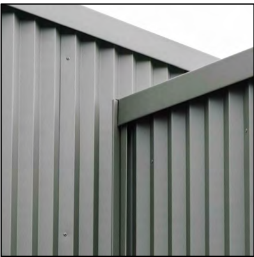
ZINC CLADDING: RHEINZINK PREPATINA GRAPHITE GREY, ZIGZAG PROFILE
