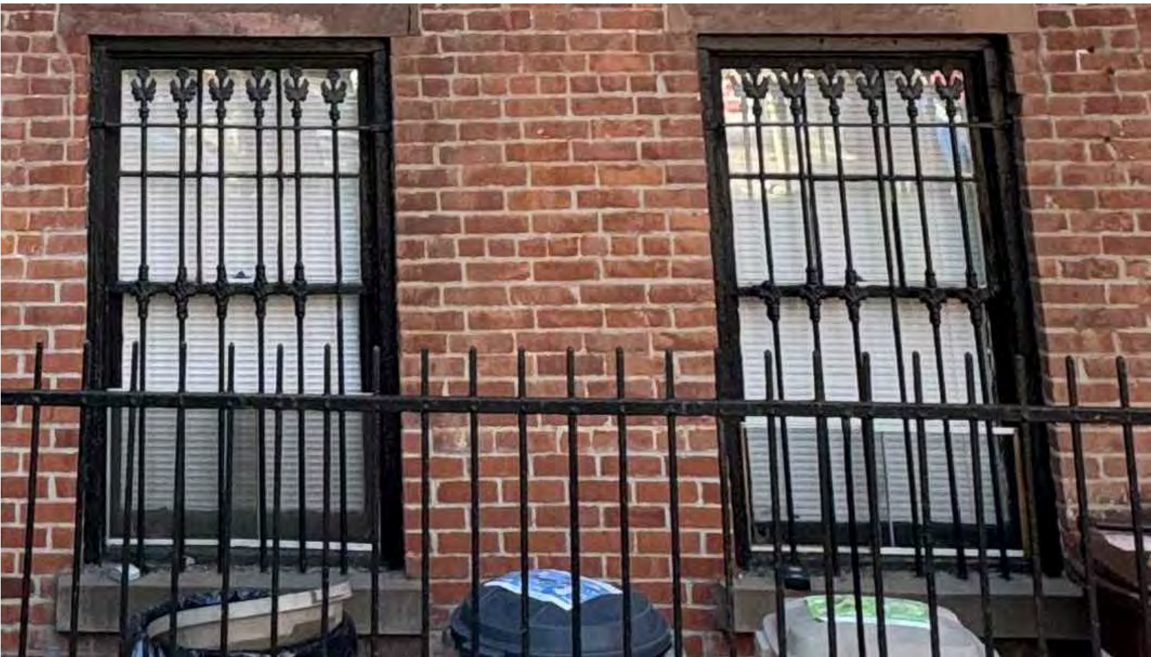
CAST IRON WINDOW BARS EAST FACADE AND EASTMOST WINDOW ON NORTH FACADE, BASEMENT LEVEL
