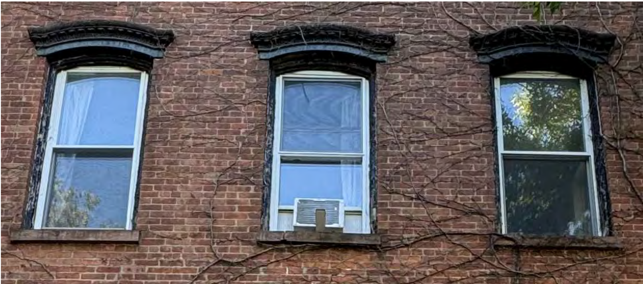
CAST IRON WINDOW LINTELS EAST FACADE, 2ND FLOOR
