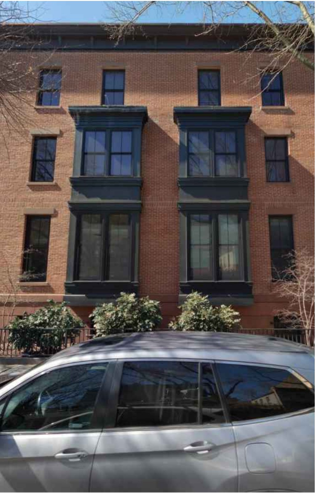
332 ADELPHI ST. FORT GREENE HISTORIC DISTRICT SQUARE PROFILE PRESSED METAL DOUBLE ORIEL WINDOWS, INTERSECTS BROWNSTONE BASE AND BANDCOURSE
