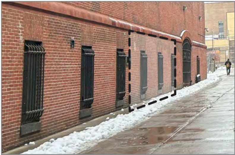
EXISTING PUNCHED WINDOW MASONRY OPENINGS TO BE EXPANDED INTO ONE LARGER ENTRANCE
