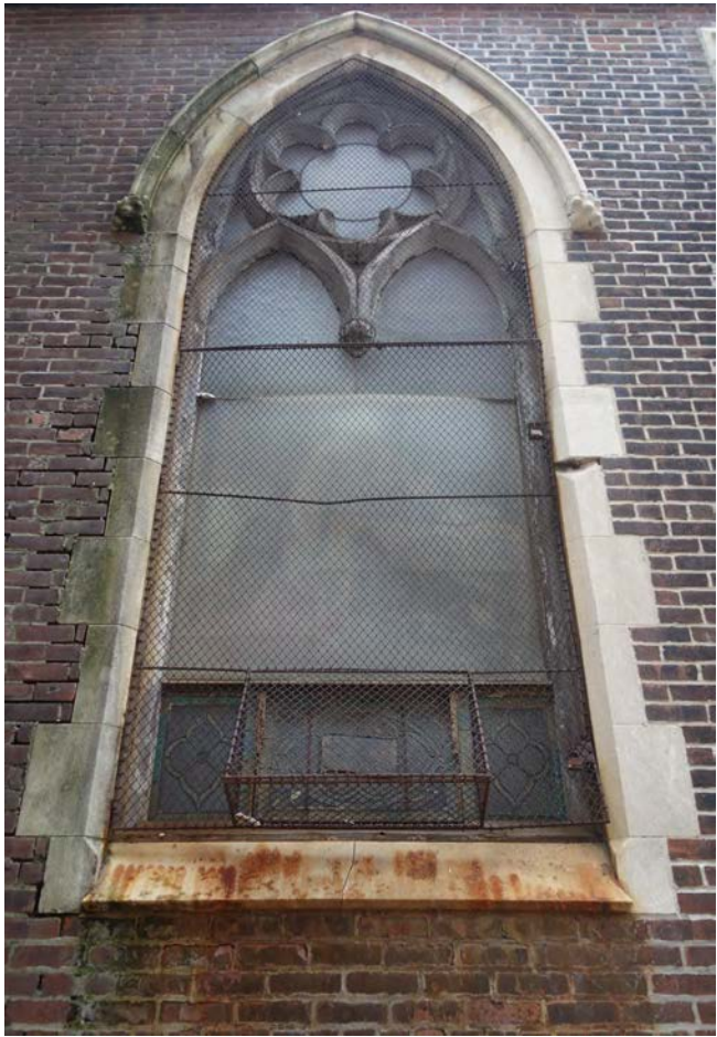
CHURCH SOUTH FACADE - NAVE MASONRY OPENING AND WOOD TRACERY (TYP. OF 2), EXT.
