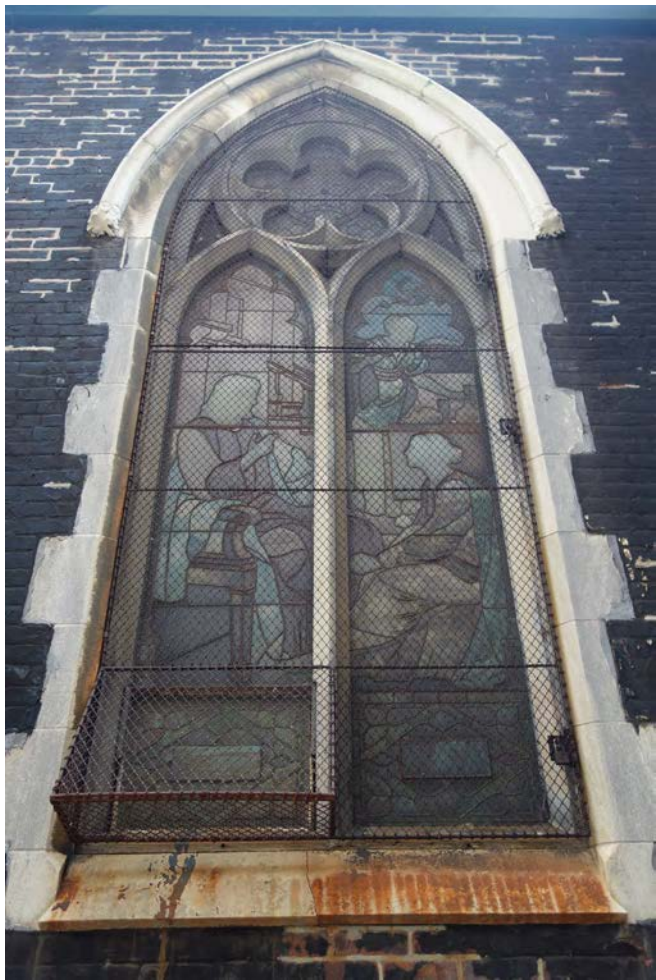
CHURCH NORTH FACADE - NAVE STAINED GLASS MASONRY OPENING AND WOOD TRACERY, EXT.
