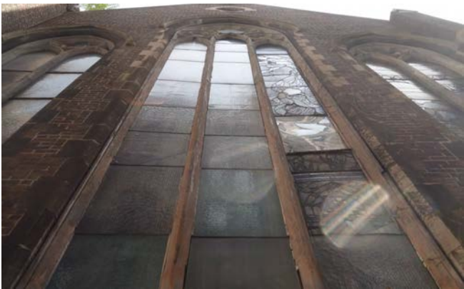
CHURCH NORTH FACADE - TRANSEPT STAINED GLASS MASONRY OPENINGS AND WOOD TRACERY
