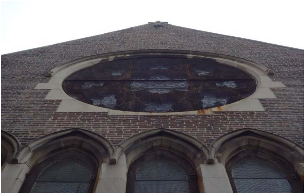
CHURCH SOUTH FACADE - TRANSEPT ROSE MASONRY OPENING AND WOOD TRACERY, TYPE 7 EXTERIOR VIEW
