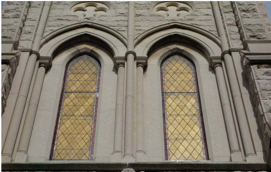
CHURCH STREET FACADE - TOWER STAINED GLASS MASONRY OPENINGS, TYPE 3 EXTERIOR VIEW
