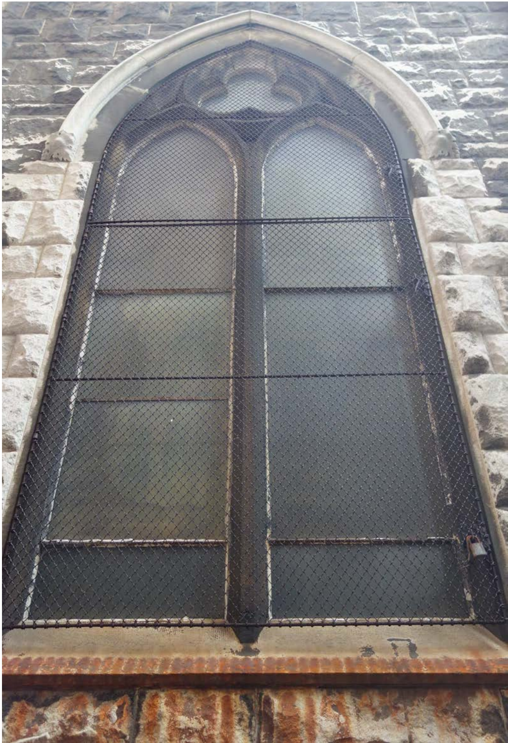
CHURCH NORTH FACADE - PORCH STAINED GLASS MASONRY OPENING AND TRACERY, TYPE 10 EXTERIOR VIEW
