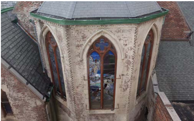
CHURCH REAR FACADE - APSE STAINED GLASS MASONRY OPENINGS AND WOOD TRACERY, EXT.
