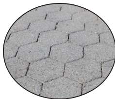
Hexagonal Asphalt Pavers
