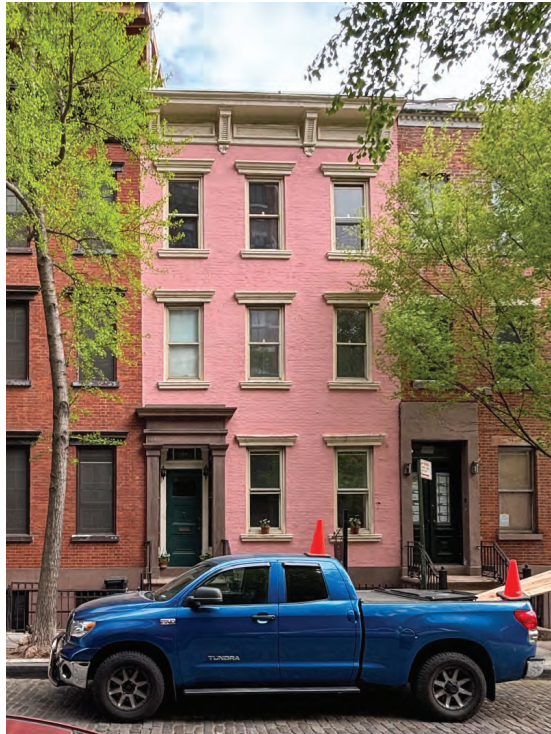
1 - View from Bank St (2025/04/25)
