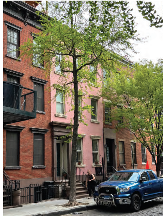
2 - View from Bank St (2025/04/25)
