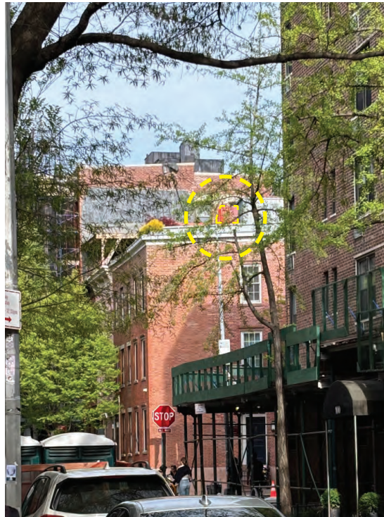
8 - View from Bank St (2025/04/25)
