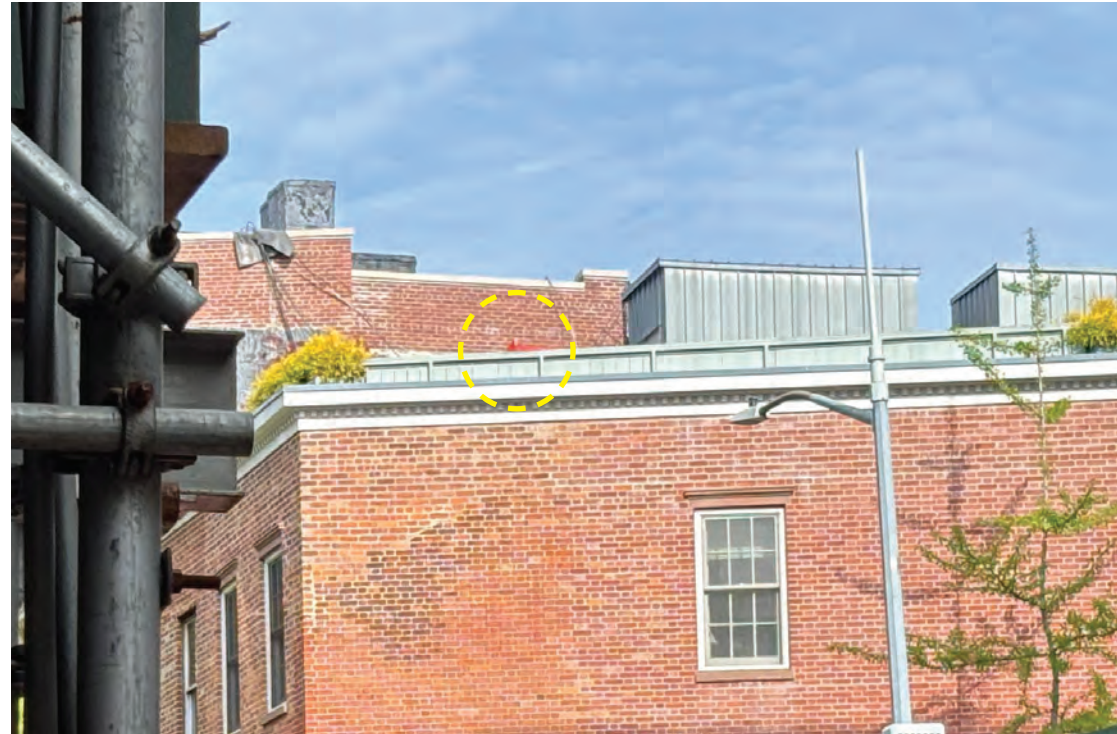
7 - View from Bank St (2025/04/25)
