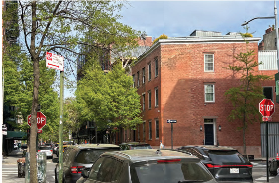
6 - View from Bank St (2025/04/25)
