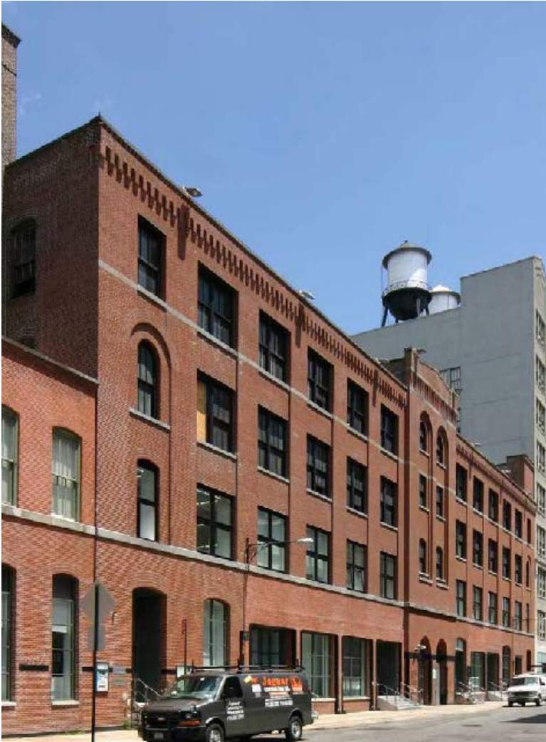
View of 521-537 W. 25 th Street. LPC West Chelsea Historic District Designation Report. 2008
