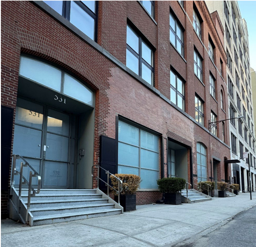
525 West 25 th Street, New York, NY Existing Conditions: detail of non-historic metal and glass infill at segmental arched and flat headed lintel conditions, non-historic stairs and handrails
