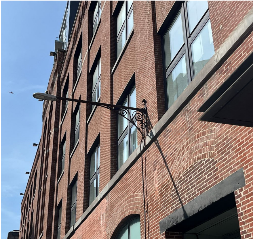
521-537 West 25 th Street, New York, NY Existing Conditions: detail of wall-mounted ornamental bracket with exposed conduit and non-historic luminaire to be restored (LPC Staff level review)
