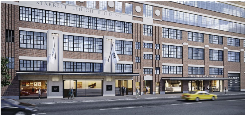
Starrett Lehigh Building, 601 West 26 th Street, New York, NY
