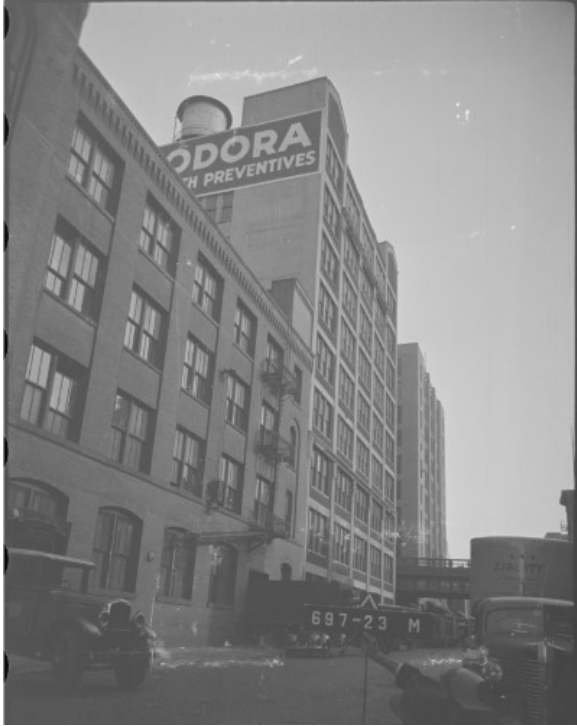
From West to East: 521-537 West 25 th Street (4 story building) 511-519 West 25 th Street (11 story bldg.)
