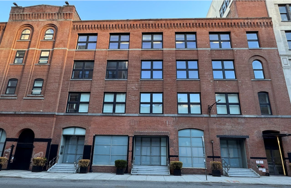
521-537 West 25 th Street, New York, NY Existing Conditions (detail view; East bays and central tower)
