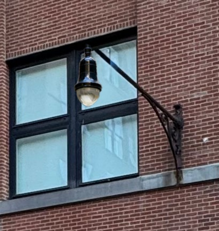
Rendered view of proposed condition: restored metal bracket with black painted finish, new tear drop luminaire, concealed conduit.
