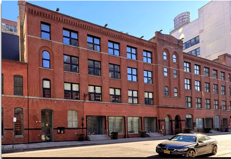
Existing Conditions of 521-537 West 25 th Street (West)
