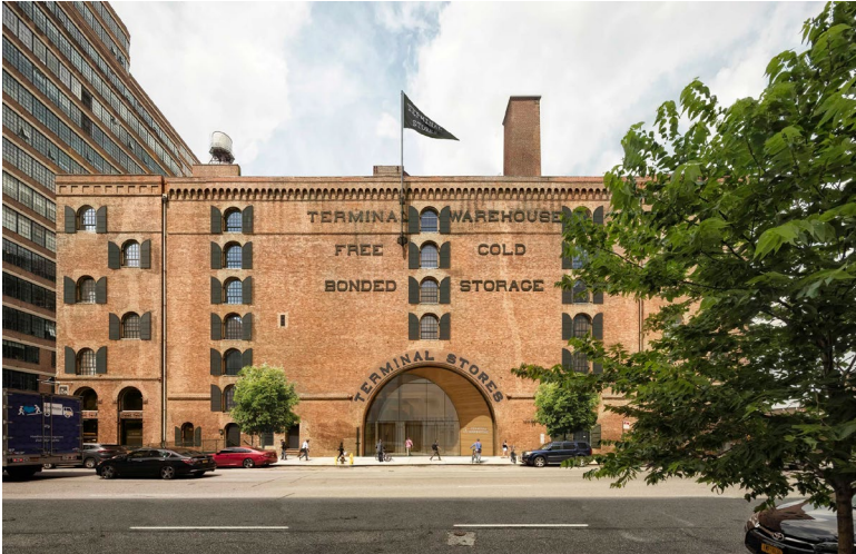
Terminal Warehouse, 261 11 th Avenue, New York, NY
