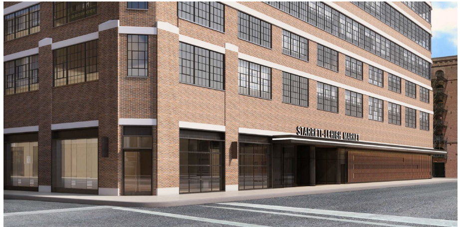
Starrett Lehigh Building, 601 West 26 th Street, New York, NY
