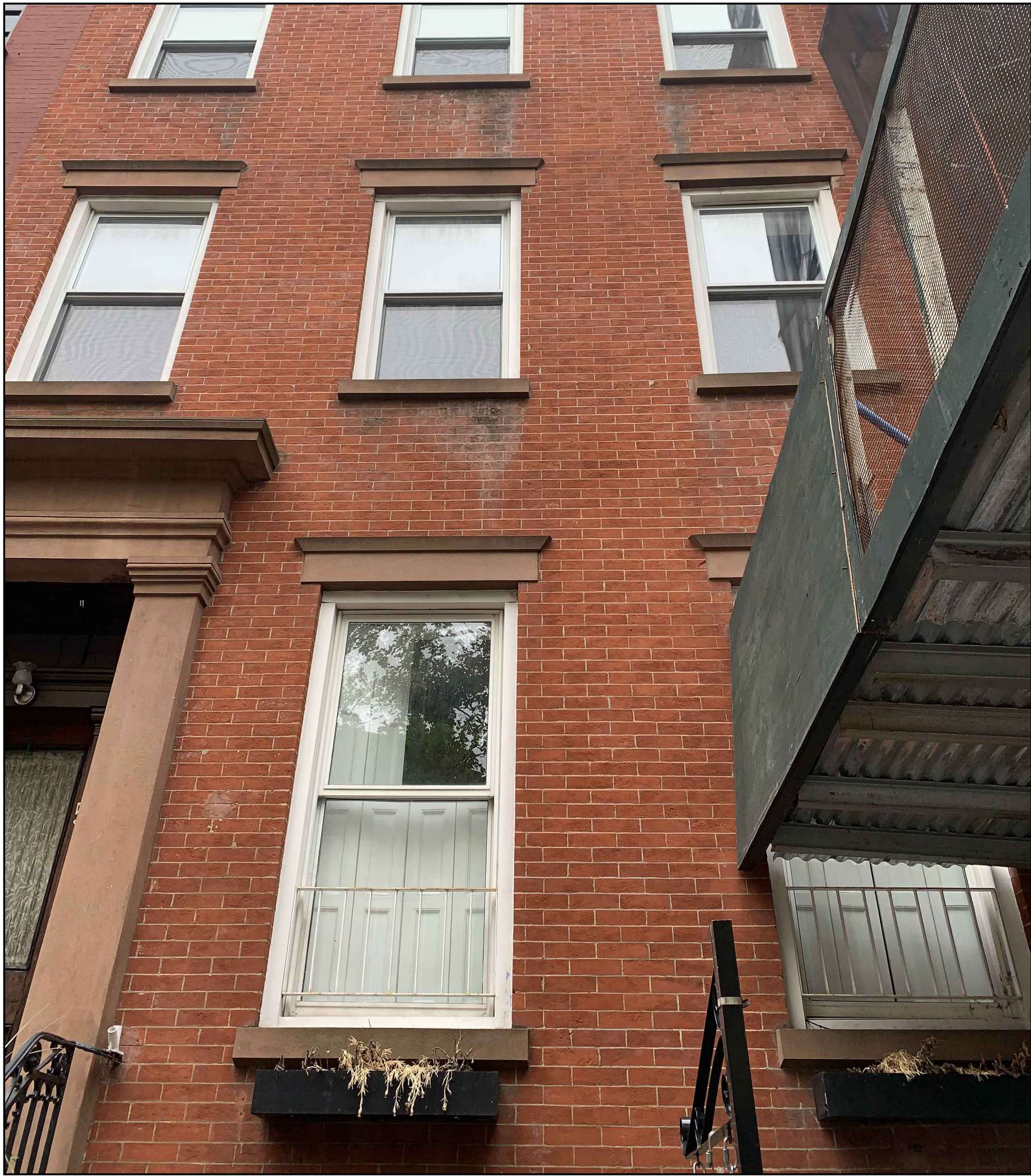
02 FRONT FACADE EXISTING WINDOWS & BRICKMOLDS FROM JORALEMON ST.
