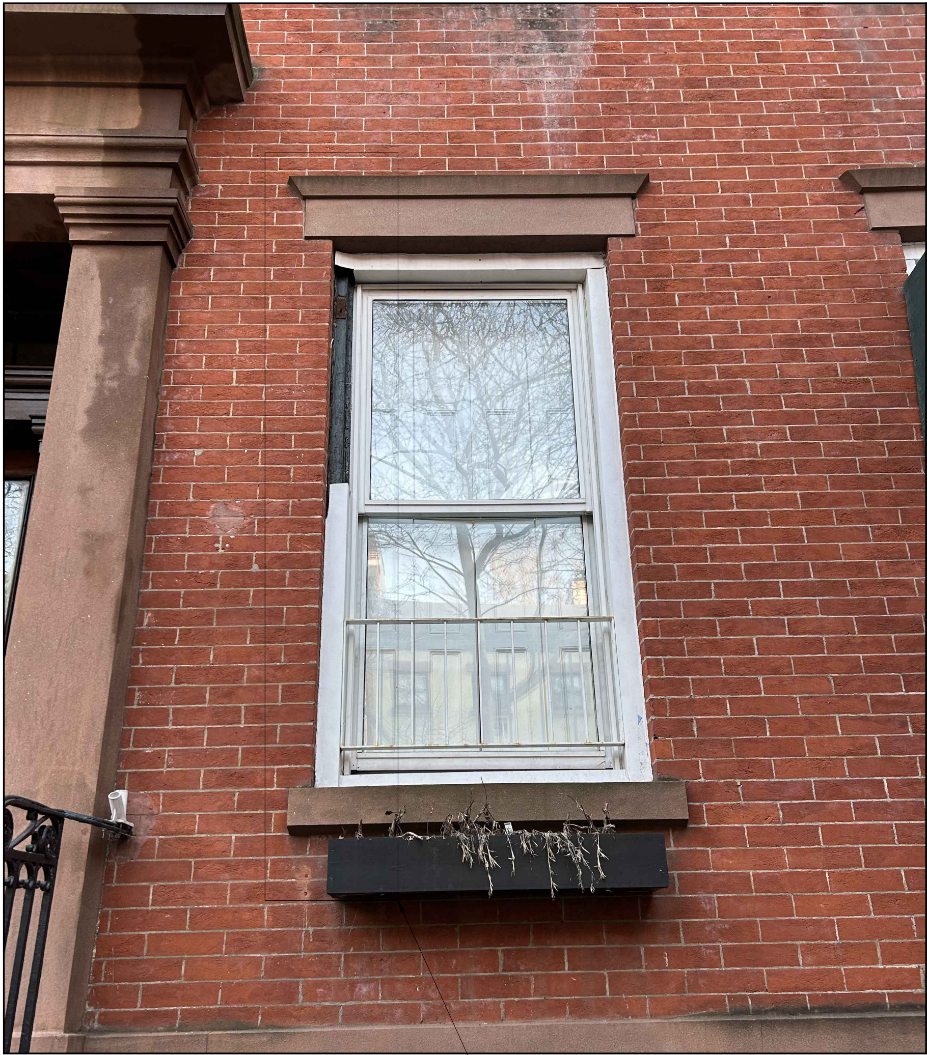
05 FRONT BRICKMOLDS FROM JORALEMON ST. W/ REMOVED PANNING
