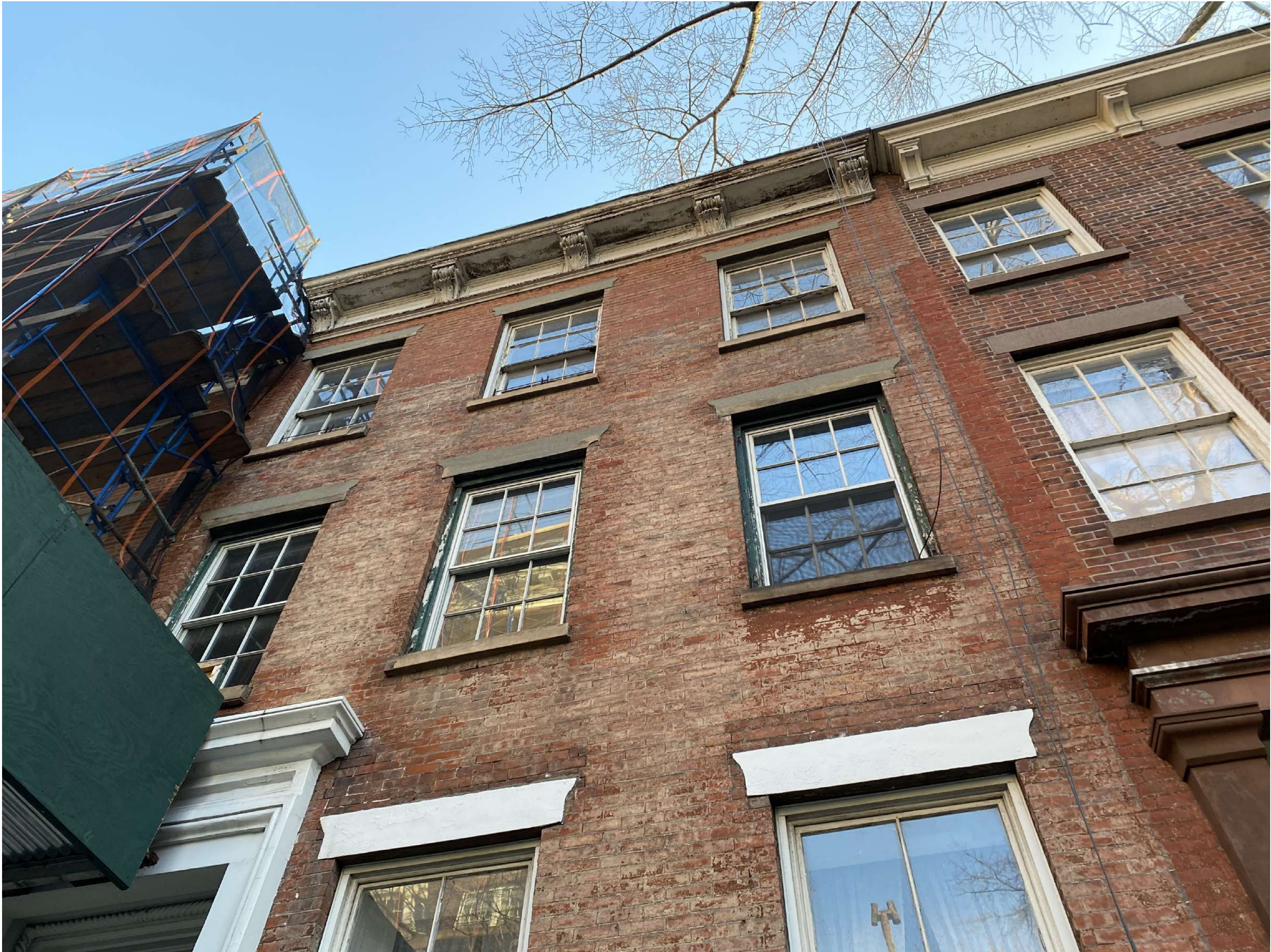
DETAIL OF EXISTING CORNICE & WINDOW HEADS/SILLS
