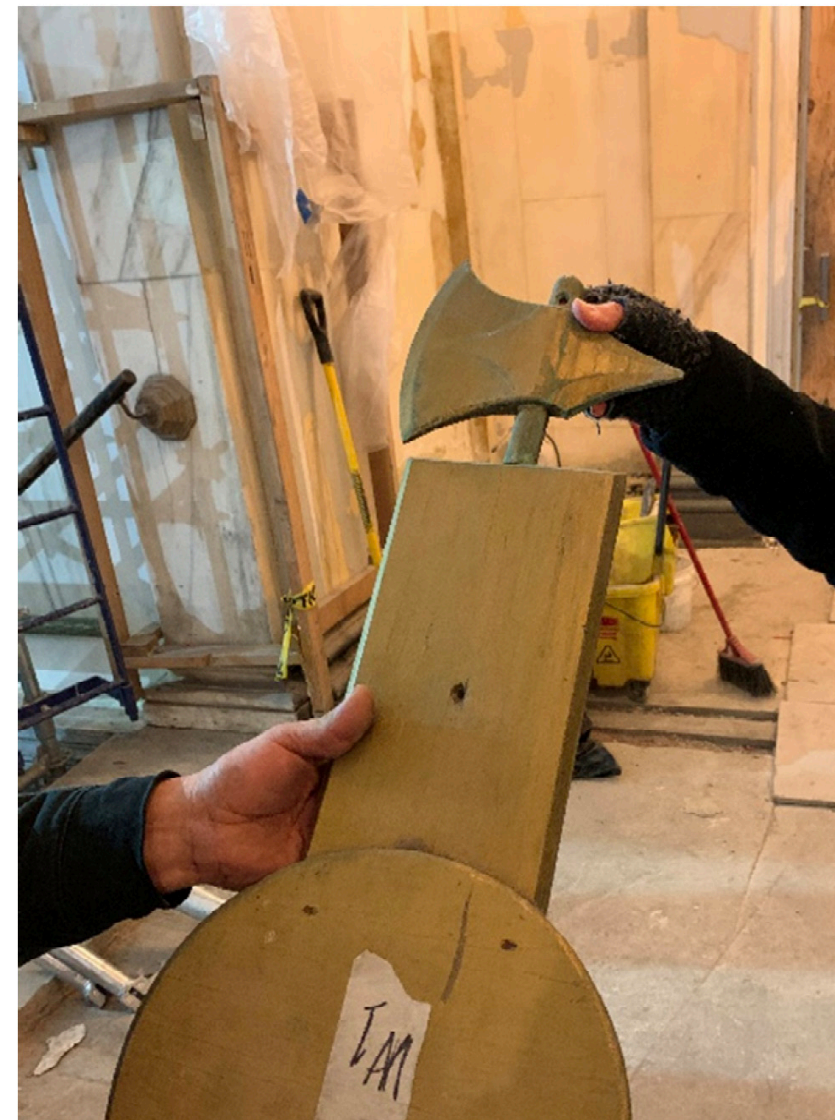
Roughly finished wood replacement of historic bronze fasces and monogram, existing with bronze axe head at all locations at the start of the project (April 2019 Beyer Blinder Belle Field Observation Report)
