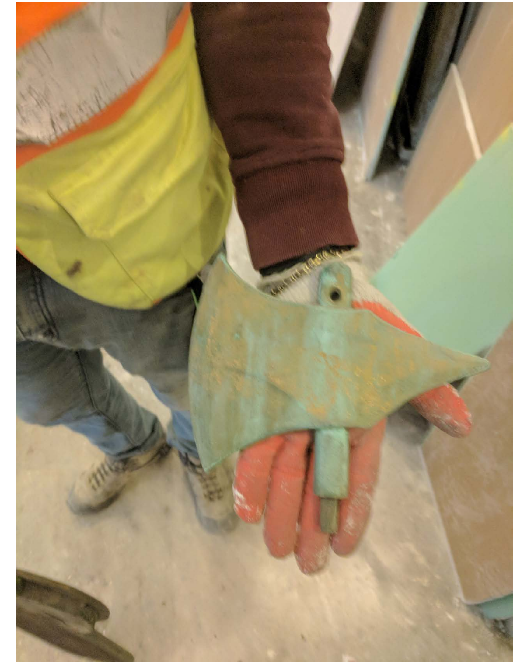
Roughly finished wood replacement of historic bronze fasces and monogram, existing with bronze axe head at all locations at the start of the project (April 2019 Beyer Blinder Belle Field Observation Report)
