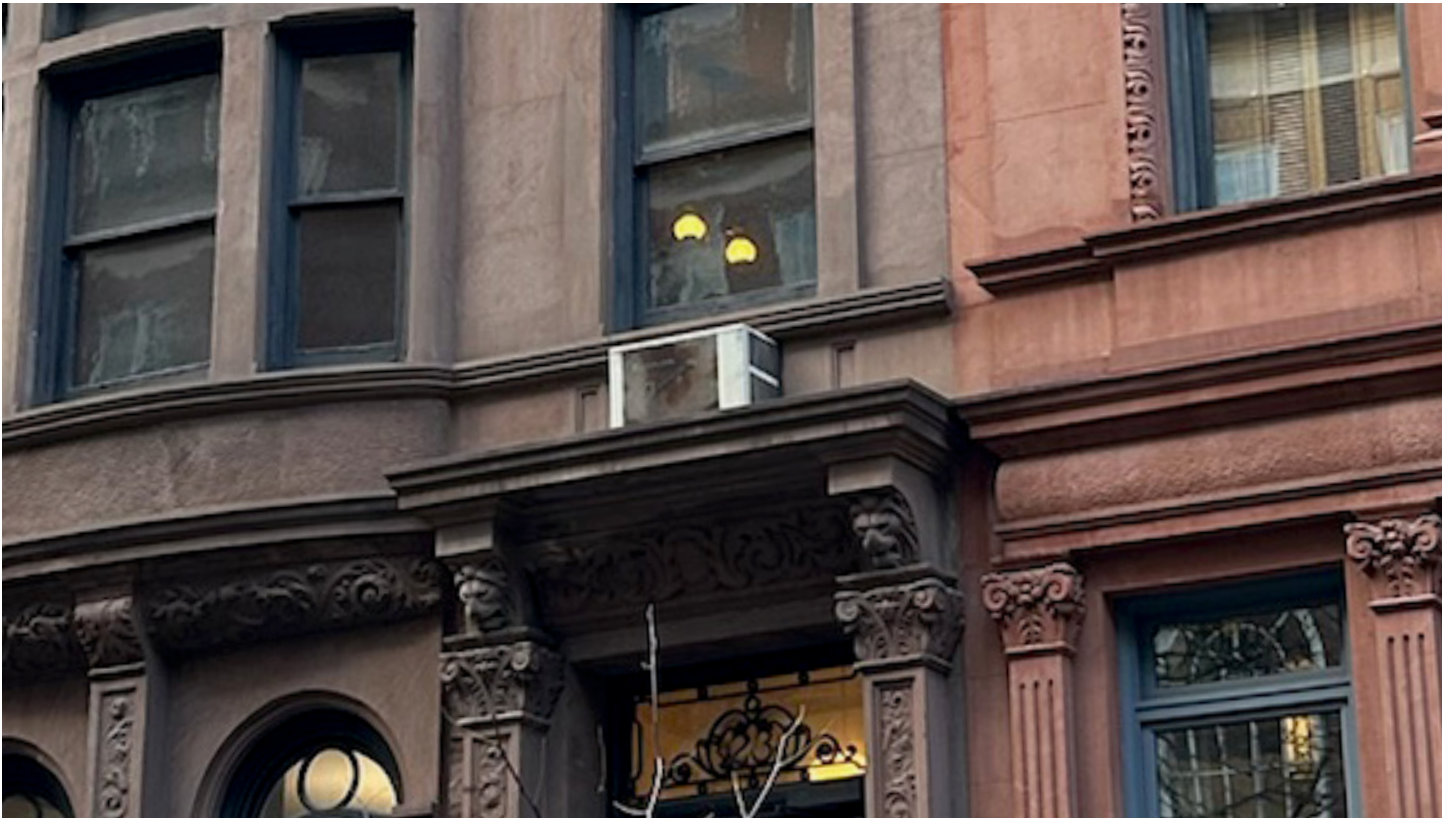
Through-wall air conditioner unit at second-floor spandrel, facing northwest.
