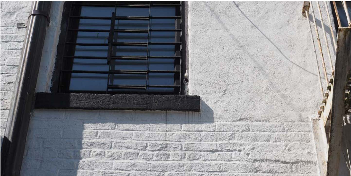
Existing fifth-story window sill and parged brickwork.
