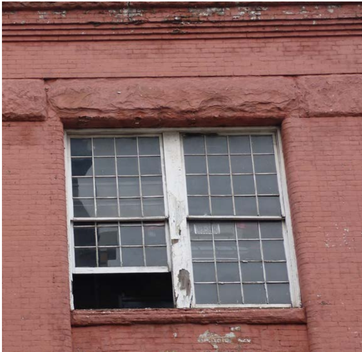
Wood paired double-hung windows with brownstone lintel.
