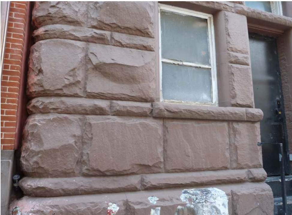
Rusticated, painted brownstone at the garage's water table.
