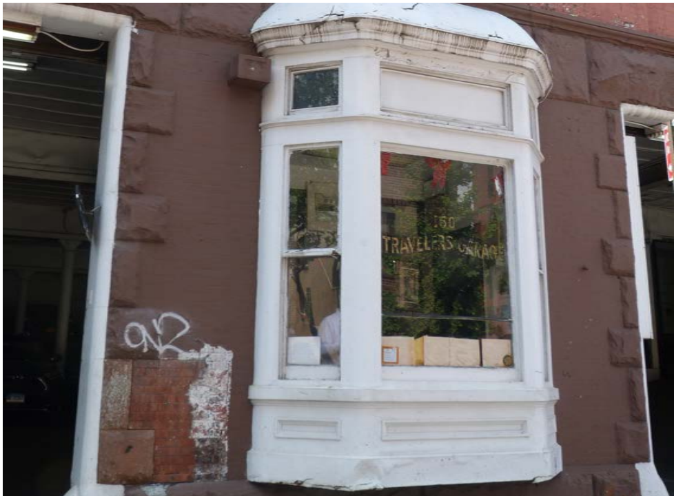
Wood paired double-hung windows with brownstone lintel.
