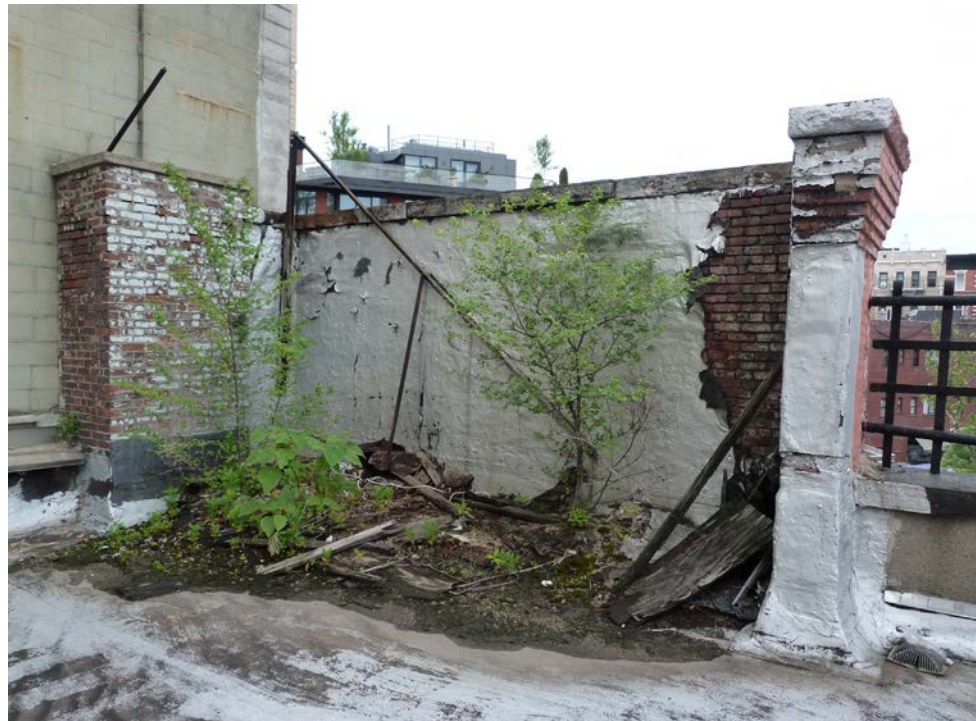
Vegetation growing behind the western projecting parapet.
