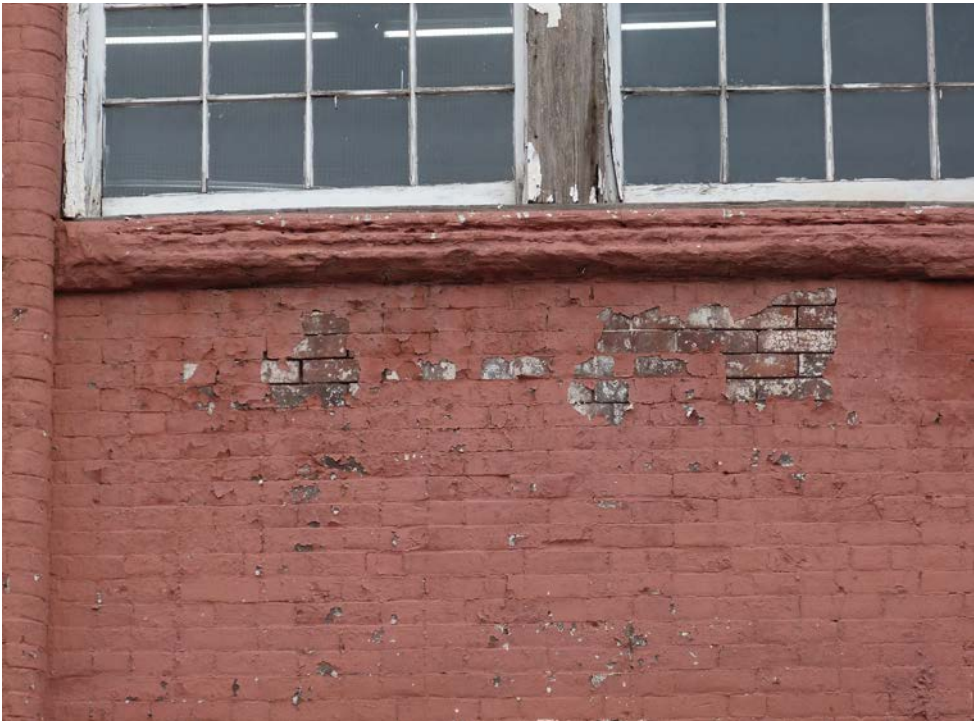
Painted brick, open joints, and sill erosion at the second story.
