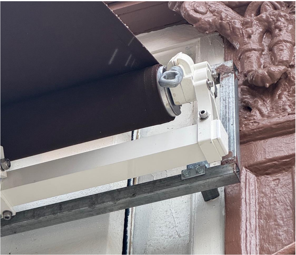
Right Anchoring on wood paneling
