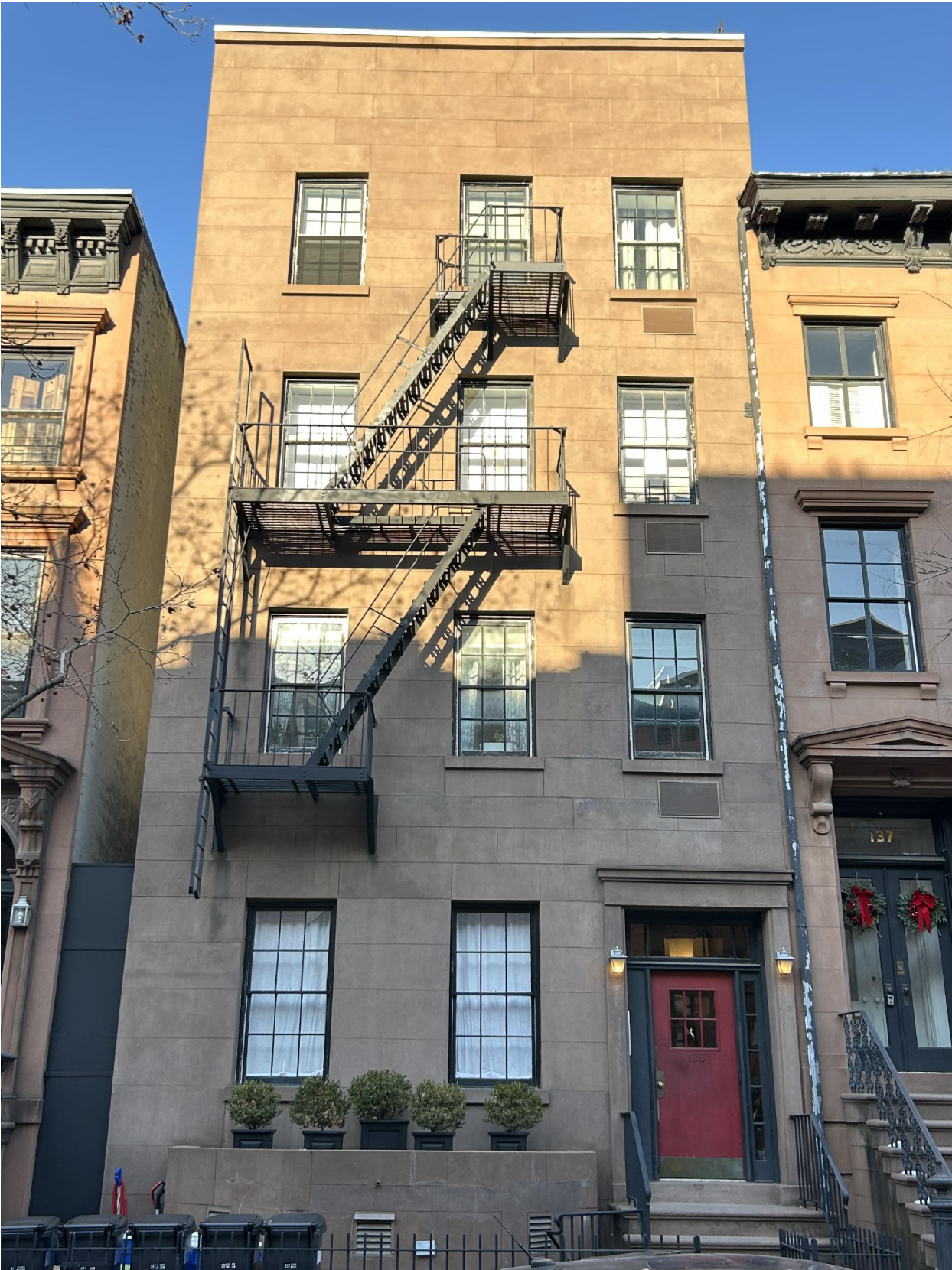
1 EXISTING FRONT FACADE
