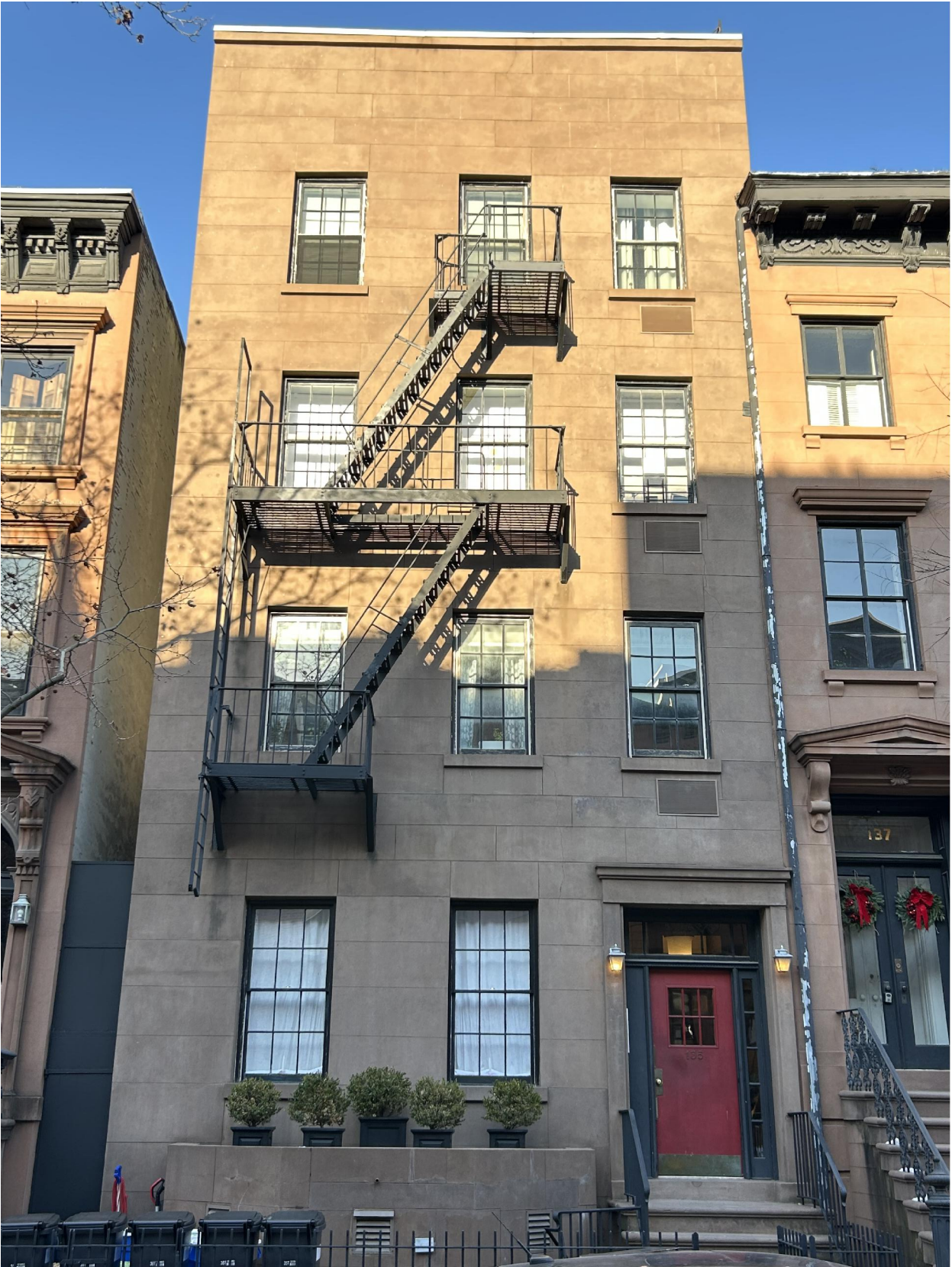
1 EXISTING FRONT FACADE
