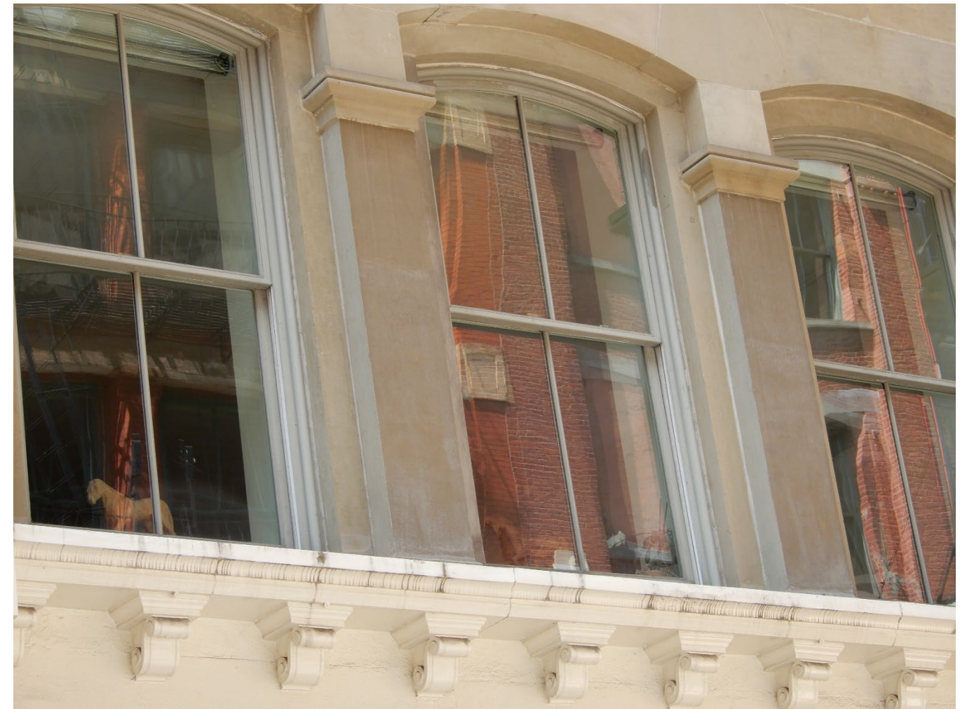
115 MERCER 2 ND FLOOR SHOWING COATED LIMESTONE AND HARDWARE FOR PREVIOUS FLAG
