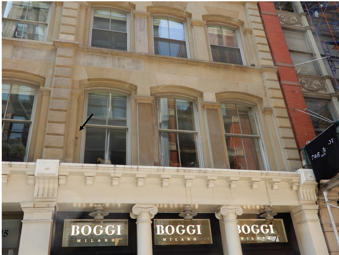
115 MERCER 2 ND FLOOR SHOWING COATED LIMESTONE AND HARDWARE FOR PREVIOUS FLAG
