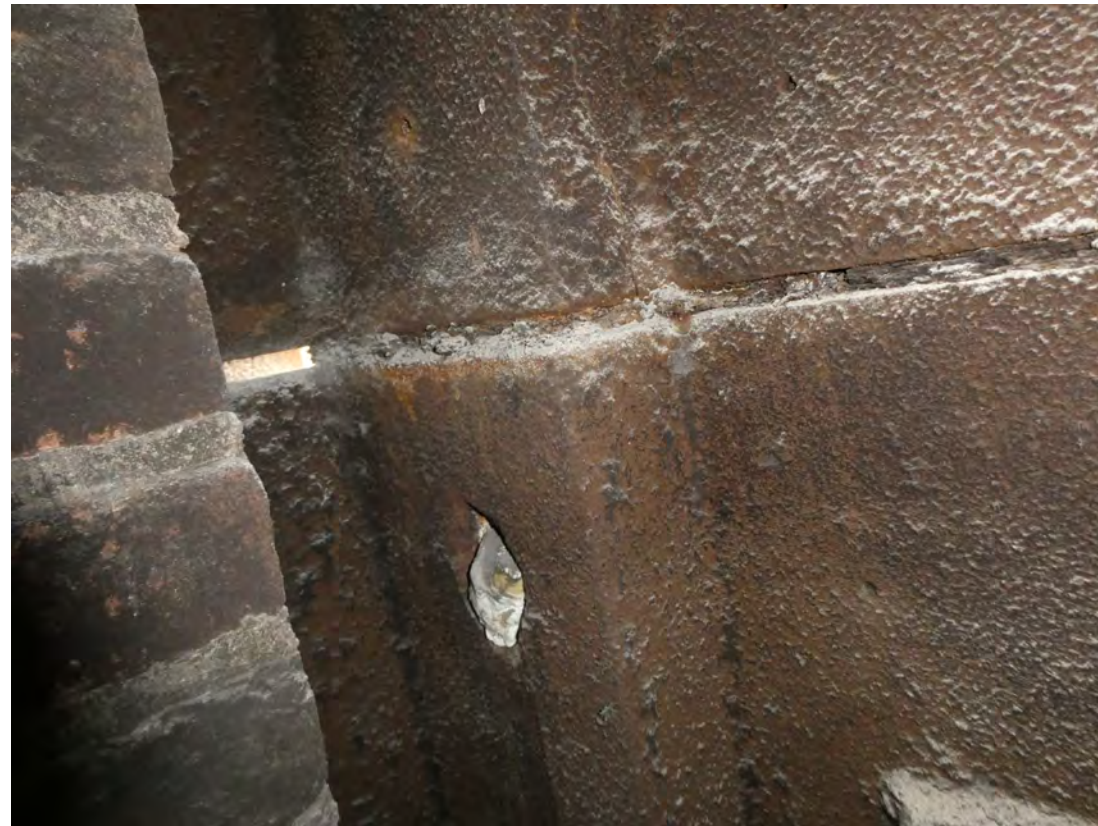
CAST-IRON CRACKING, RUST JACKING AND DISPLACEMENT
