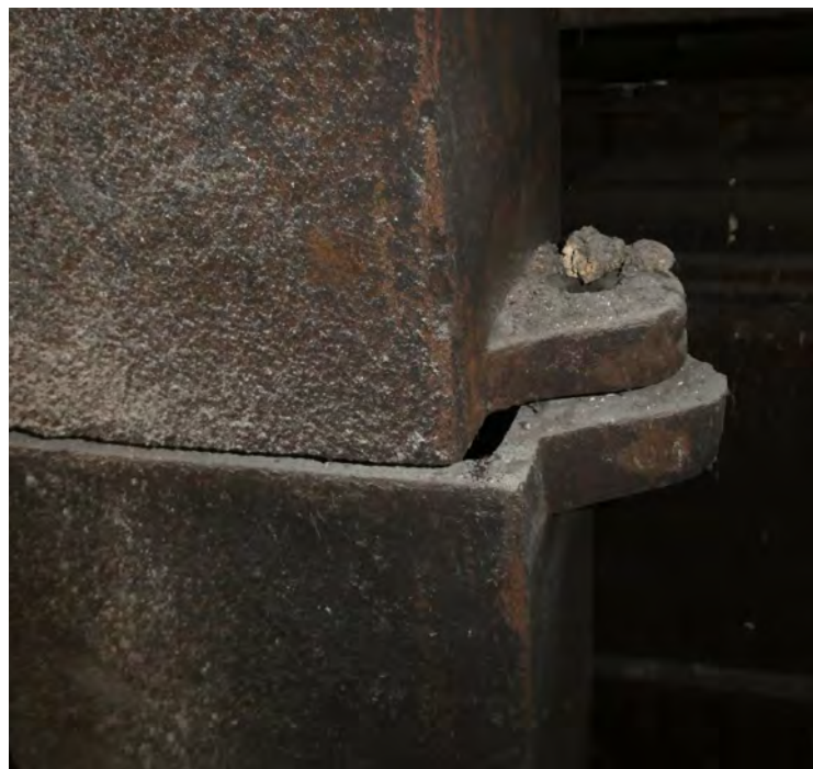
CAST-IRON CRACKING AND DISPLACEMENT
