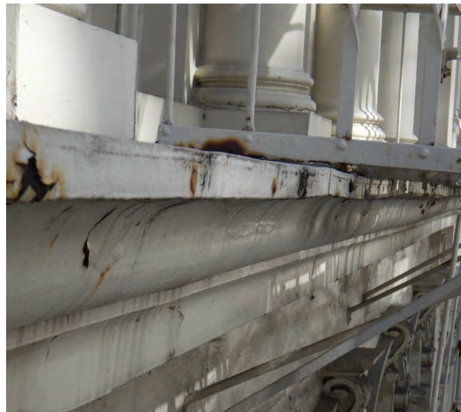
FIRE ESCAPE PENETRATIONS AND WARPING AT WATER TABLES
