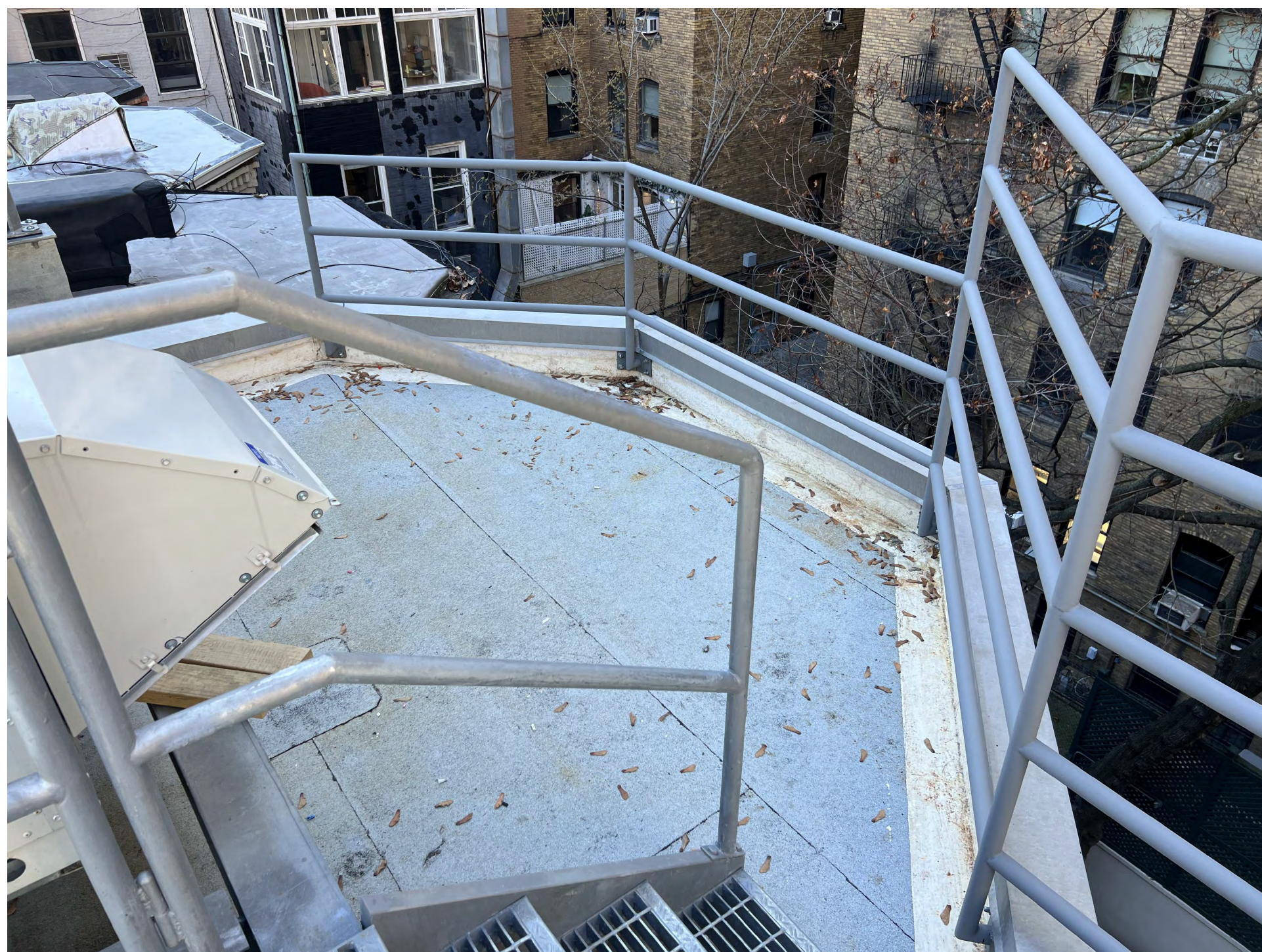
AS BUILT PARAPET AND FDNY RAILINGS
