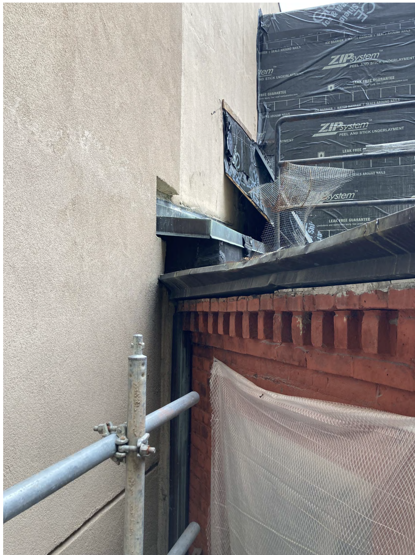
PHOTOS OF EXISTING DAMAGED BRICK CORBEL AND GUTTER POST REMOVAL
