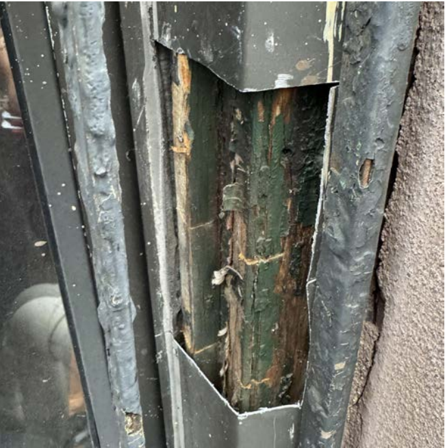
2 EXISTING BRICKMOLD
