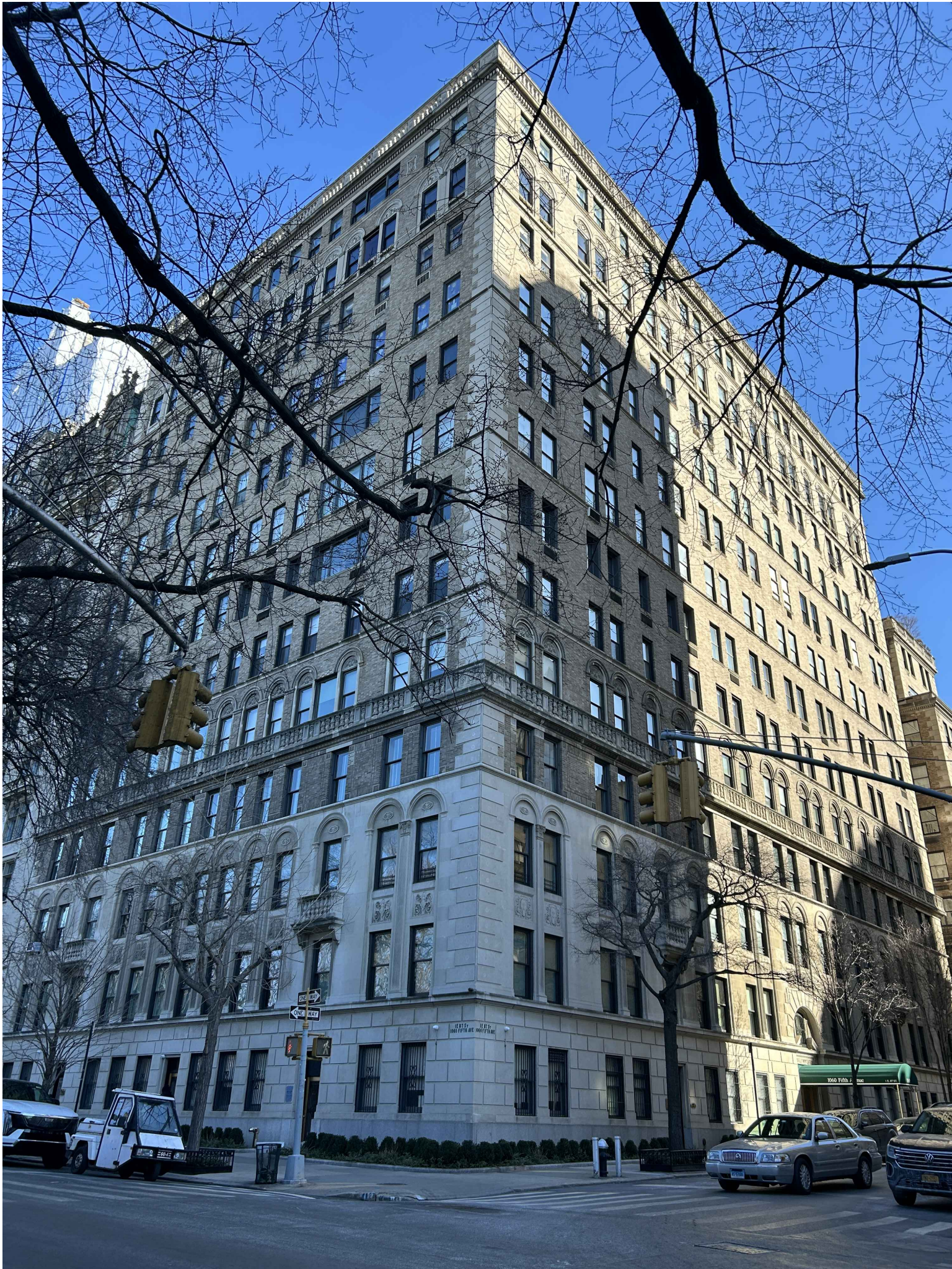
STREET VIEW - NORTHEAST CORNER OF FIFTH AVE. AND 87TH ST.
