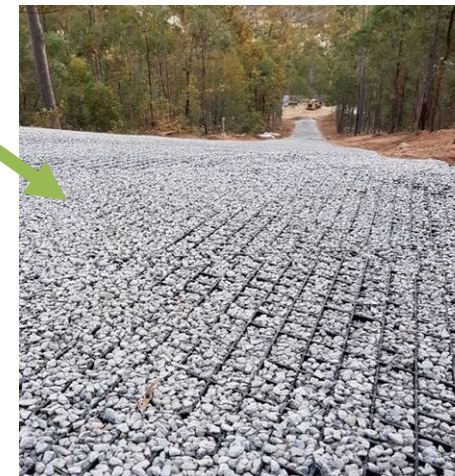
Proposed Diamond Grid filled w/ gravel - Path Profile - 5.5" depth
