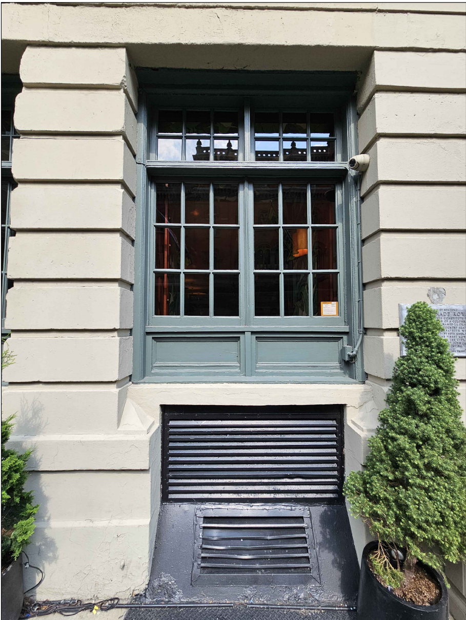
EXISTING WINDOW WITH VENT GRILL
