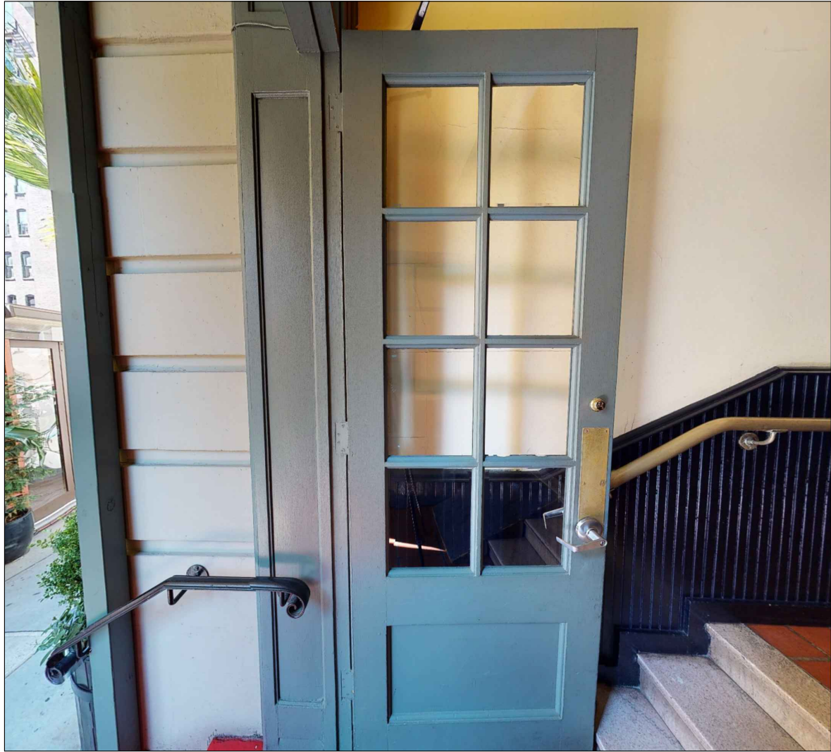
EXISTING ENTRANCE DOOR & RAILINGS (LEFT)
