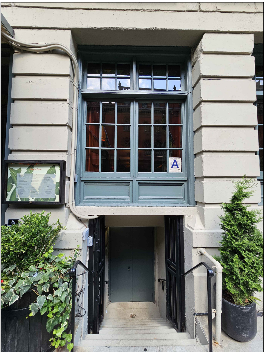
EXISTING WINDOW WITH ACCESS TO THE BASEMENT
