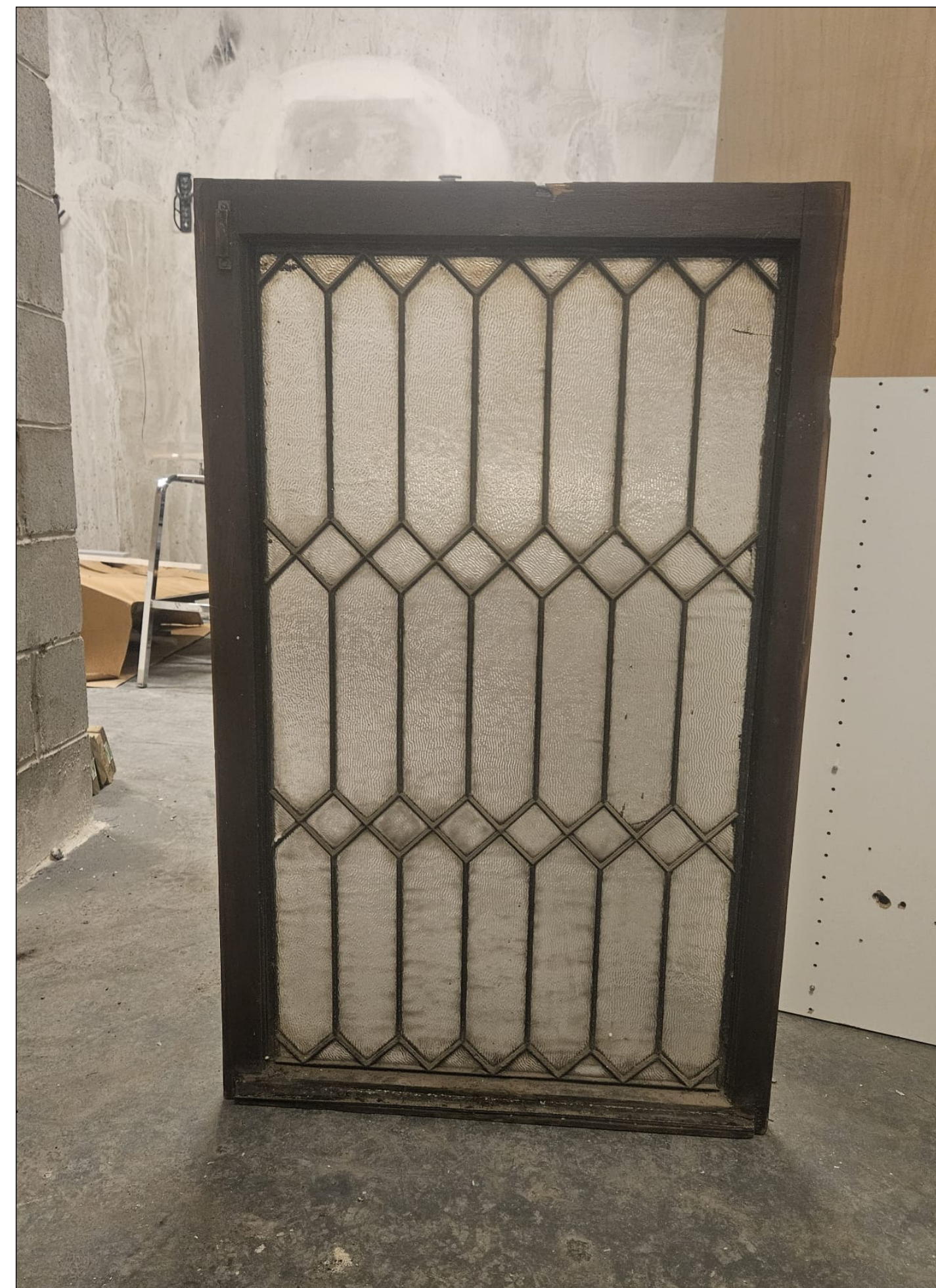
- REMOVED & STORED ORIGINAL WINDOWS
