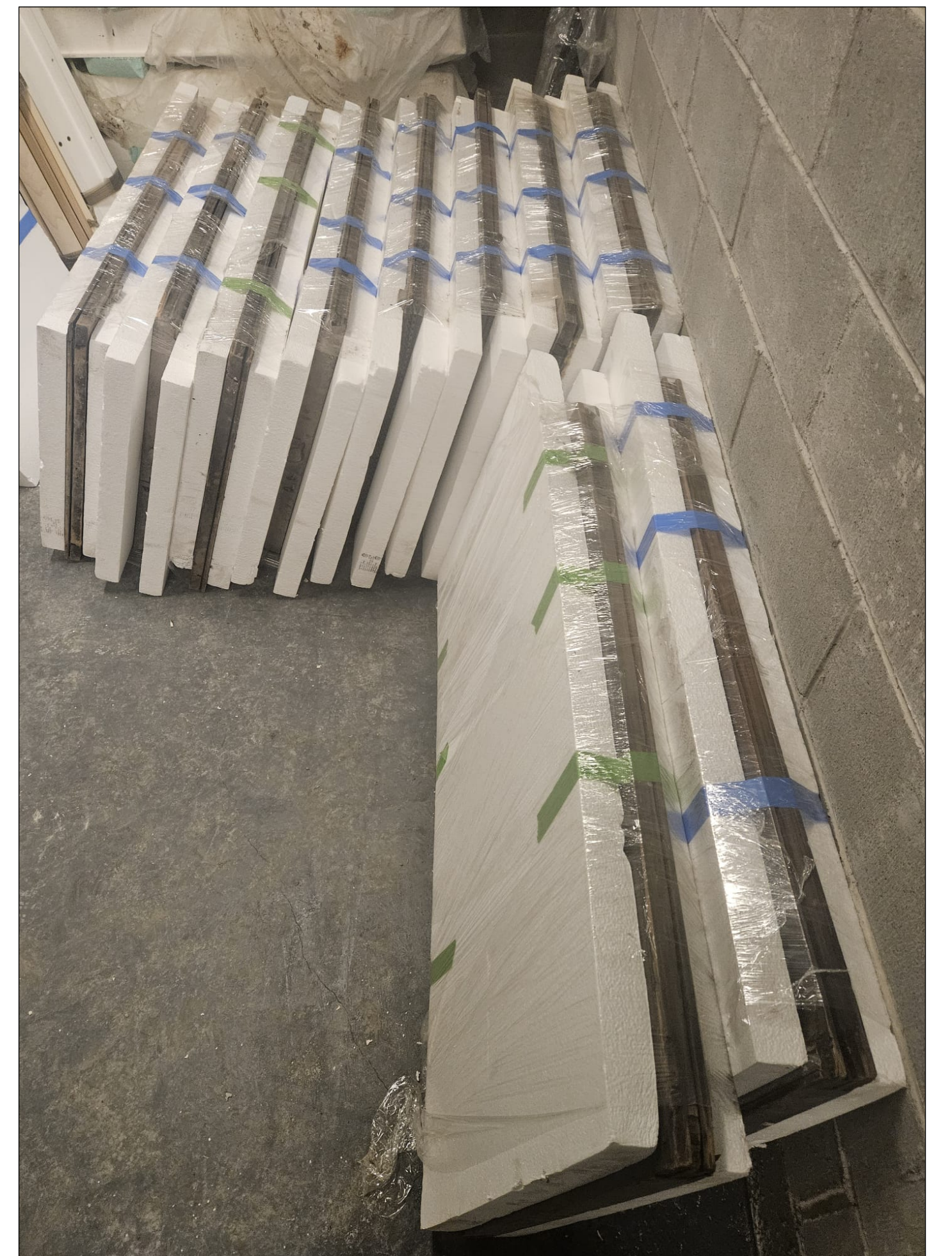
- REMOVED & STORED ORIGINAL WINDOWS
