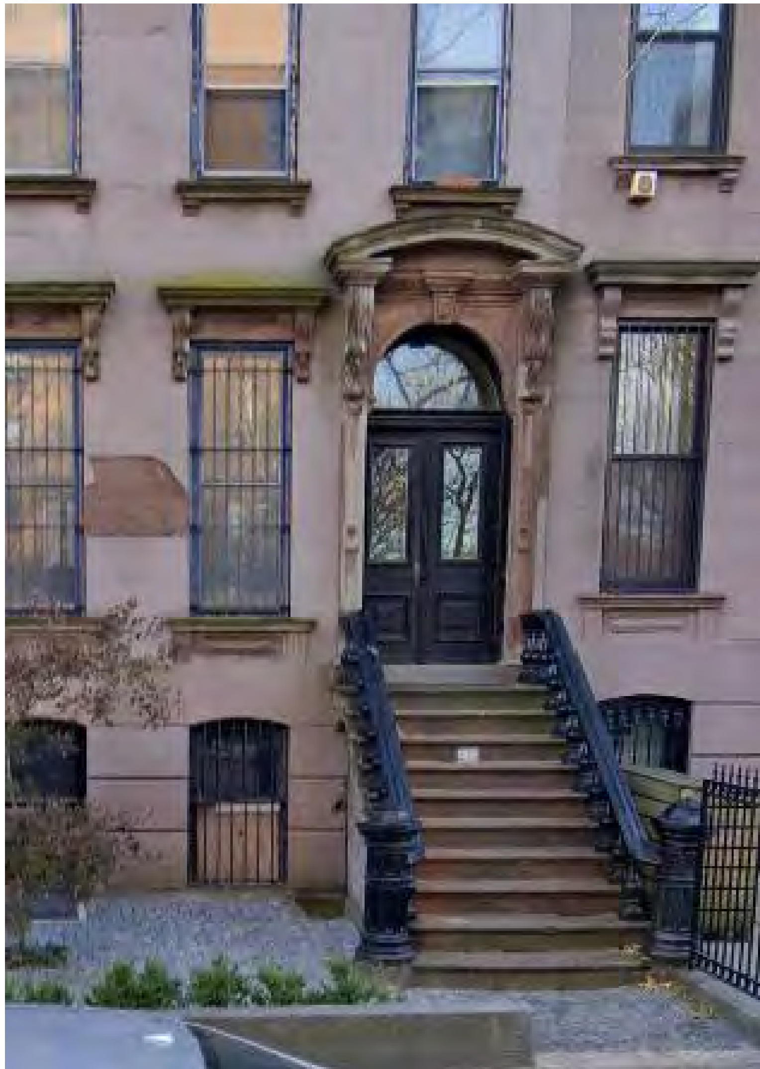
04 AREAWAY PAVING PHOTO 2017 STREET VIEW
