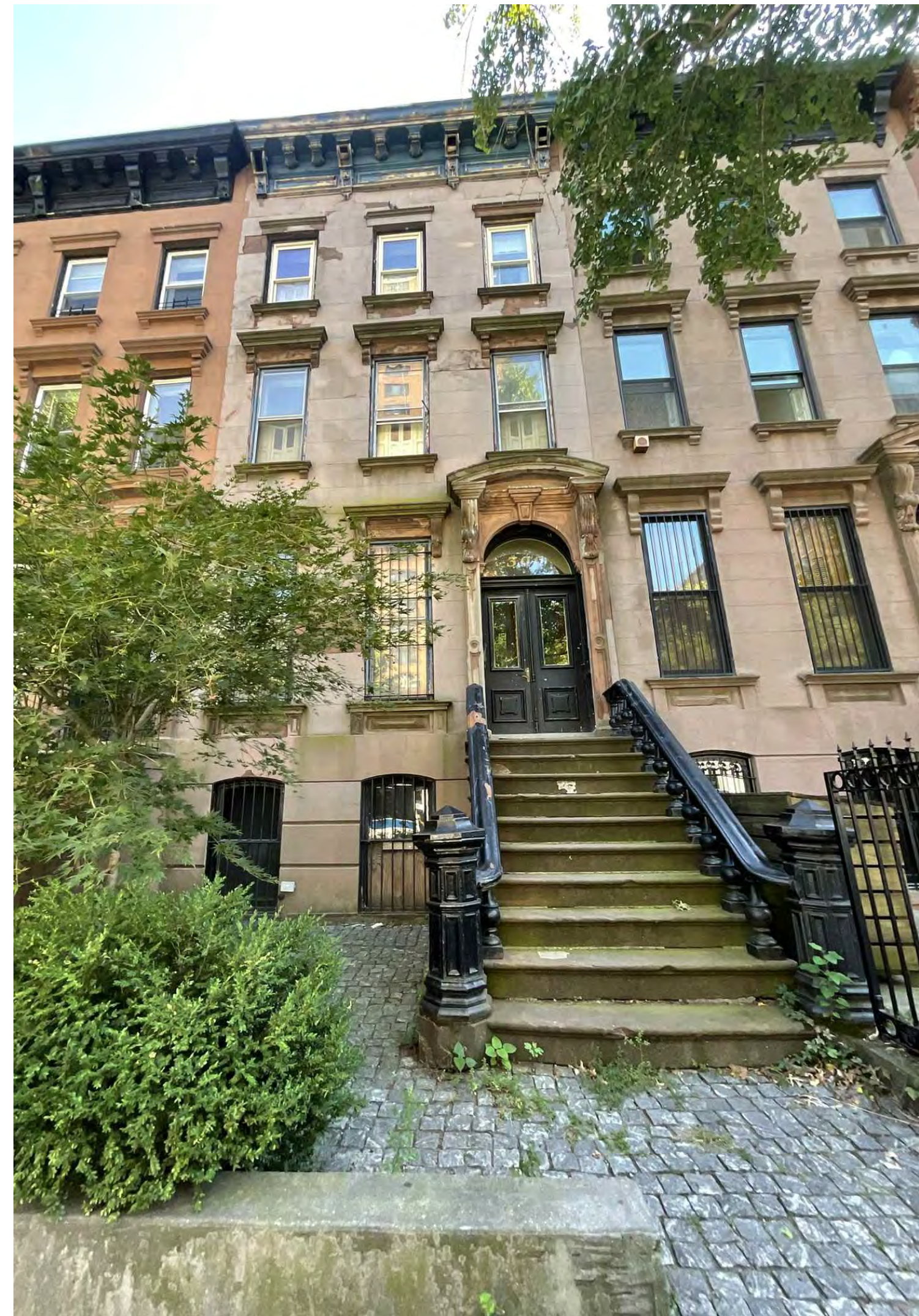
05 AREAWAY PAVING PHOTO 2025
