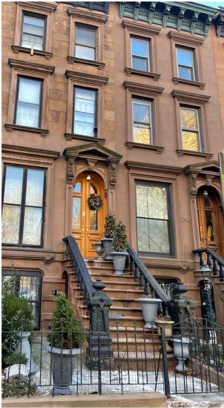
01 AREAWAY PAVING PHOTO 294 LAFAYETTE AVE.
