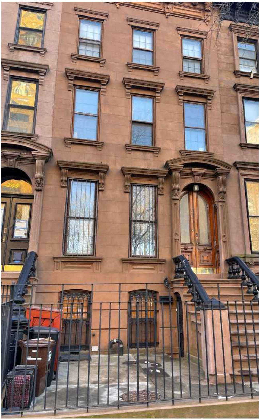
02 AREAWAY PAVING PHOTO 296 LAFAYETTE AVE.
