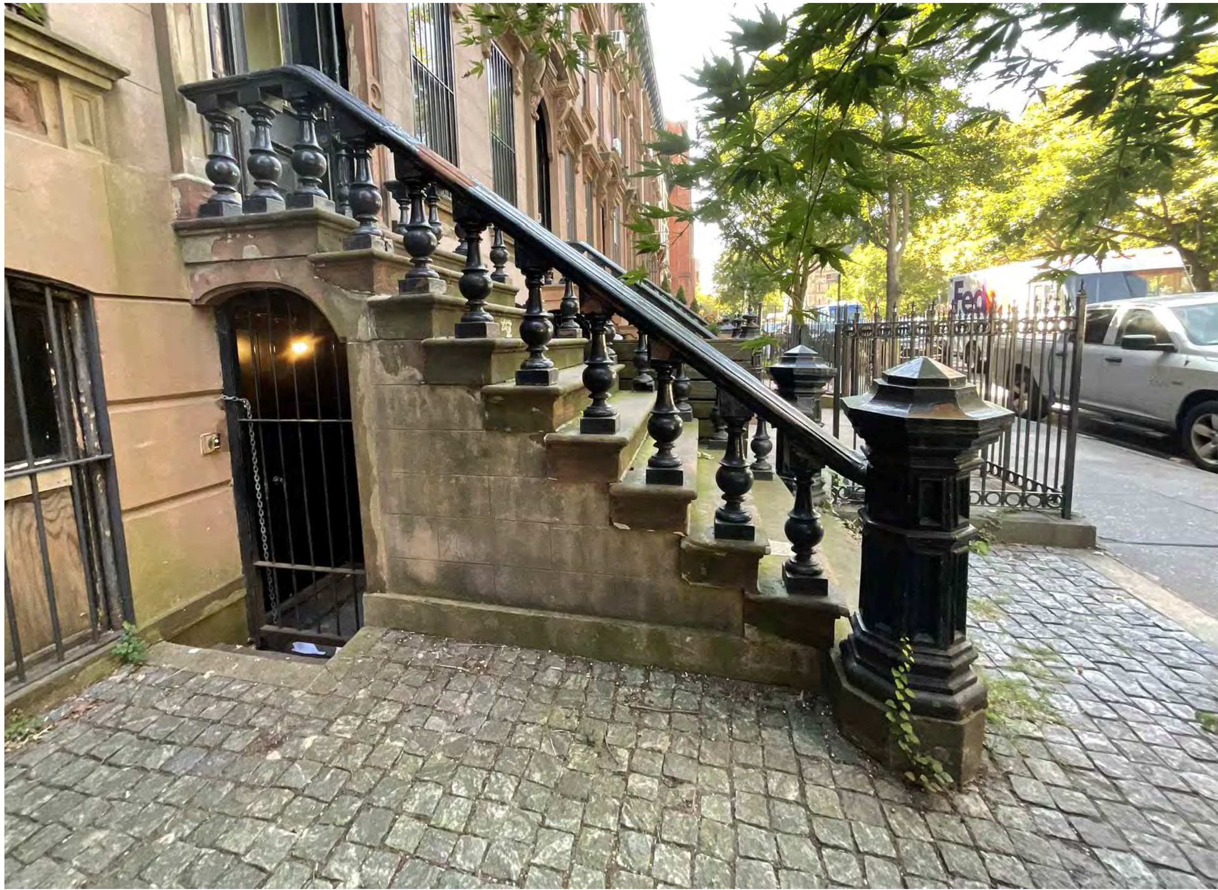
01 AREAWAY PAVING PHOTO 2025 1
