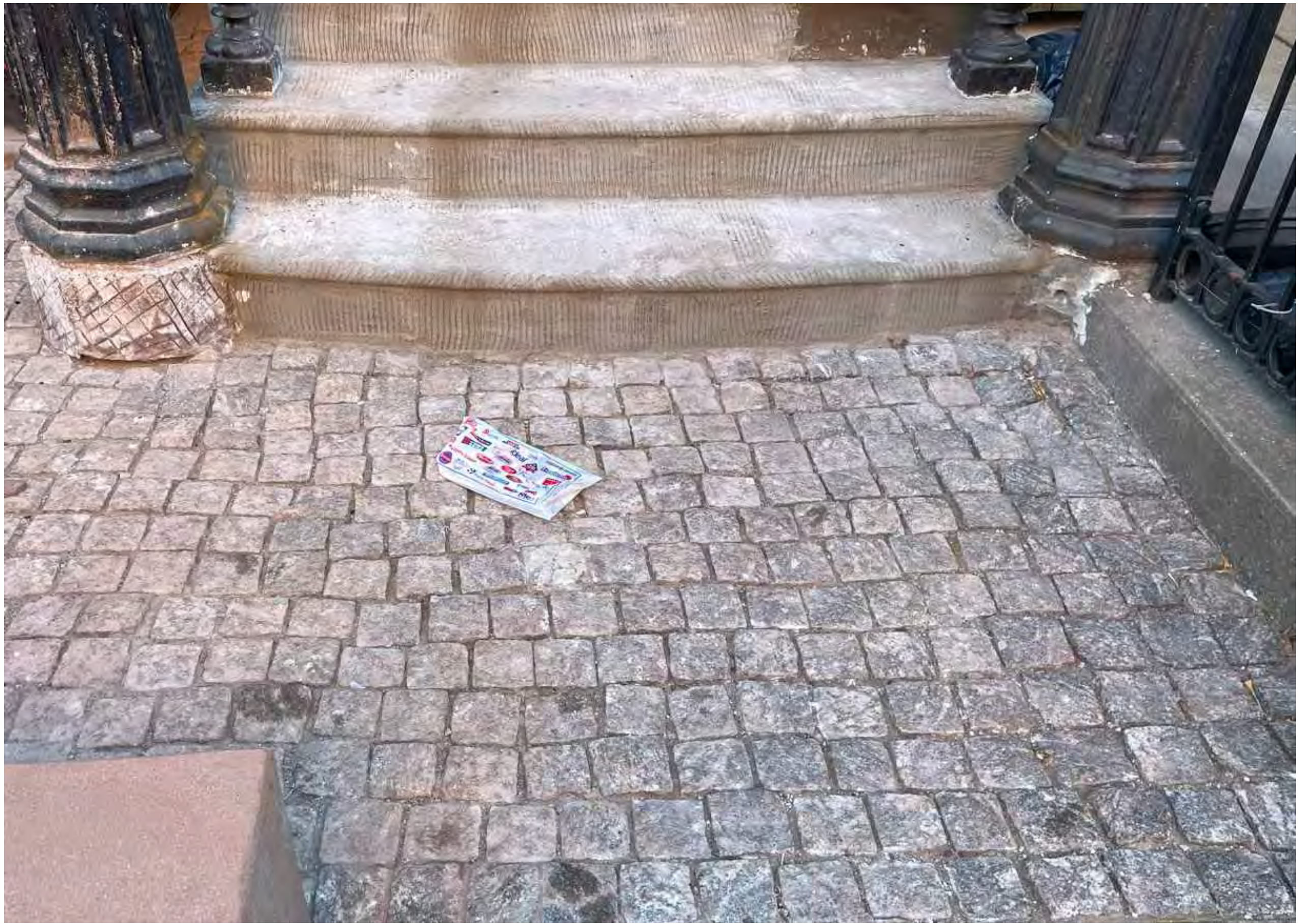
02 AREAWAY PAVING PHOTO 2025 2
