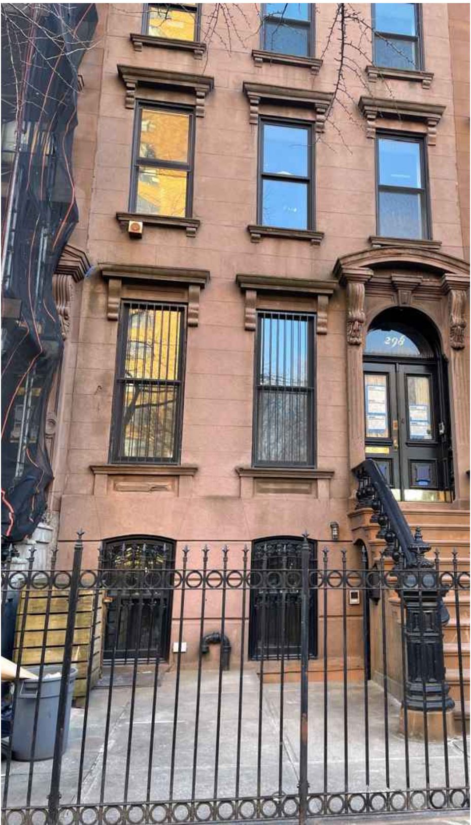
03 AREAWAY PAVING PHOTO 298 LAFAYETTE AVE.
