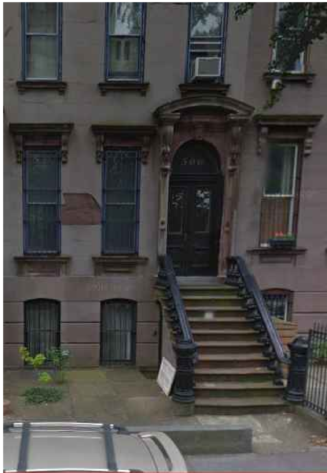
02 AREAWAY PAVING PHOTO 2012 STREET VIEW
