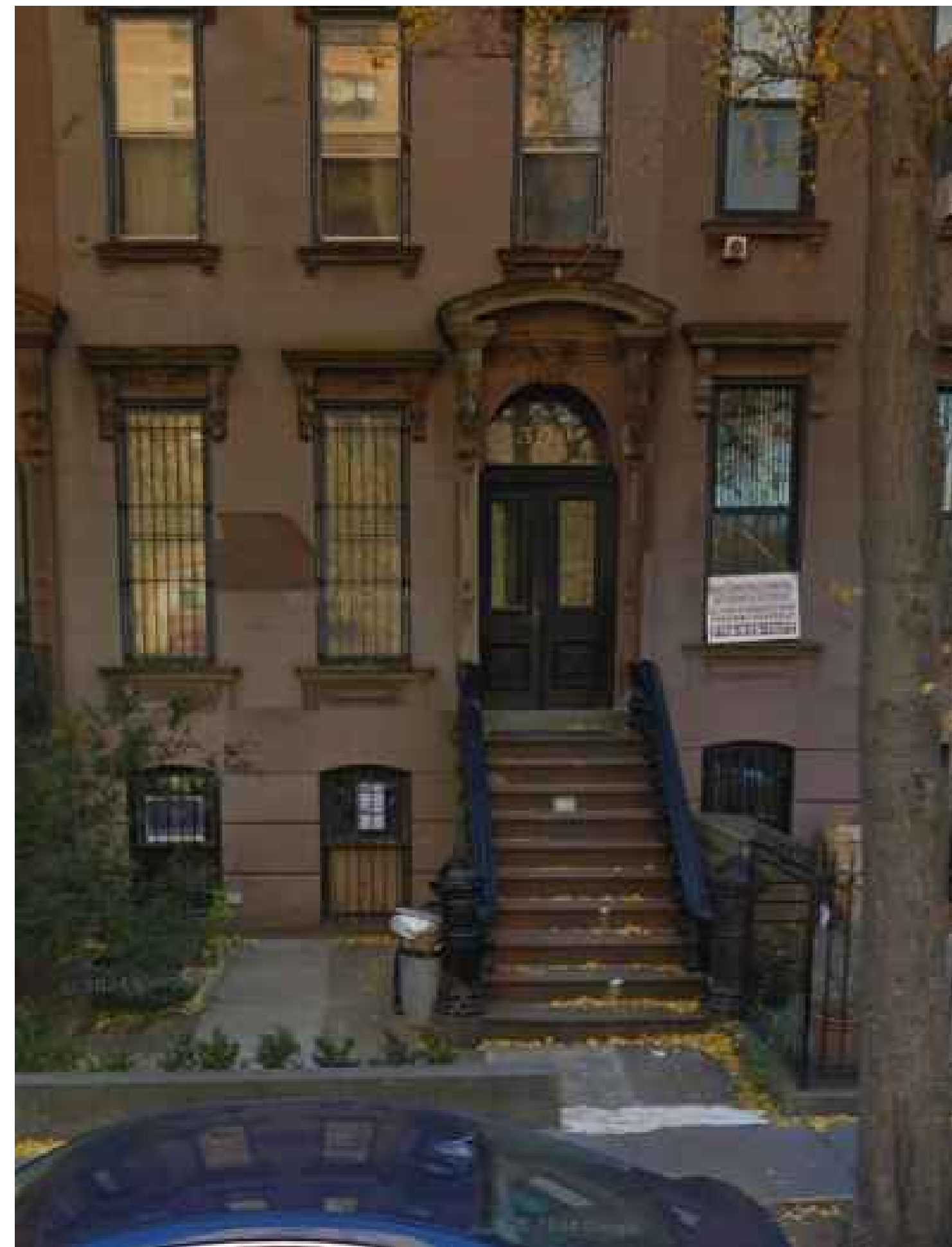
03 AREAWAY PAVING PHOTO 2016 STREET VIEW
