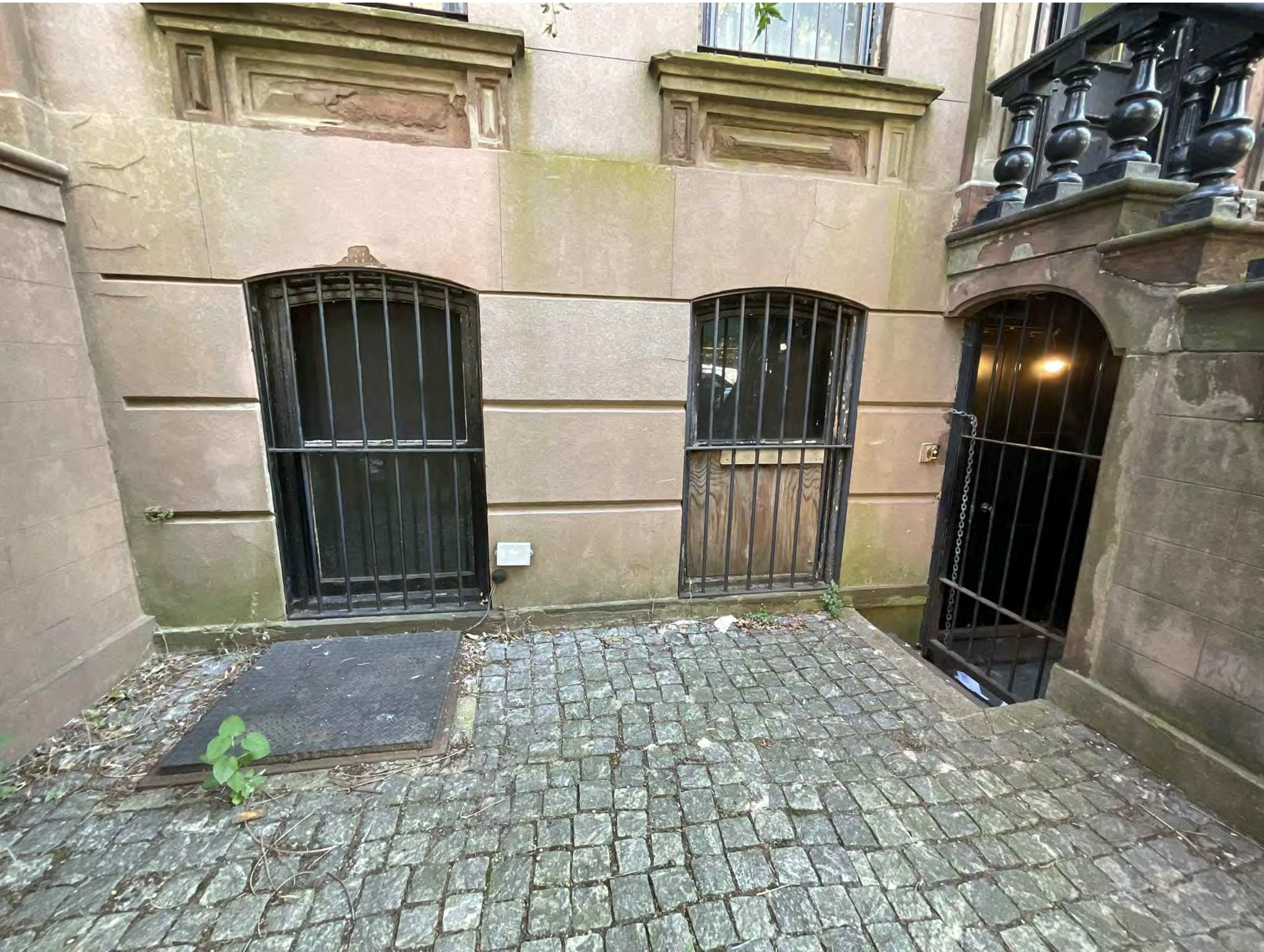
03 AREAWAY PAVING PHOTO 2025 3
