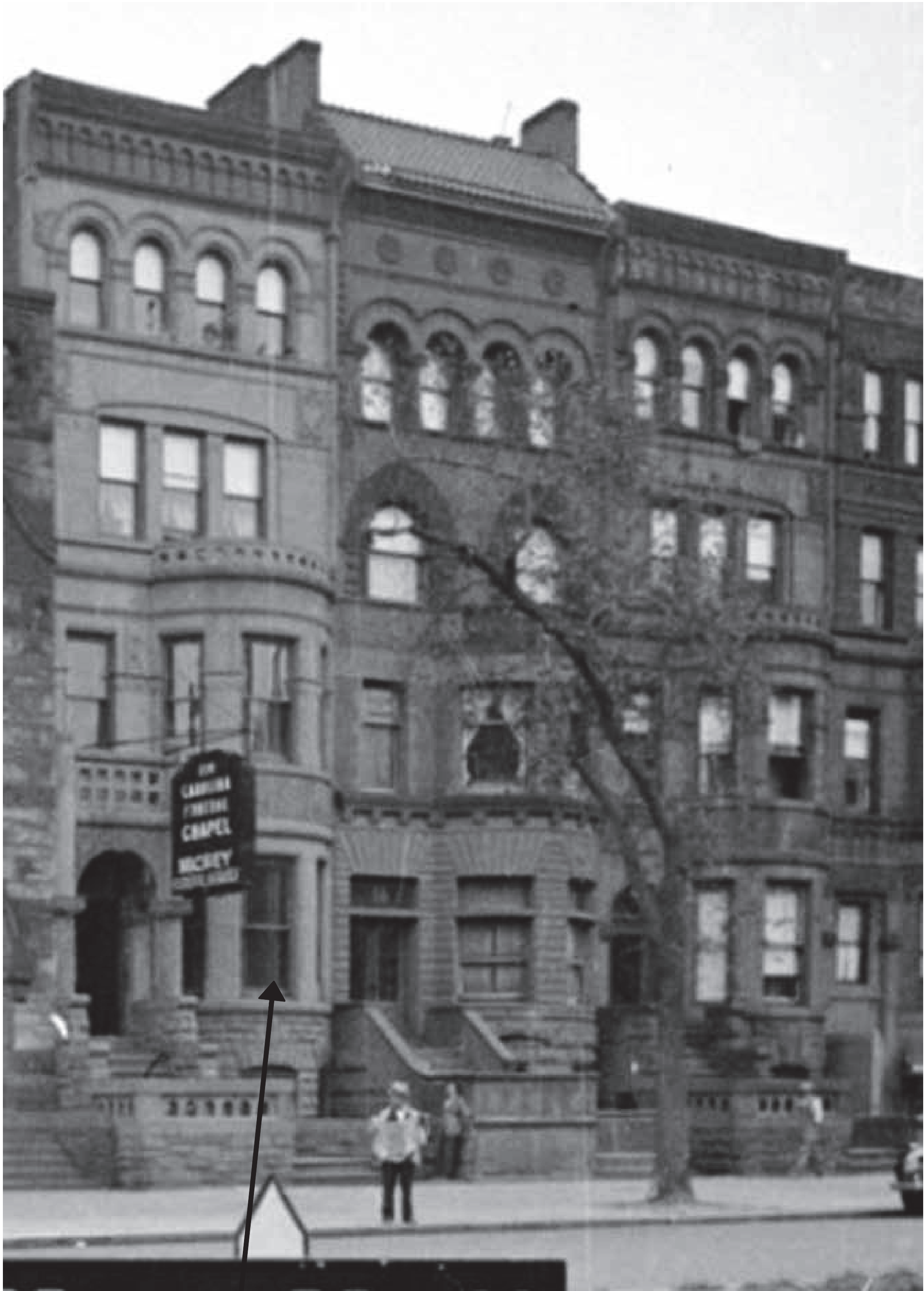
PHOTO OF (A TOTAL # OF 8) EXISTING BENT GLAZED WINDOWS AT BAY
