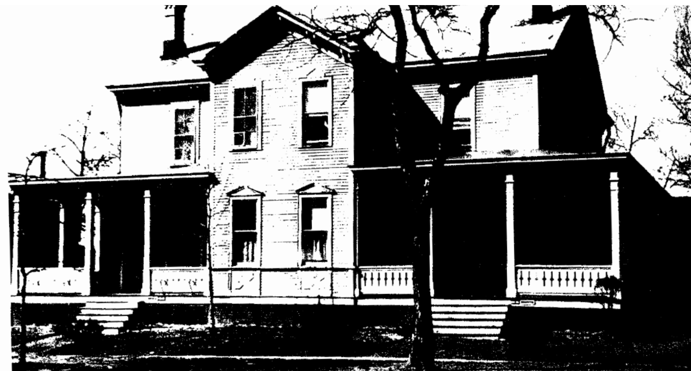
1934 - ORIGINAL WOOD SIDING VISIBLE
