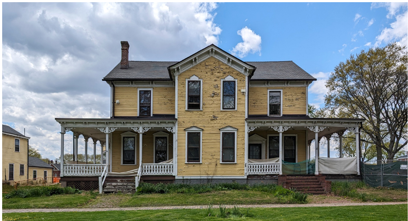
2024 - ASBESTOS SIDING REMOVED, ORIGINAL WOOD SIDING VISIBLE
