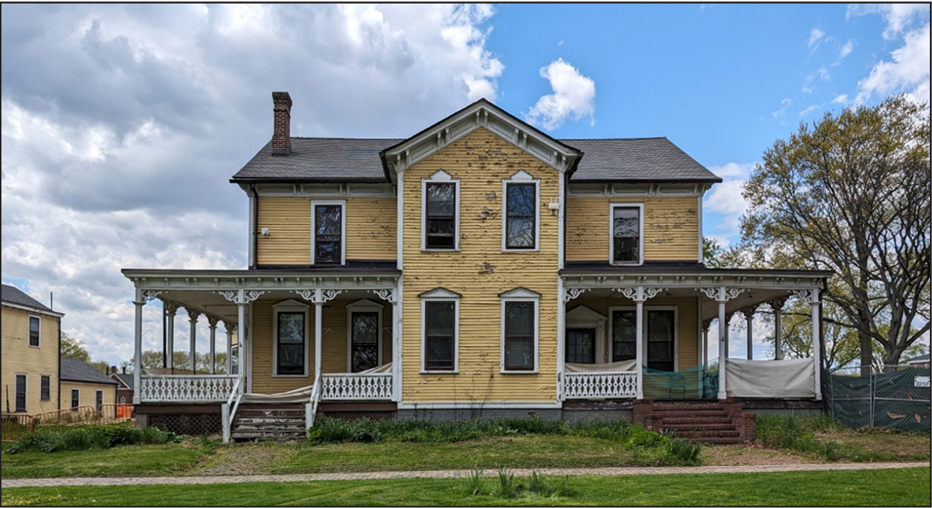
2024 - ASBESTOS SIDING REMOVED, ORIGINAL WOOD SIDING VISIBLE
