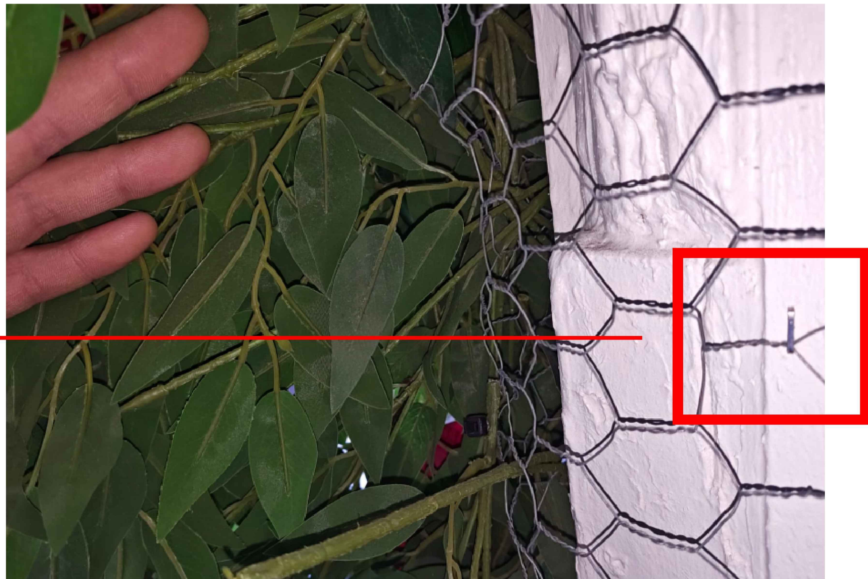
Mesh wiring secured with staple gun, stapled off to the side to prevent damage to molding.
