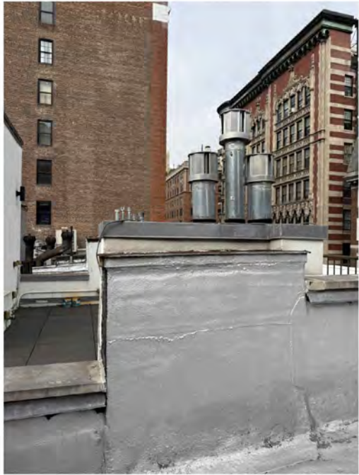
EXISTING EXHAUST DUCTS AT 52 EAST 66TH WILL BE MAINTAIN, EXISTING CHIMNEY FLUTE AT 54 EAST 66TH NOT IN USE, TO BE CAPPED.
