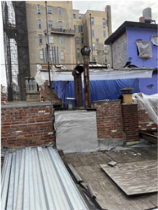
EXISTING EXHAUST FLUTE AT 54 EAST 66TH NOT IN USE, TO BE CAPPED.
