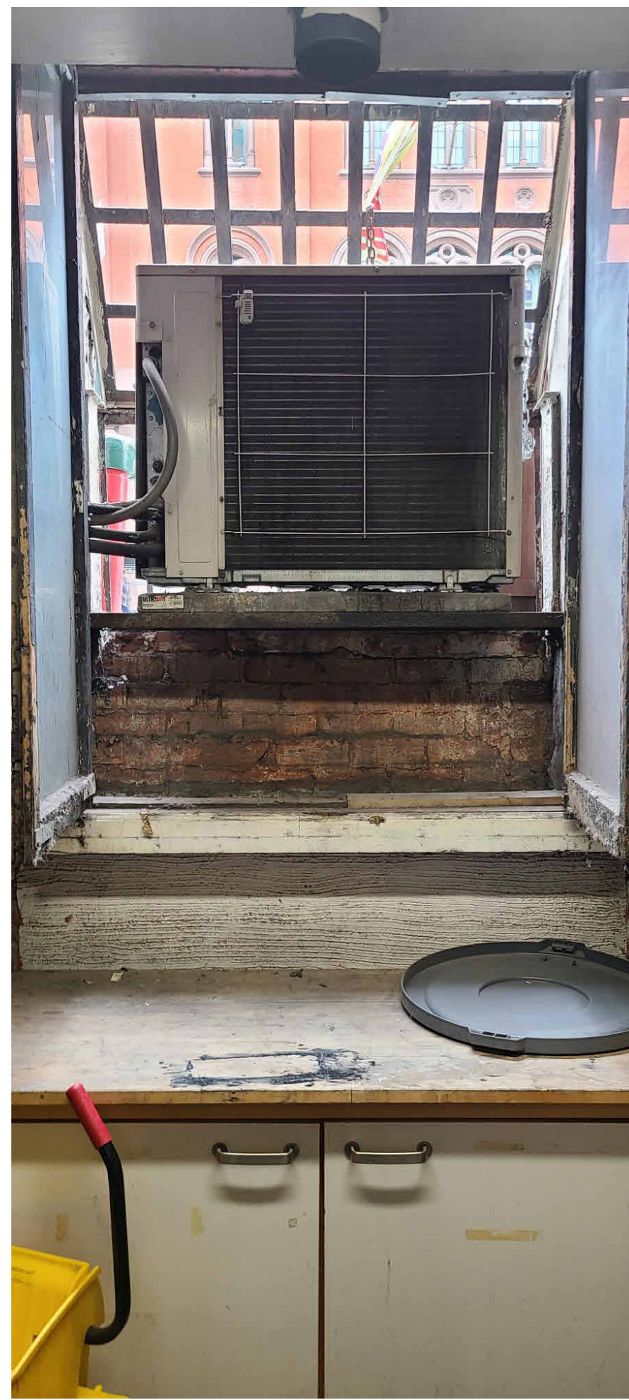
CURRENT PHOTO OF CELLAR WINDOW FROM INSIDE - CELLAR LEVEL
