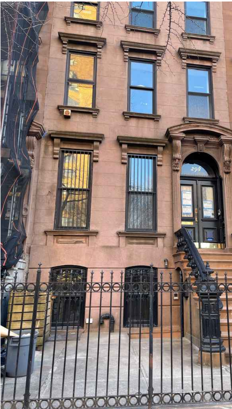
03 AREAWAY PAVING PHOTO 298 LAFAYETTE AVE.
