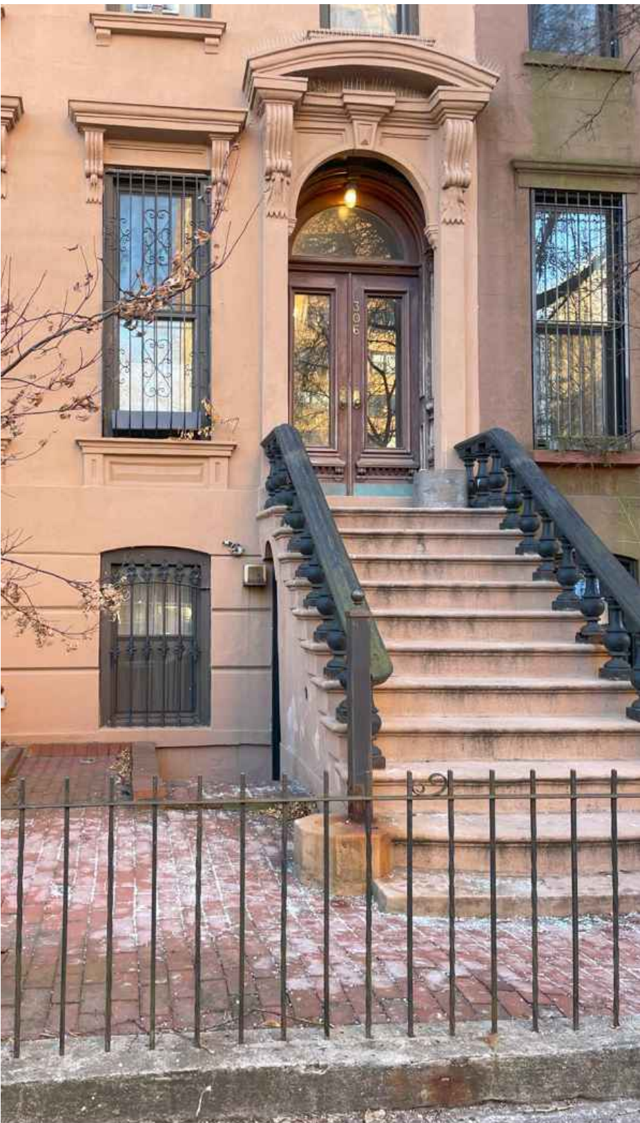
05 AREAWAY PAVING PHOTO 306 LAFAYETTE AVE.
