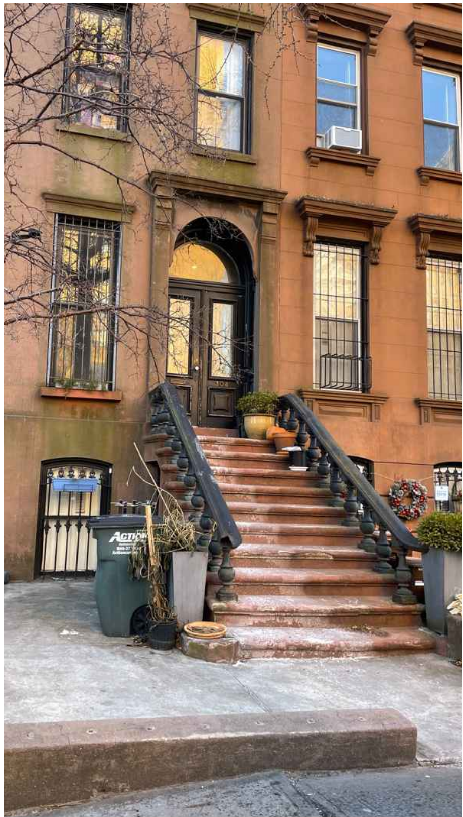
04 AREAWAY PAVING PHOTO 304 LAFAYETTE AVE.
