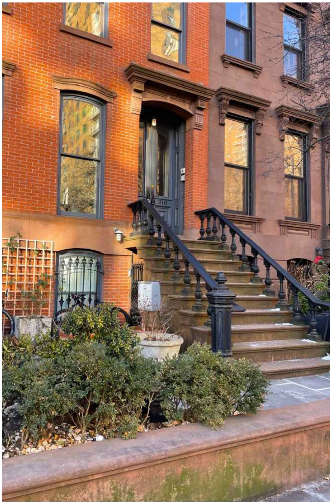
07 AREAWAY PAVING PHOTO 310 LAFAYETTE AVE.
