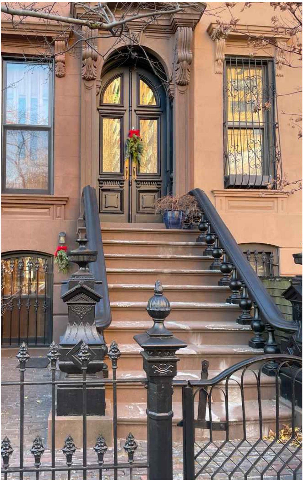
06 AREAWAY PAVING PHOTO 308 LAFAYETTE AVE.
