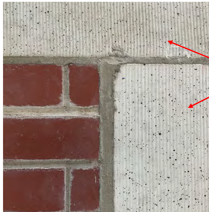
Ashlar Cladded Units South Elevation.
