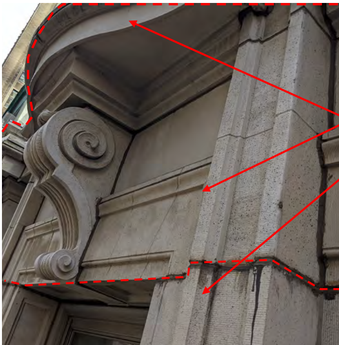
Water-Table and Window Head Units North Elevation.
