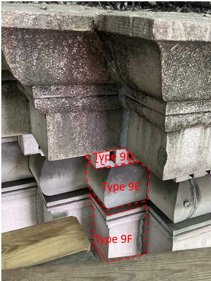
Photo: 9 North Elevation: 10/21/2024 North Setback Corner. Overall view: Type 9D, 9E, and 9F. Replacement in Cast Stone.
