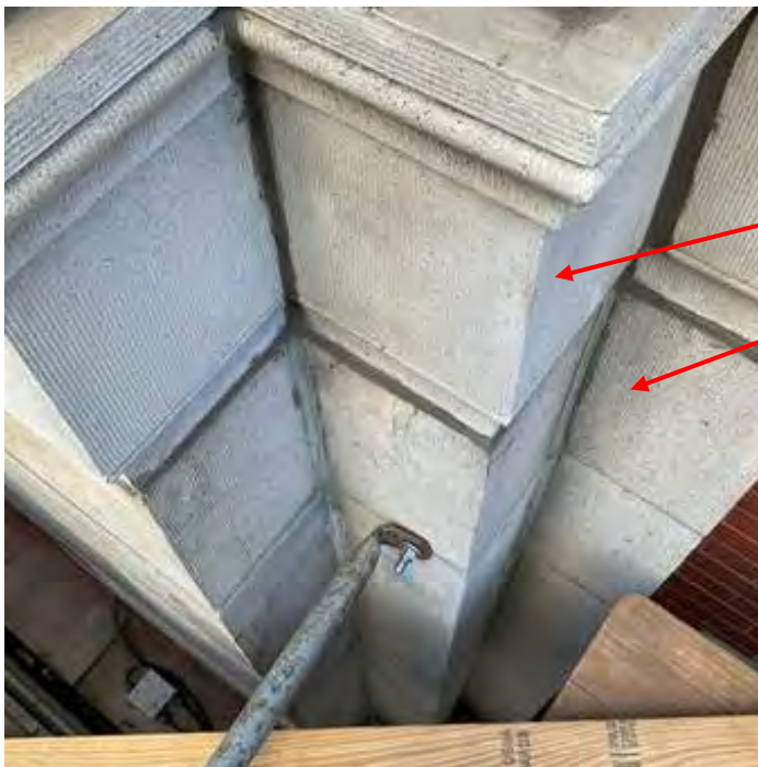
Water-Table Corner Units North Elevation.
