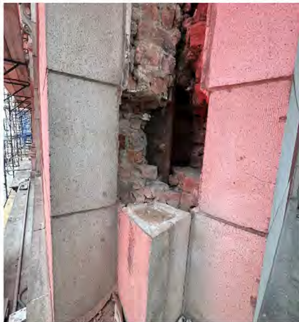
3 PROBE: EXISTING INSTALLATION OF TERRA COTTA AND STEEL CONDITION SCALE: N.T.S.
