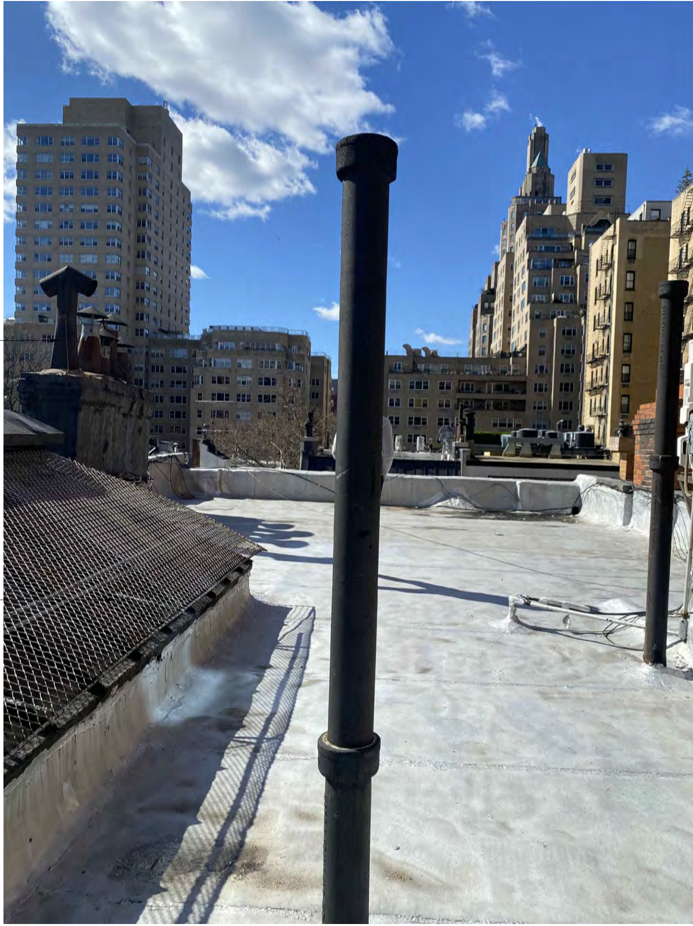
1 SITE PHOTOS: EXISTING ROOF VIEWING SOUTH NTS
