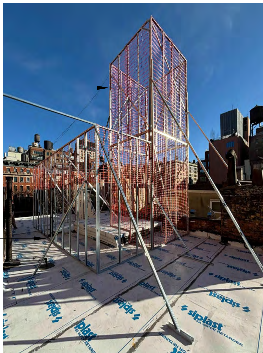
PHOTOS OF BULKHEAD & ELEVATOR SHAFT MOCKUP NTS
