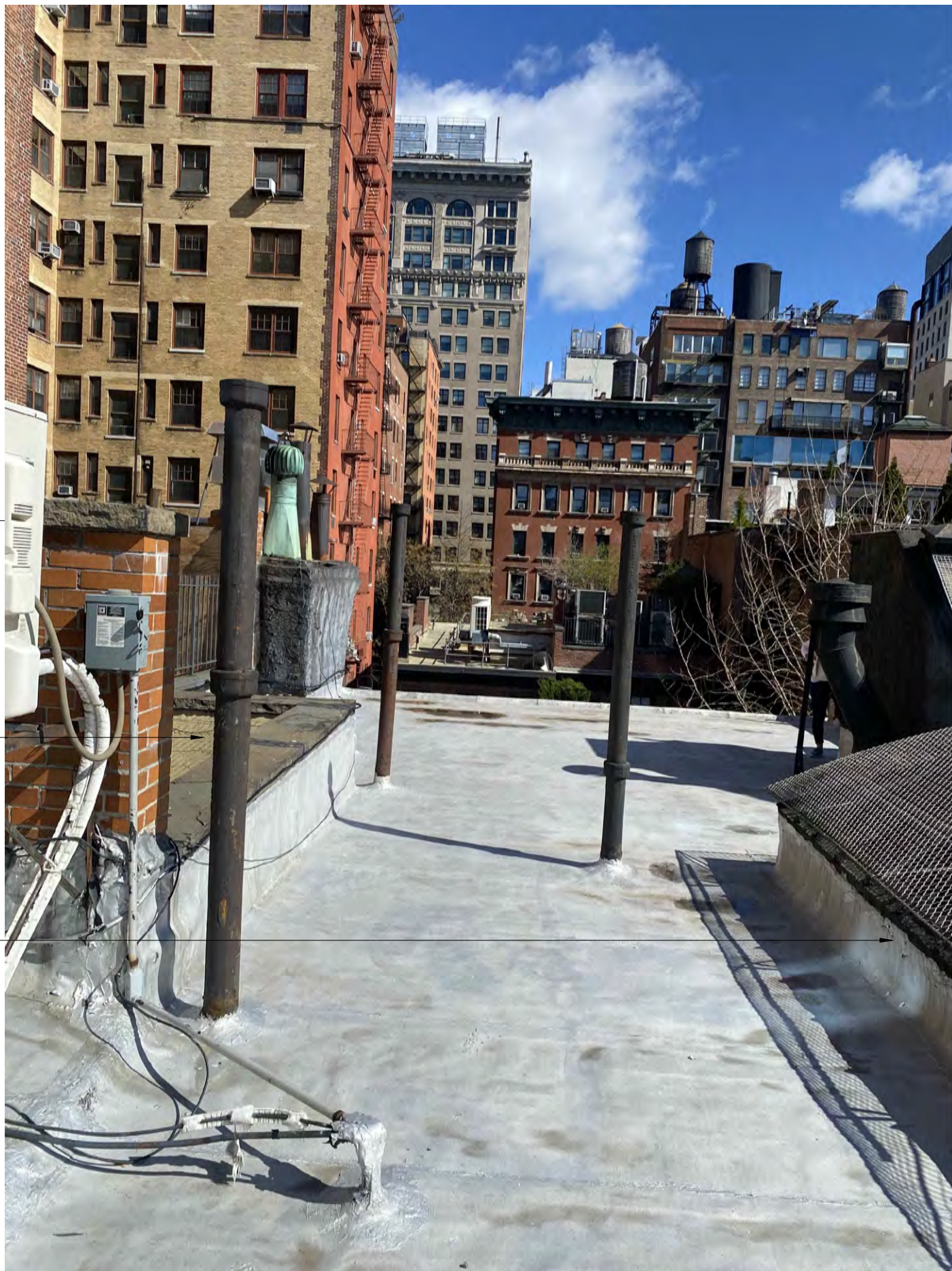
2 SITE PHOTOS: EXISTING ROOF VIEWING NORTH NTS
