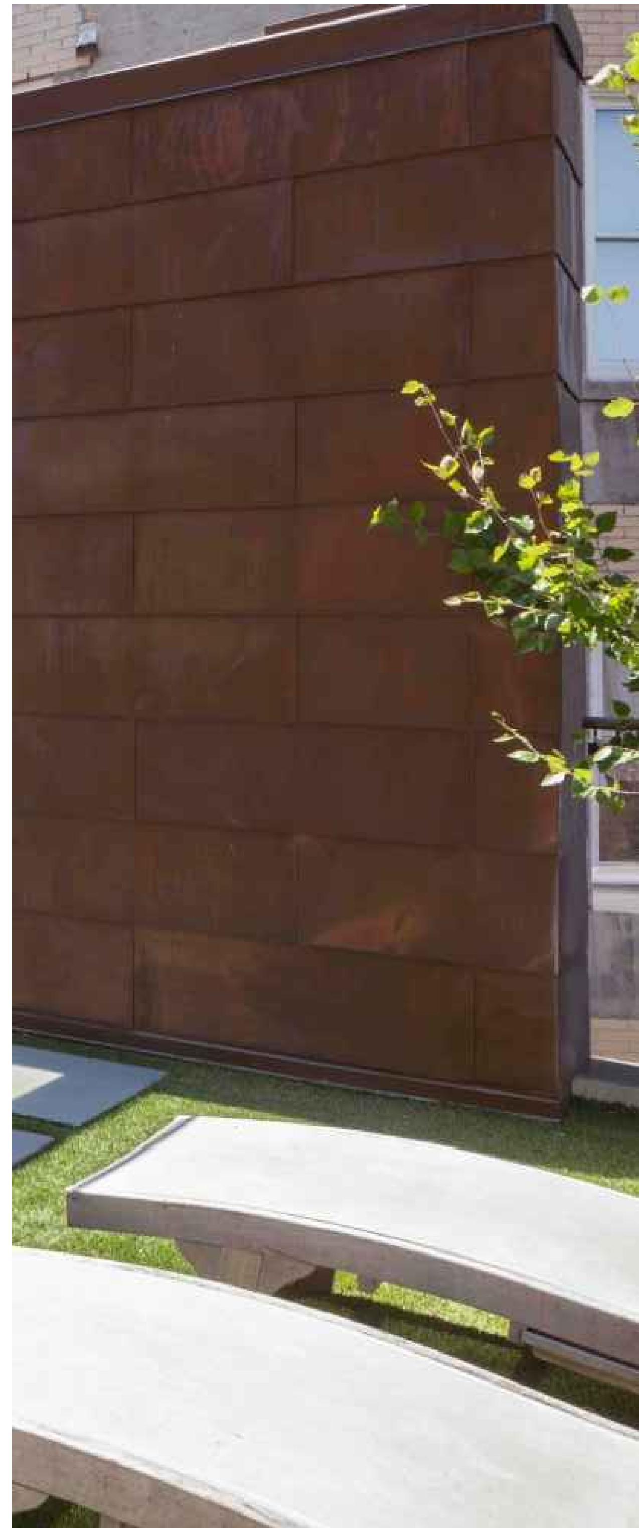
3 MATERIAL: COPPER PANEL CLADDING NTS
