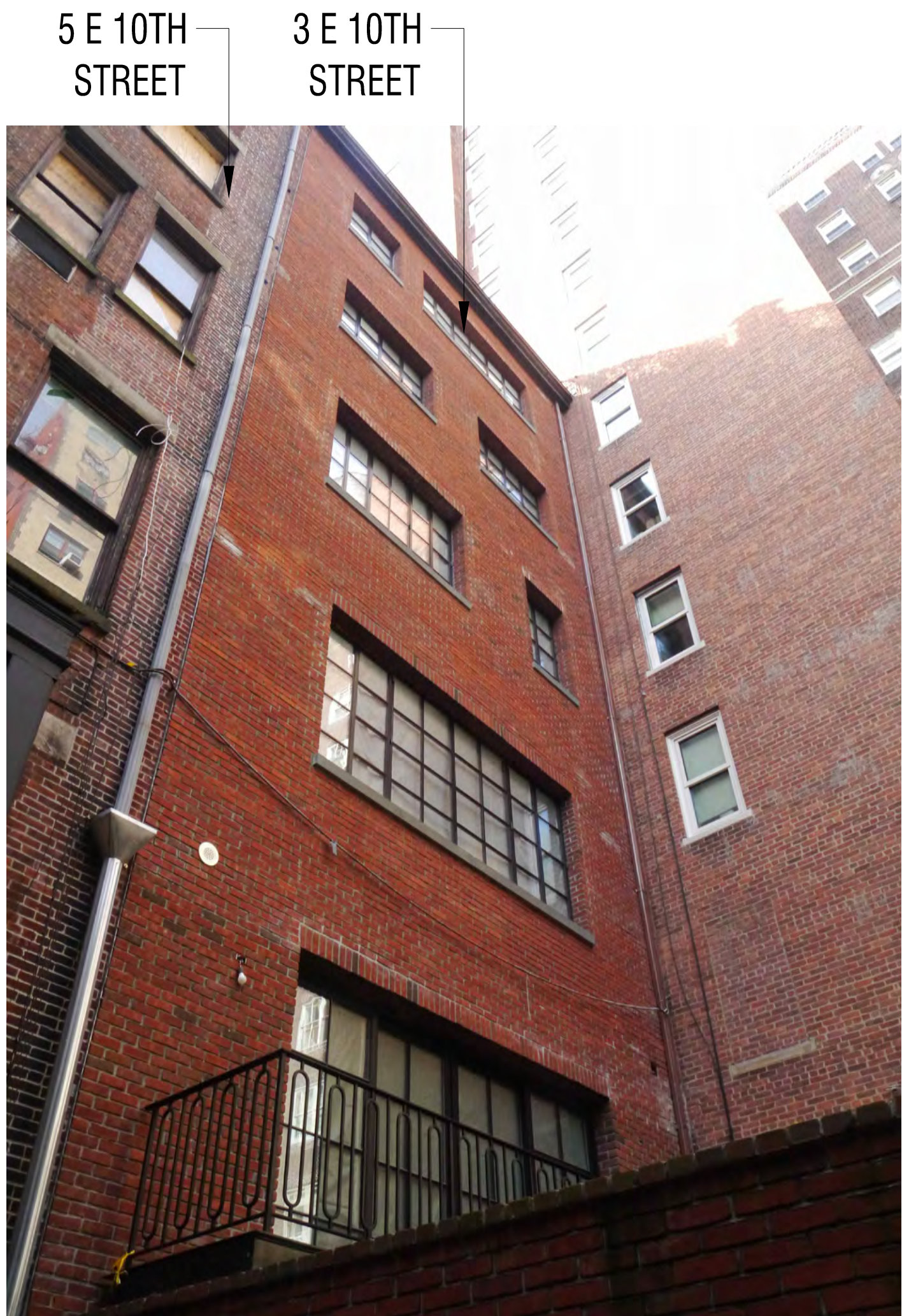
1 SITE PHOTOS: ADJACENT, 3 E 10TH STREET REAR FACADE NTS
