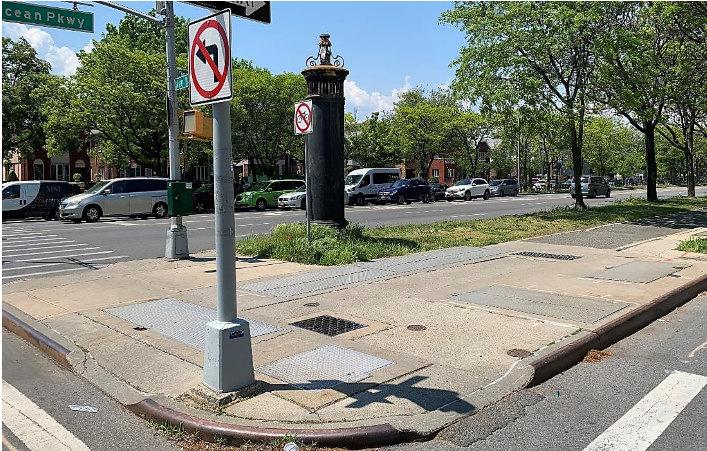
View northwest at air intake stack and flush hatches and vents on the median (May 2021)
