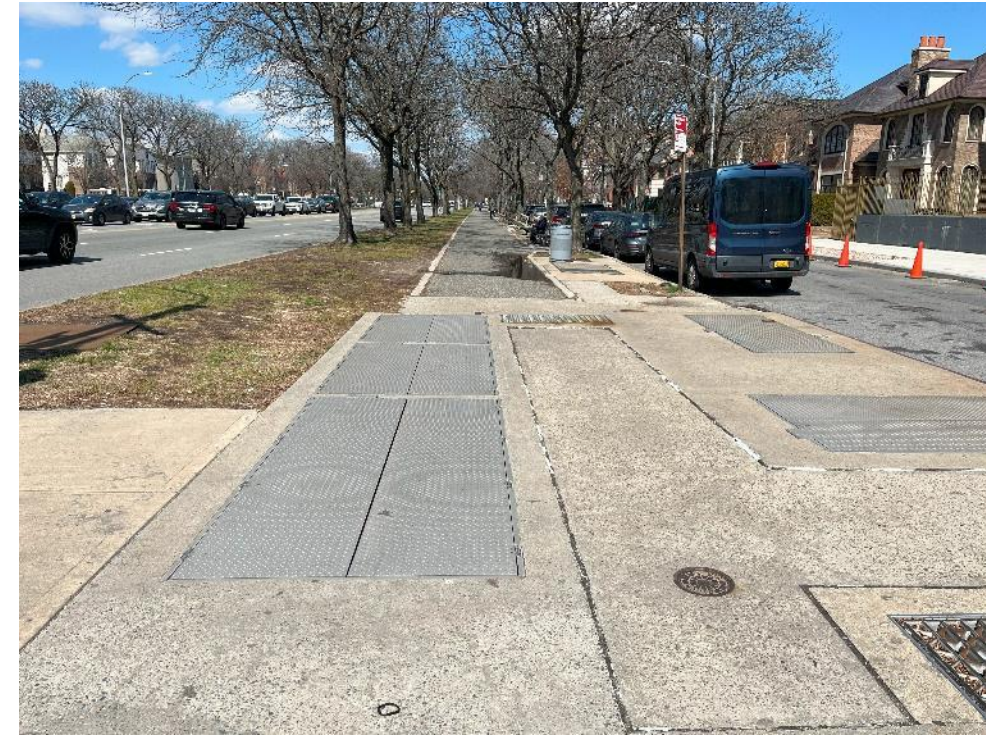
Detail of flush hatches to station below (March 2025)
