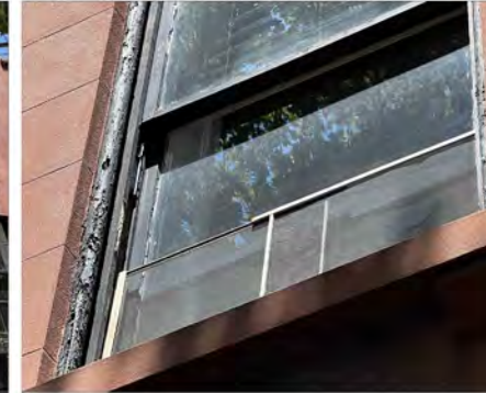
EXISTING 2" WOOD CUSTOM (VUE) BRICK MOLD - TO BE REPLACED IN KIND.
