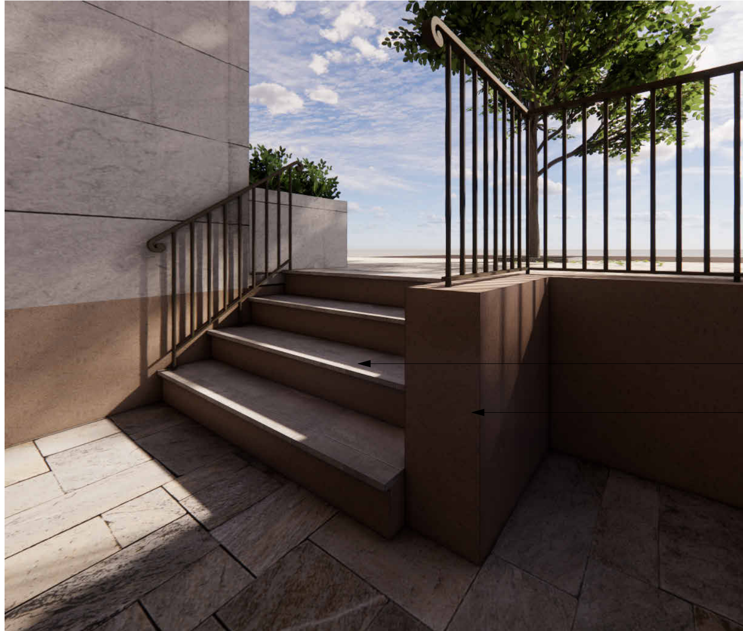
PROPOSED FRONT STAIR - NEW METAL HANDRAIL WITH DETAILS TO REPLICATE EXISTING GUARDS. PAINTED BLACK.
