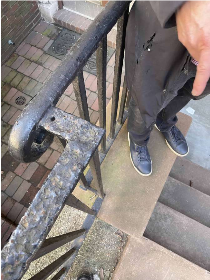
PHOTOGRAPHS OF EXISTING GUARDRAIL. REPLICATE DETAILING FOR NEW HANDRAIL IN PROPOSED CONFIGURATION.
