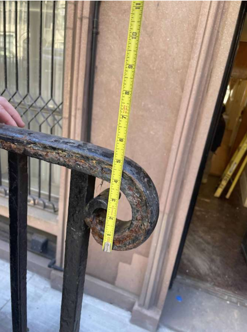
PHOTOGRAPHS OF EXISTING GUARDRAIL. REPLICATE DETAILING FOR NEW HANDRAIL IN PROPOSED CONFIGURATION.
