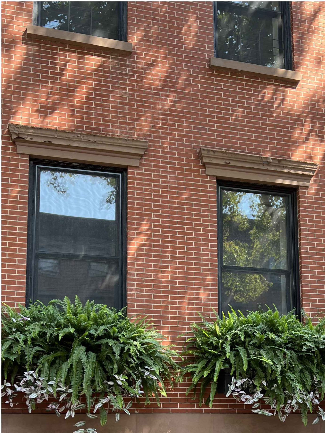
3 EXISTING FRONT WINDOWS & LINTELS LPC-04 SCALE: NTS
