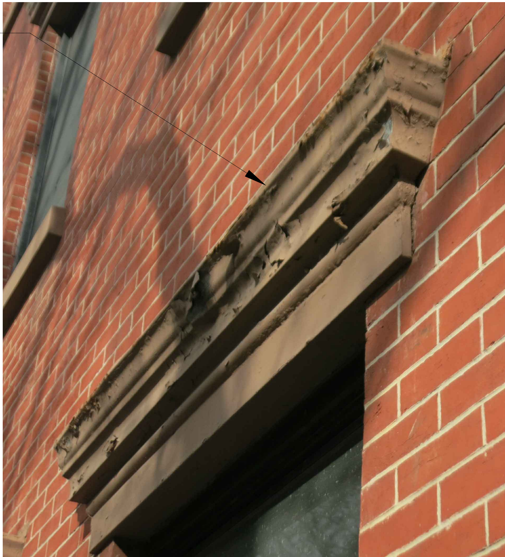
6 EXISTING SHEET METAL LINTELS LPC-04 SCALE: NTS
