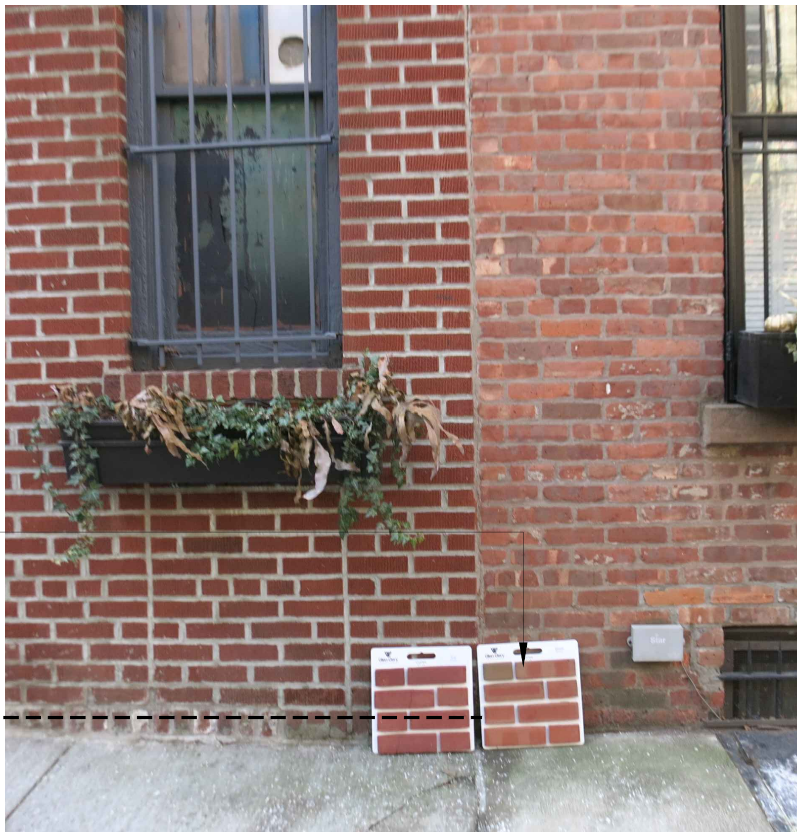
3 BRICK SELECTION PHOTO LPC-16 SCALE: NOT TO SCALE
