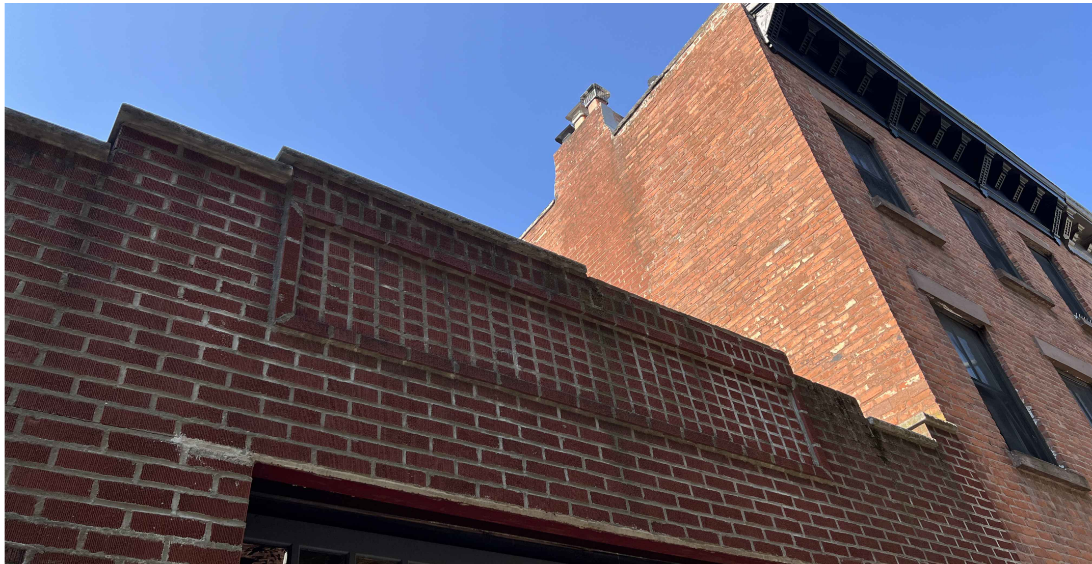
5 EXISTING STRIATED AND TAPESTRY BRICK PHOTO LPC-16 SCALE: NOT TO SCALE
