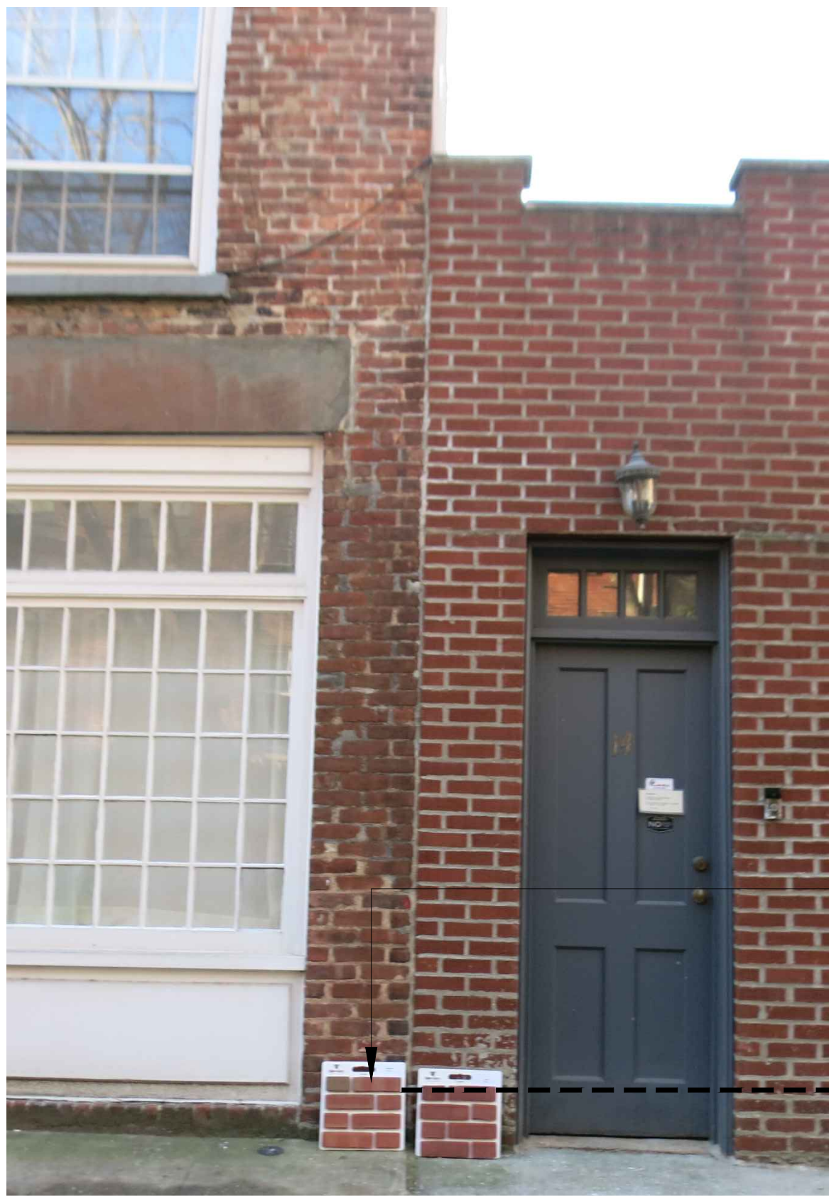
1 BRICK SELECTION PHOTO LPC-16 SCALE: NOT TO SCALE
