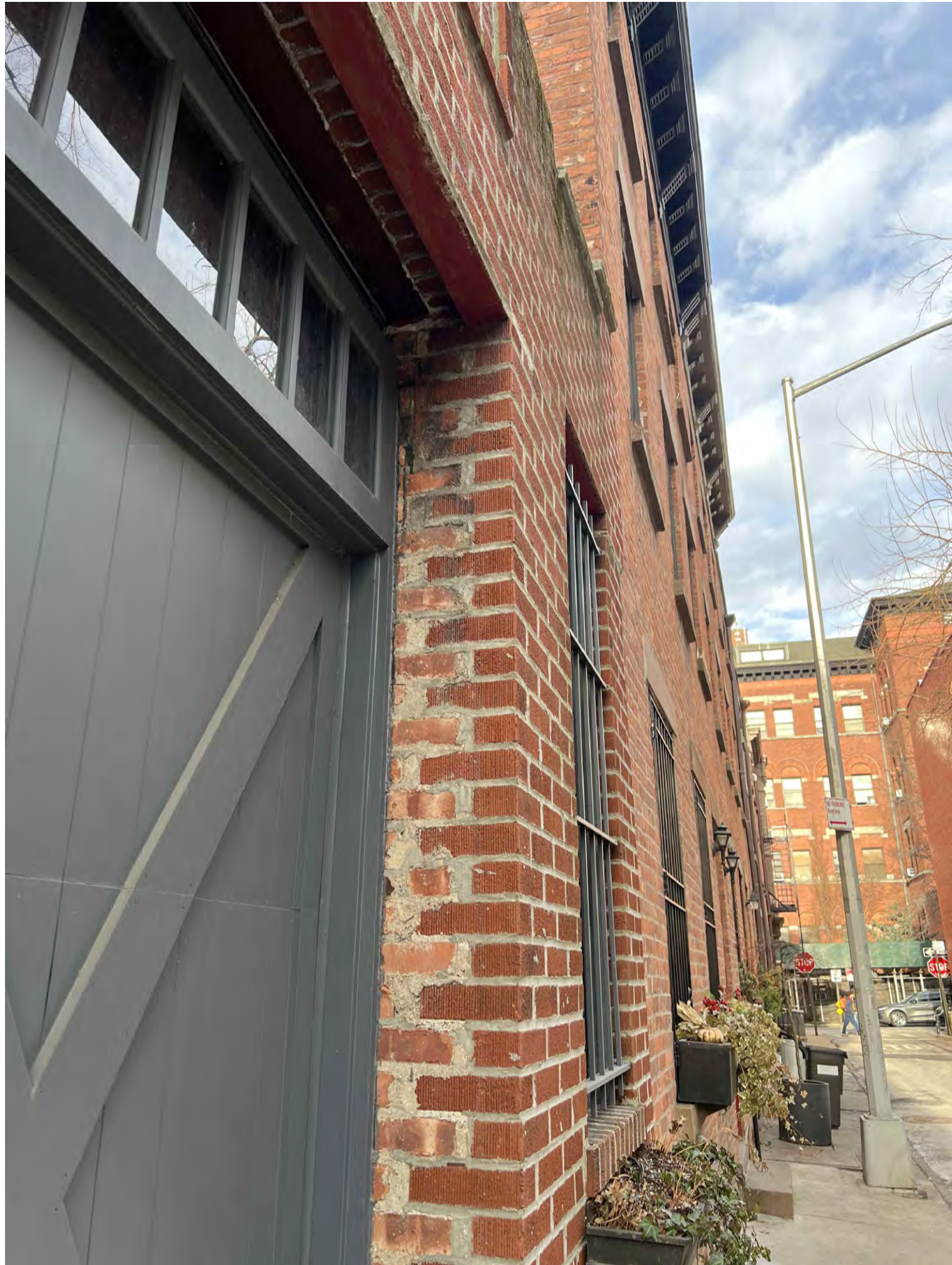
6 EXISTING MISMATCHED BRICK LPC-16 SCALE: NOT TO SCALE
