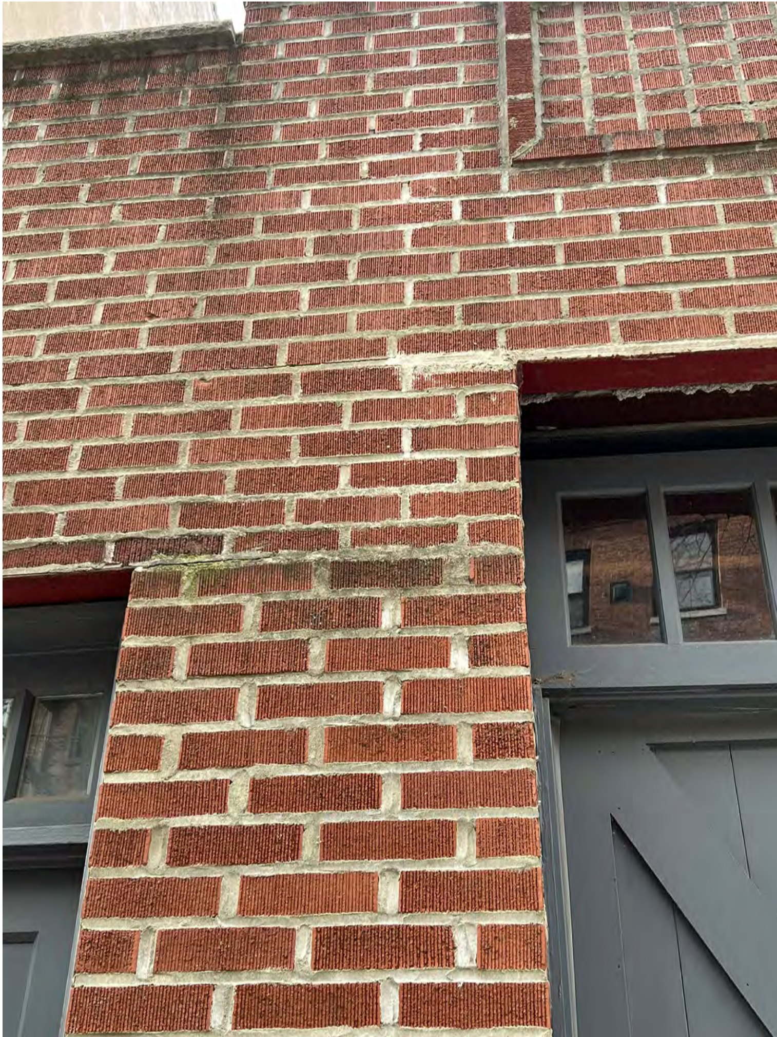
7 EXISTING STRIATED FACE BRICK LPC-16 SCALE: NOT TO SCALE
