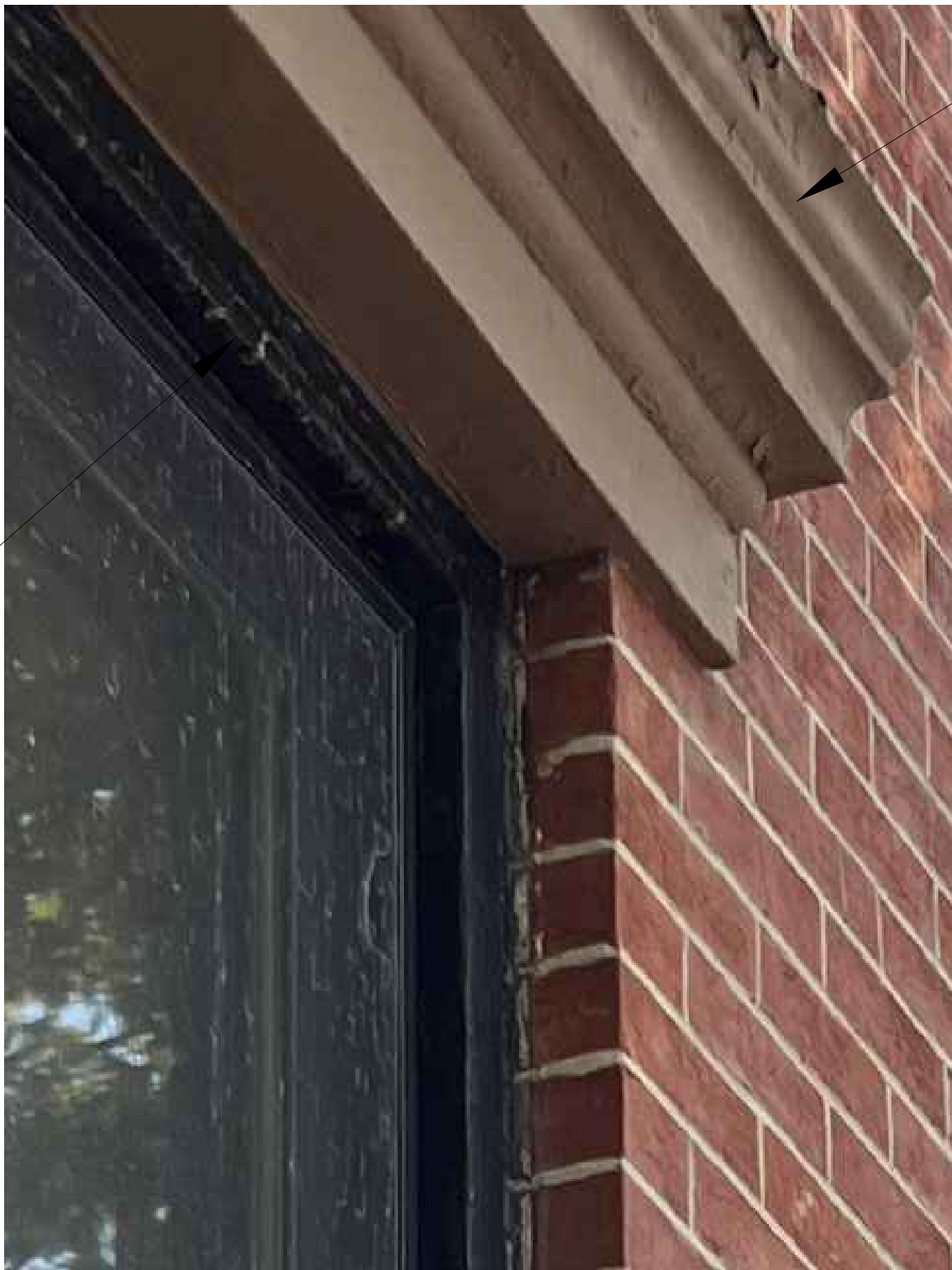
5 EXISTING BRICKMOLD LPC-04 SCALE: NTS
