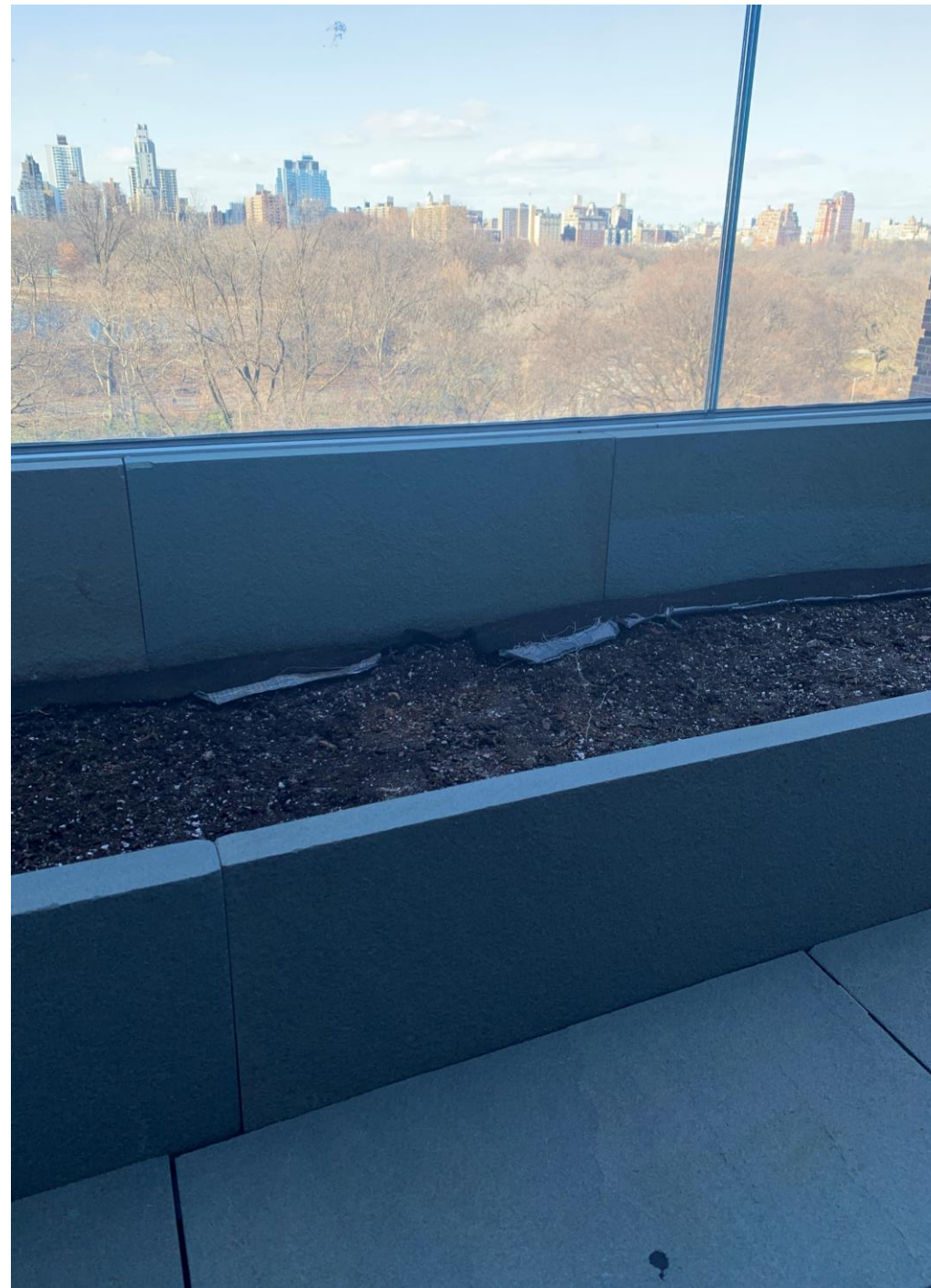
AS BUILT STONE TILE PLANTER AT BASE OF RAILING
