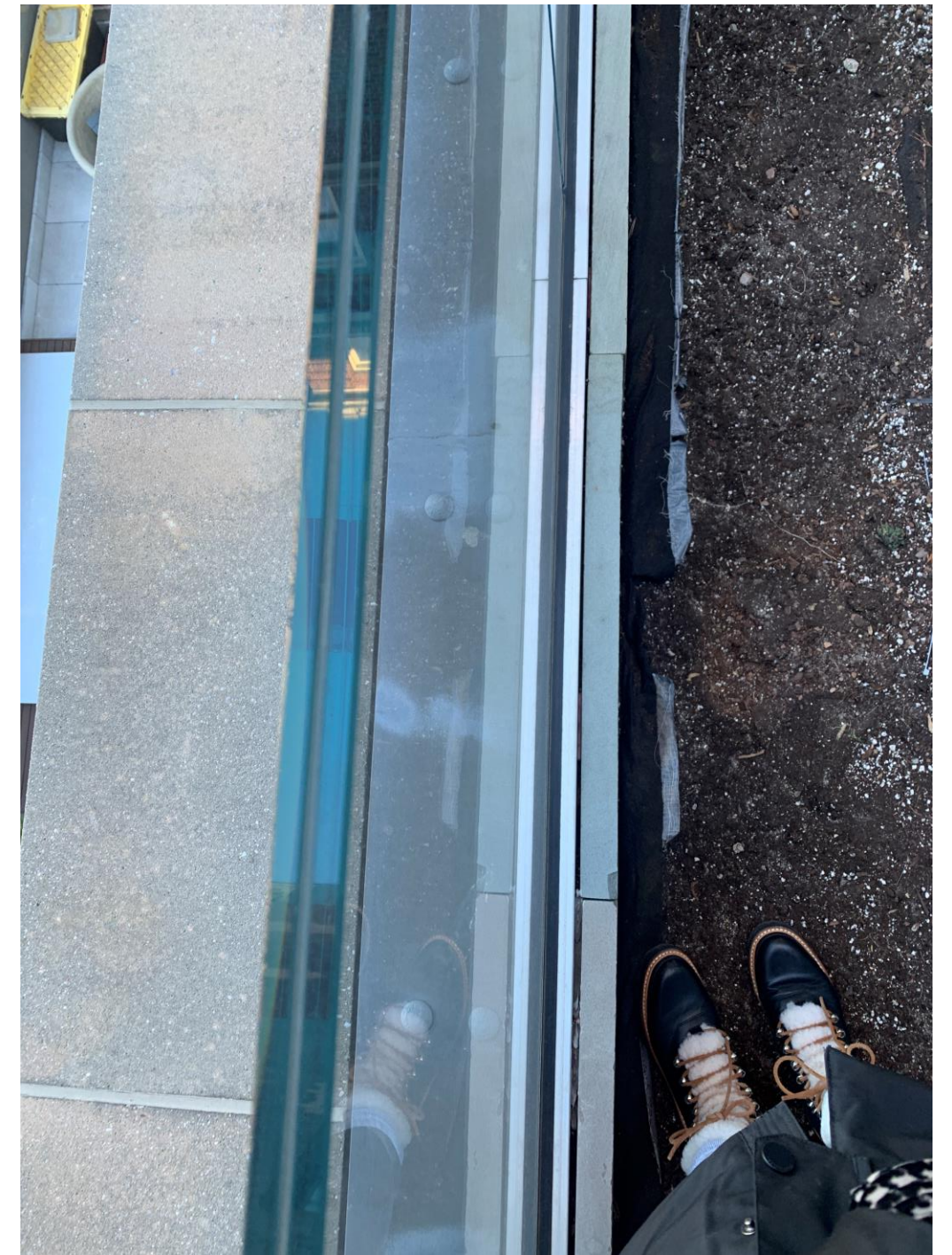
AS BUILT STAINLESS STEEL SHOE AND GLASS PANELS
