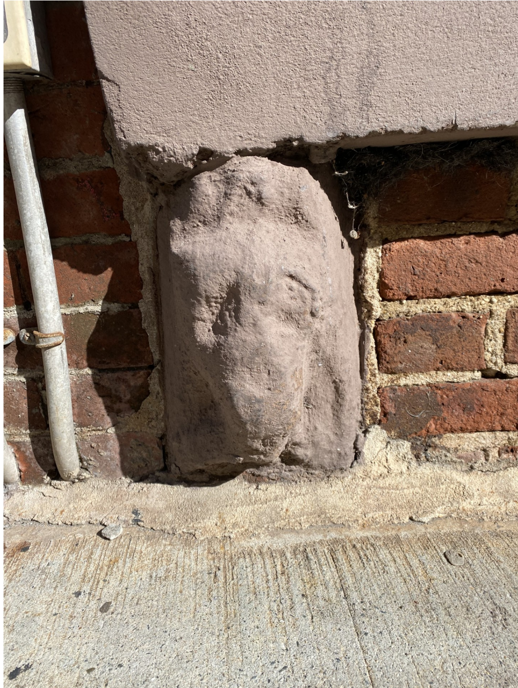
CLOSE-UP OF BRACKET BELOW LINTEL
