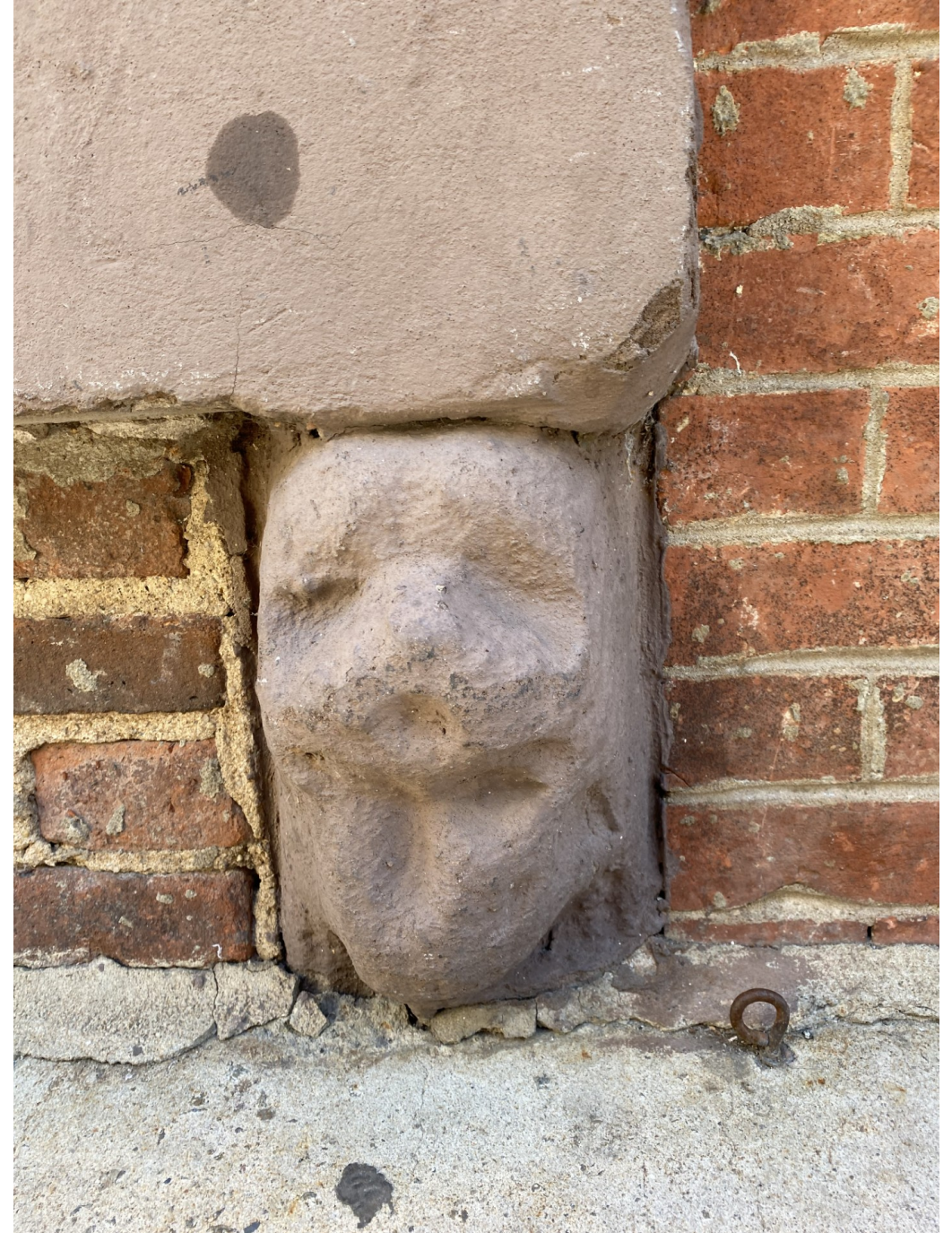
CLOSE-UP OF BRACKET BELOW LINTEL
