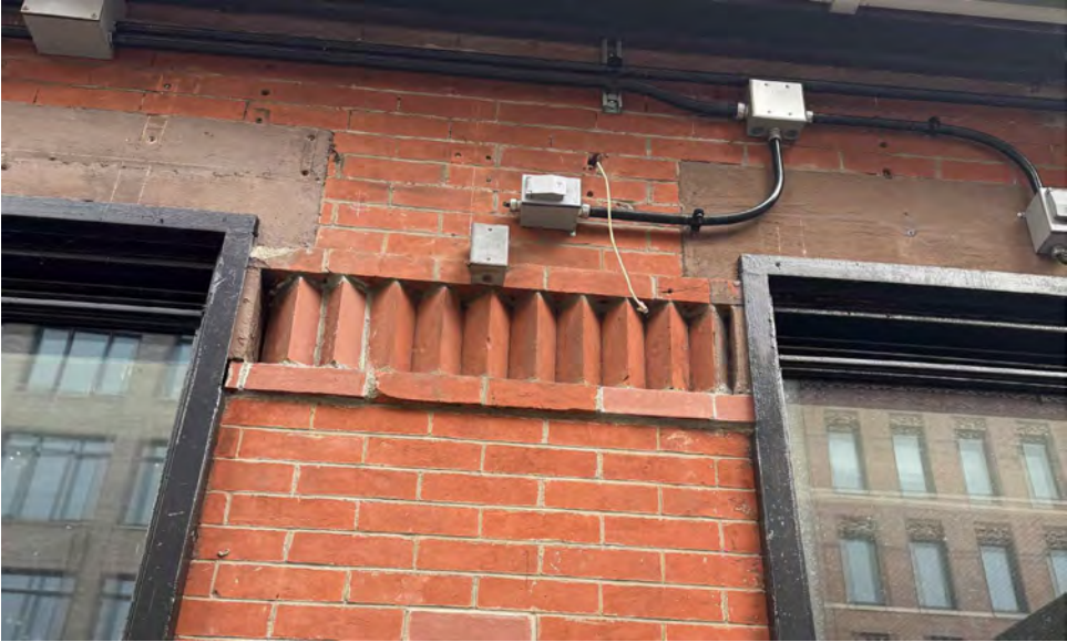
EXISTING SAWTOOTH DETAIL AT GANSEVOORT STREET
