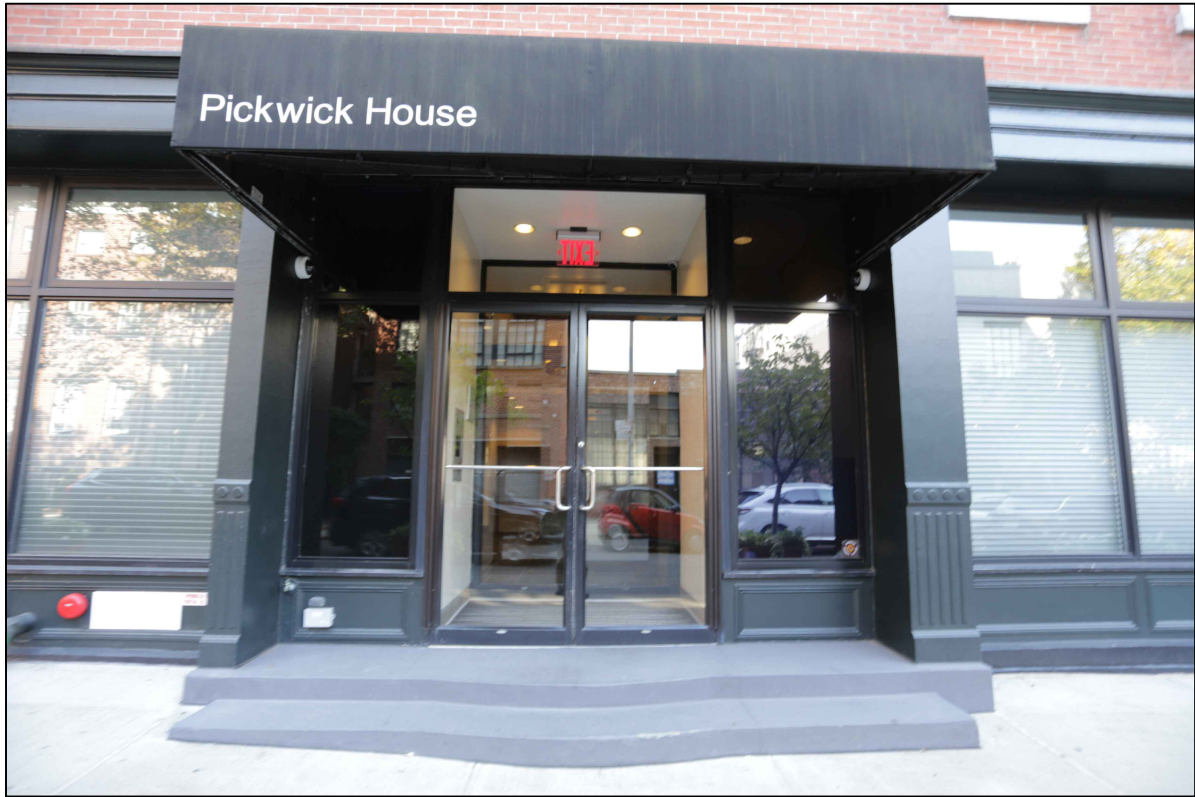
Entrance. Aluminum doors are 7'-4" high and are proposed to be replaced with doors 8'-0" high as this is the only door accessing the building.
