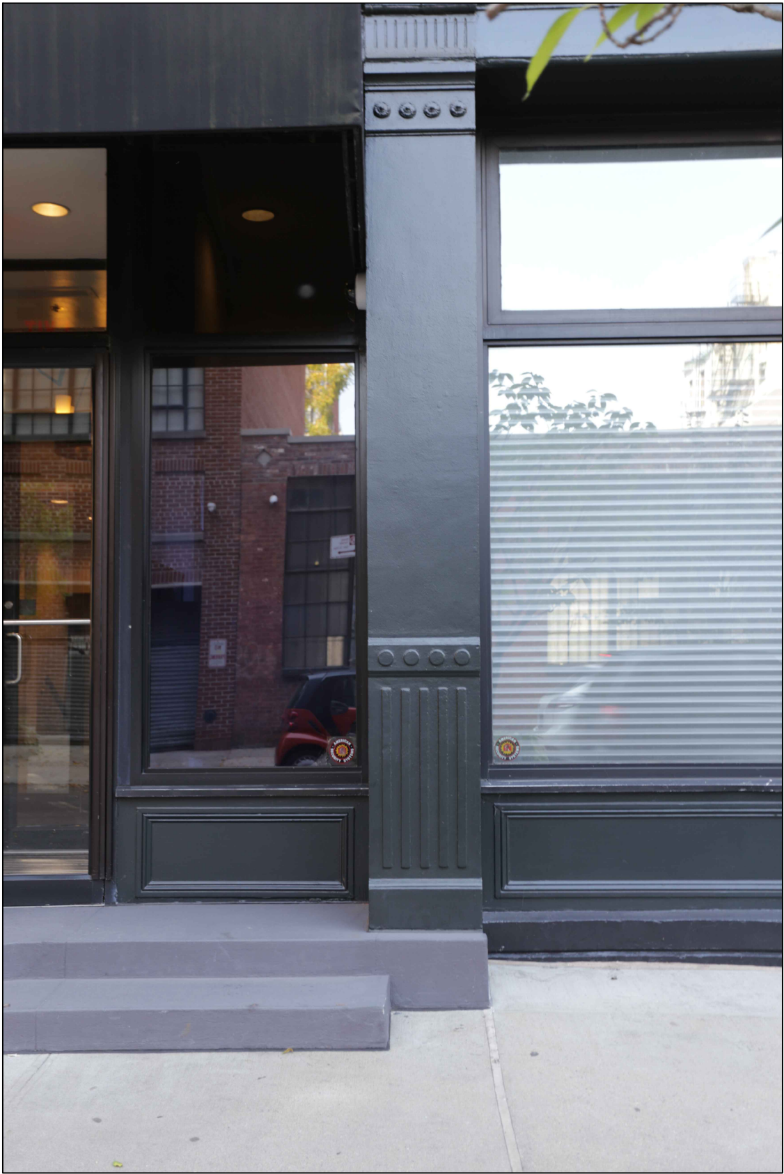
Comparative photograph of bulkhead at entrance and adjacent bay. Bulkheads are aluminum storefronts with wood bulkheads and applied wood panel moldings. Transom bars do not align.
