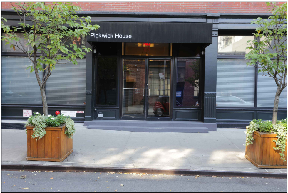
Entrance with aluminum doors and wood bulkhead to be removed and replaced with millwork based on the historic storefronts.
