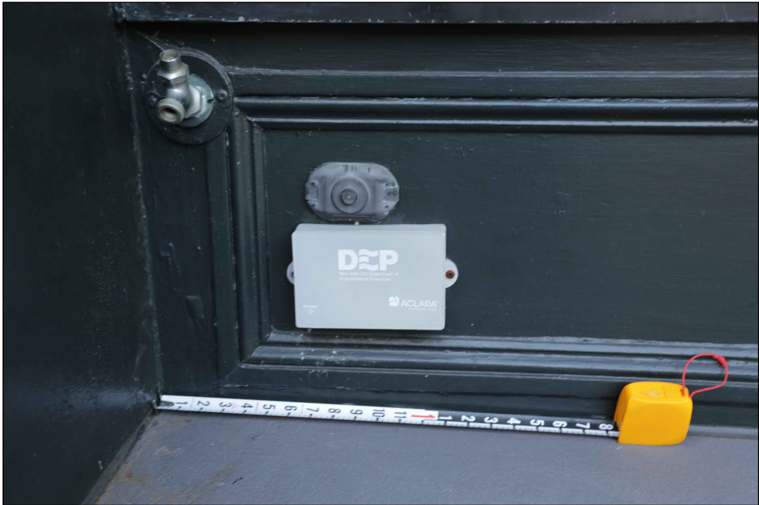
Detail photograph of the lower bulkhead infill, this area is wood with shallow applied wood panel molding with field-applied paint finish. Cast iron pier is at left.
