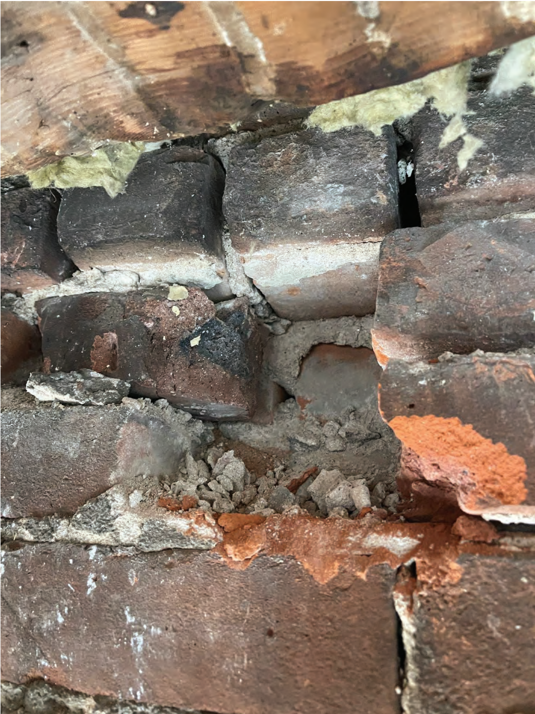
Photo # 3- Brick broken and missing with mortar turning to sand and dust.
