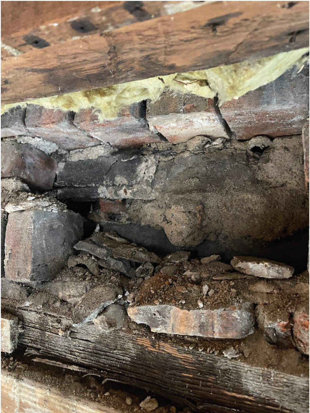
Photo # 1- Missing bricks and mortar with air pockets in each joints.
