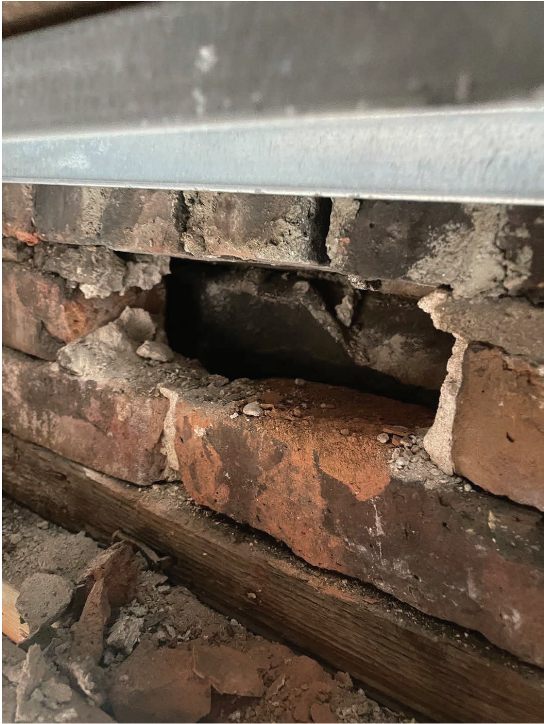
Photo # 2- Missing bricks, compromised mortar joints, decomposed mortar
