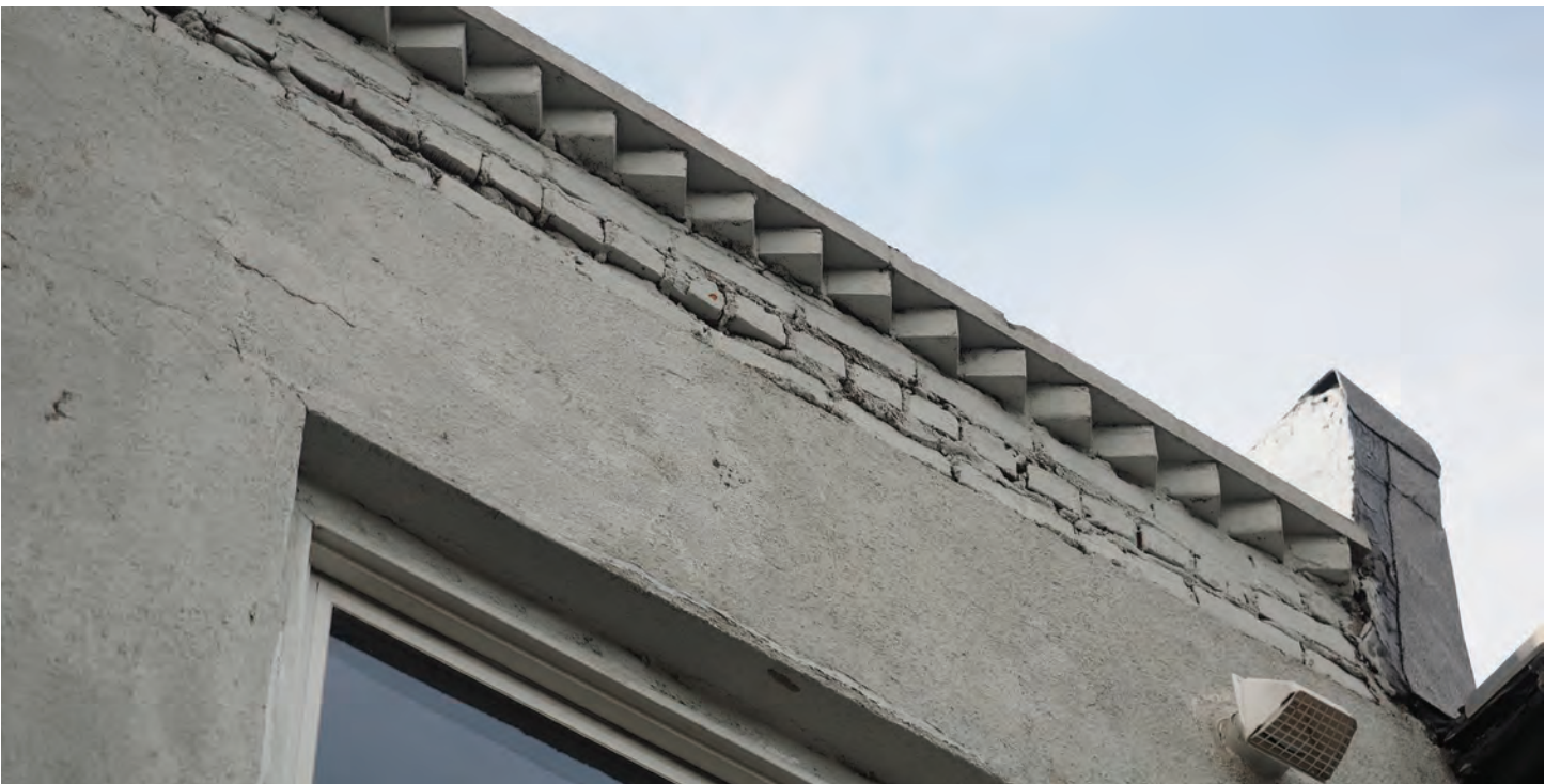
Detail of existing, non-historic rear cornice condition
