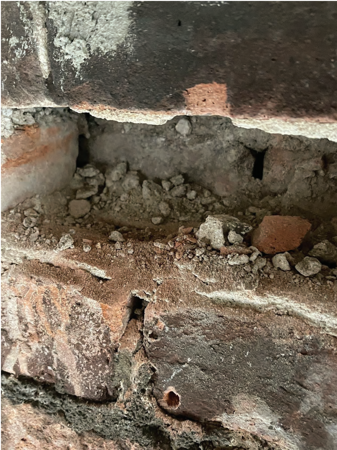
Photo # 4- Cracking separation between bricks, decomposed mortar
