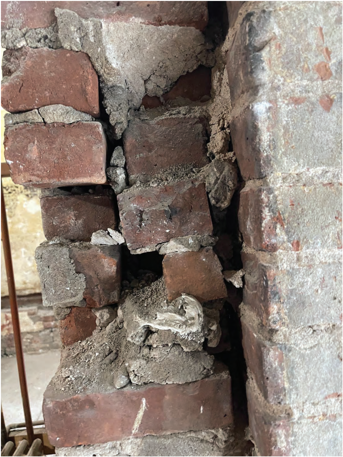
Photo # 5- Cracking, missing and separation between bricks, loss of mortar.
