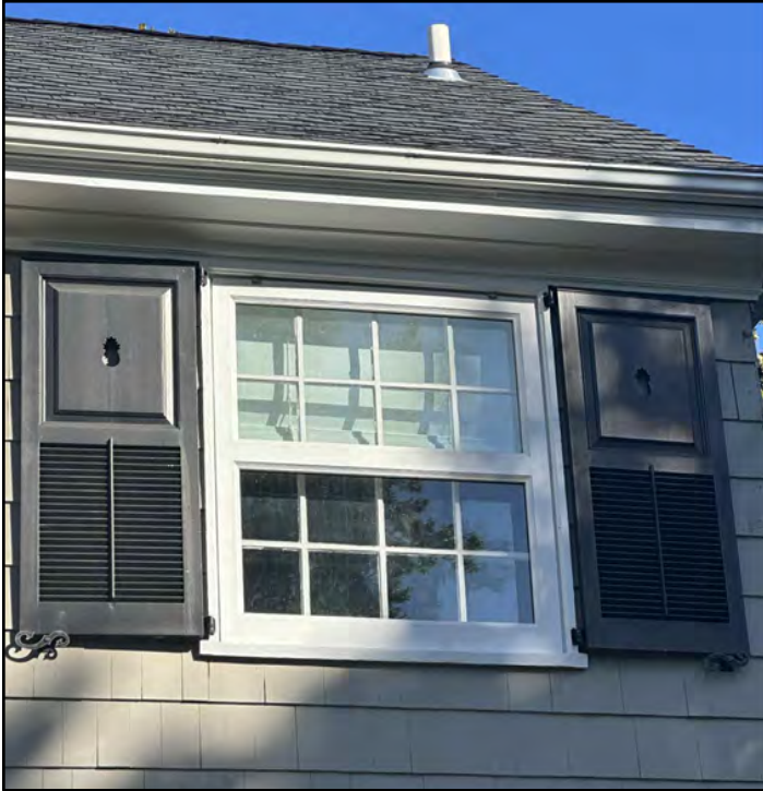
WINDOW TYPE "M" — 4'-0" X 4'-5 1/2" DOUBLE HUNG WINDOW EXISTING: 3 VERTICAL PROFILES, 1 HORIZONTAL PROFILE PER STASH PROPOSED: 3 VERTICAL PROFILES, 1 HORIZONTAL PROFILE PER STASH
