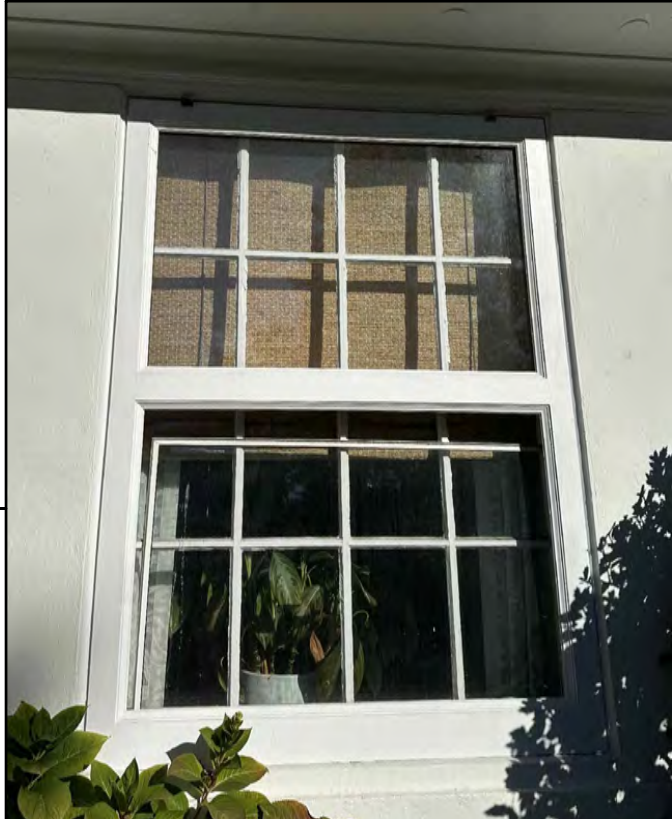
WINDOW TYPE "B" — 4'-0" X 4'-5 1/2" DOUBLE HUNG WINDOW EXISTING: 3 VERTICAL PROFILES, 1 HORIZONTAL PROFILE PER STASH PROPOSED: 3 VERTICAL PROFILES, 1 HORIZONTAL PROFILE PER STASH
