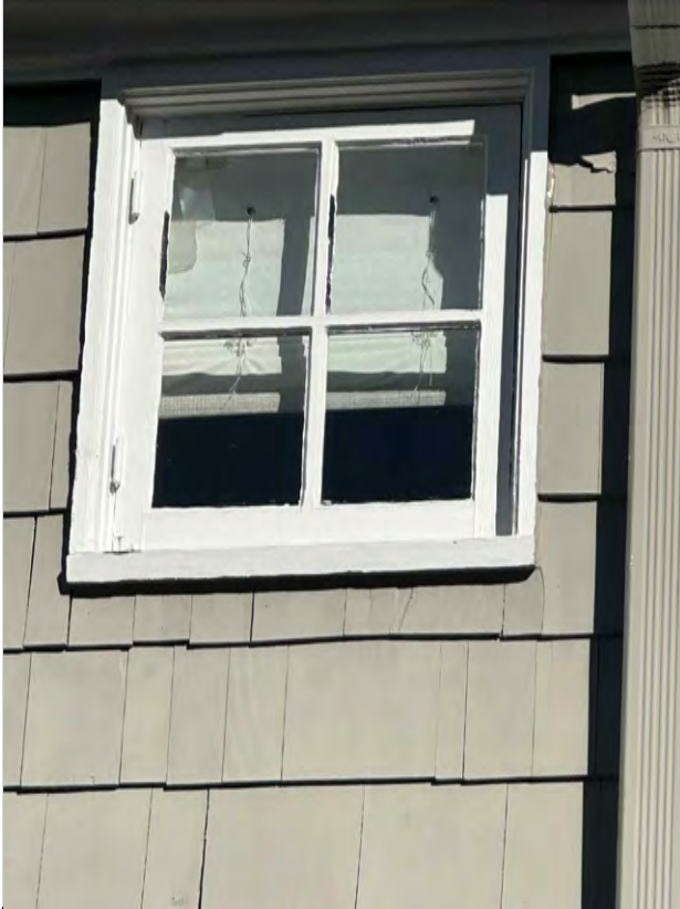
WINDOW TYPE "N" — 2'-0 1/2" X 2'-6" CASEMENT WINDOW EXISTING: 1 VERTICAL PROFILE, 1 HORIZONTAL PROFILE PROPOSED: 1 VERTICAL PROFILE, 1 HORIZONTAL PROFILE
