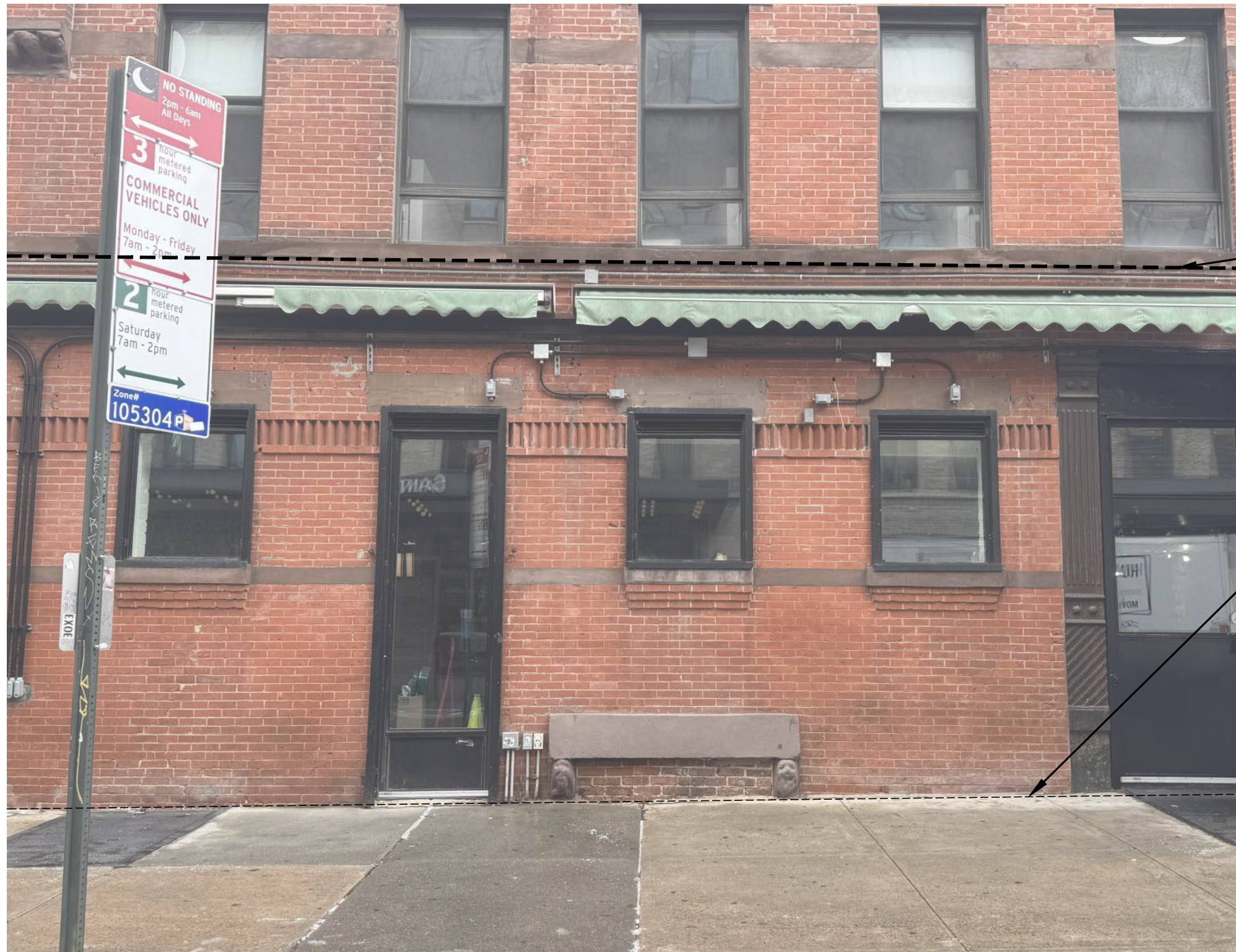
VIEW FROM GANSEVOORT STREET FACING NORTH
