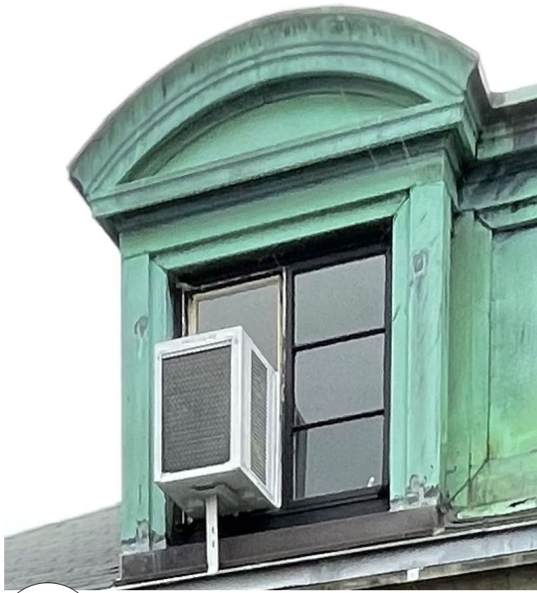
P1 DETAIL VIEW at CASEMENT WINDOW WITH A/C UNIT A/C TO BE REMOVED & WINDOW RESTORED
