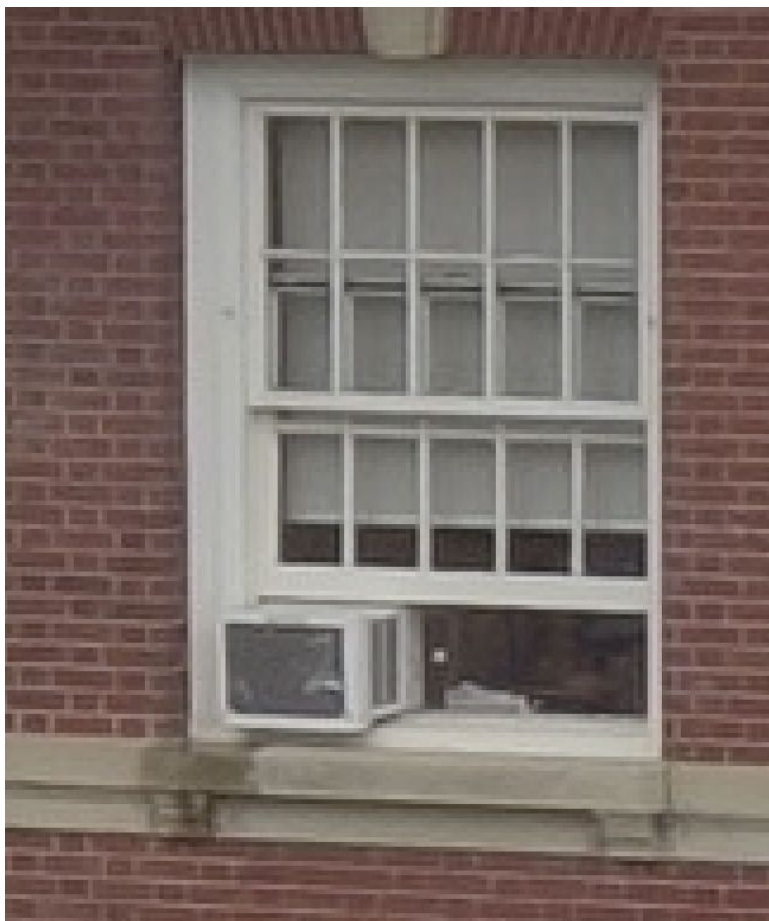
P2 DETAIL VIEW at DH WINDOW WITH A/C UNIT A/C TO BE REMOVED & WINDOW RESTORED
