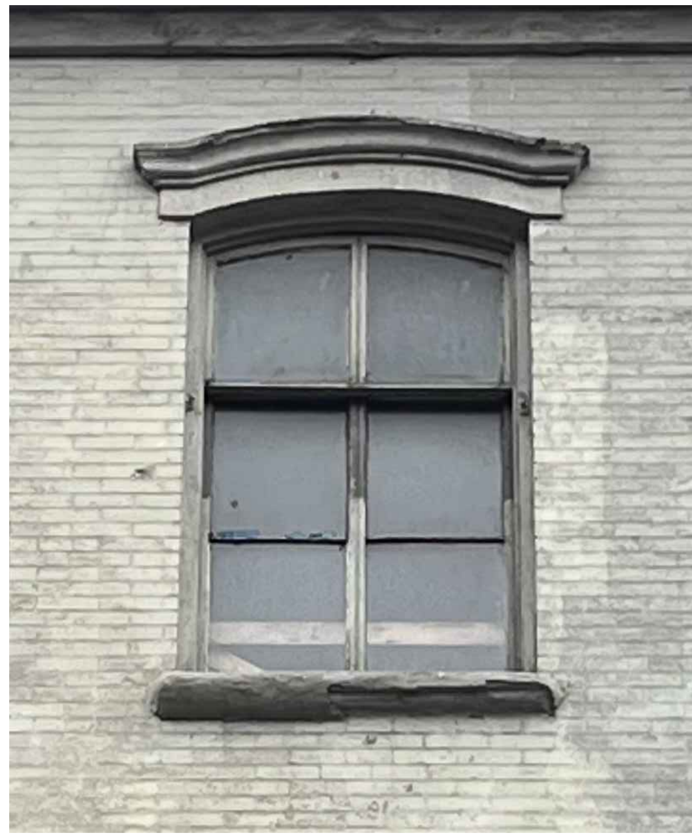
4 EXIST. SINGLE-HUNG (114) ON 3RD FLOOR: 3
