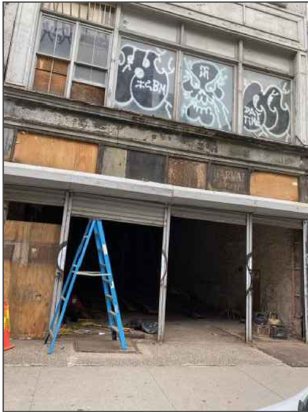
2 STOREFRONT AT 114 CHAMBERS ST
