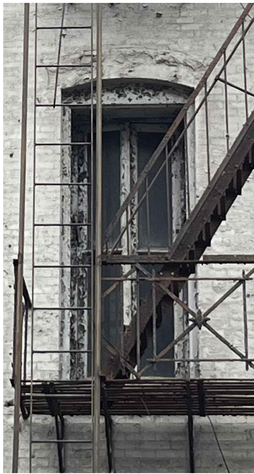
2 EXIST. FRENCH DOOR (112) ON 2ND FLOOR: 1 ON 3RD FLOOR: 1 ON 4TH FLOOR: 1
