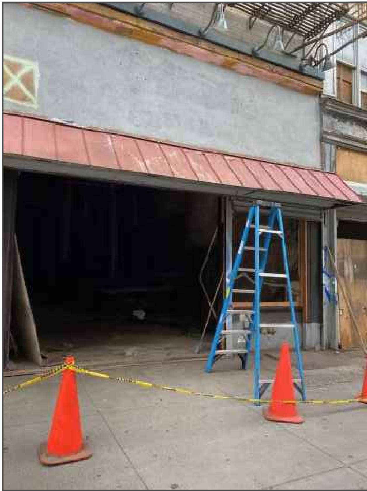
1 STOREFRONT AT 112 CHAMBERS ST
