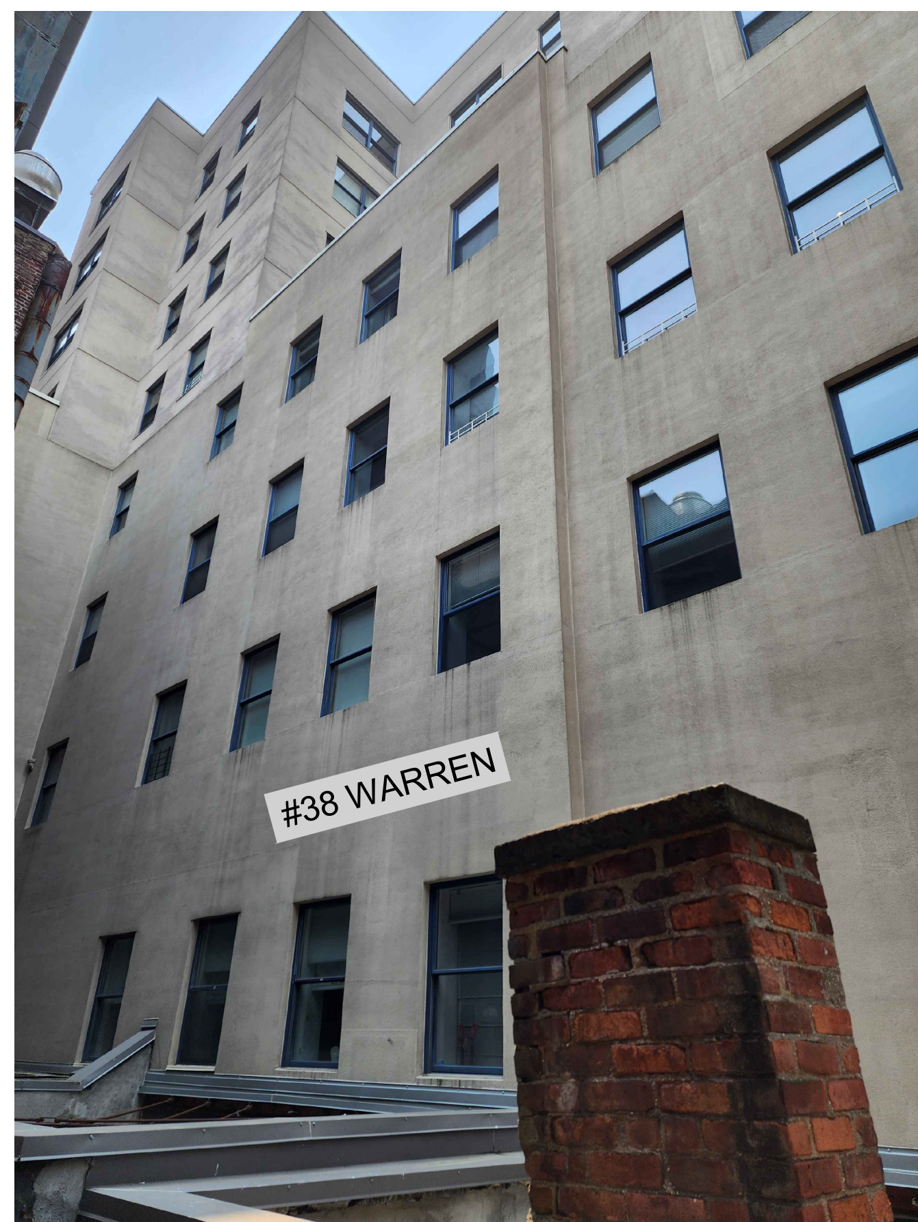
4 EXISTING NEIGHBOR'S REAR FACADES
