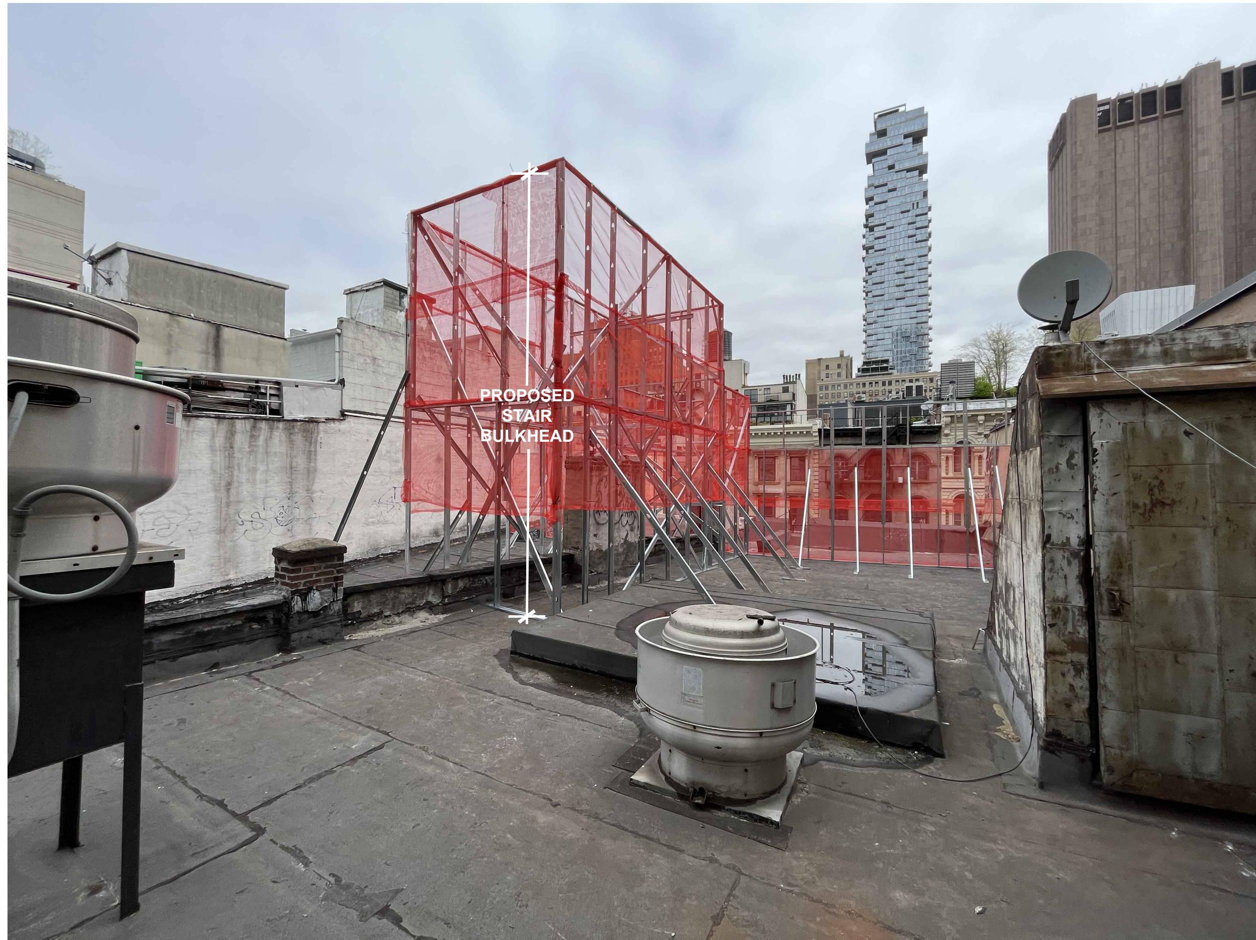
3 VIEW FROM BACK OF ROOF - WITH MOCKUP
