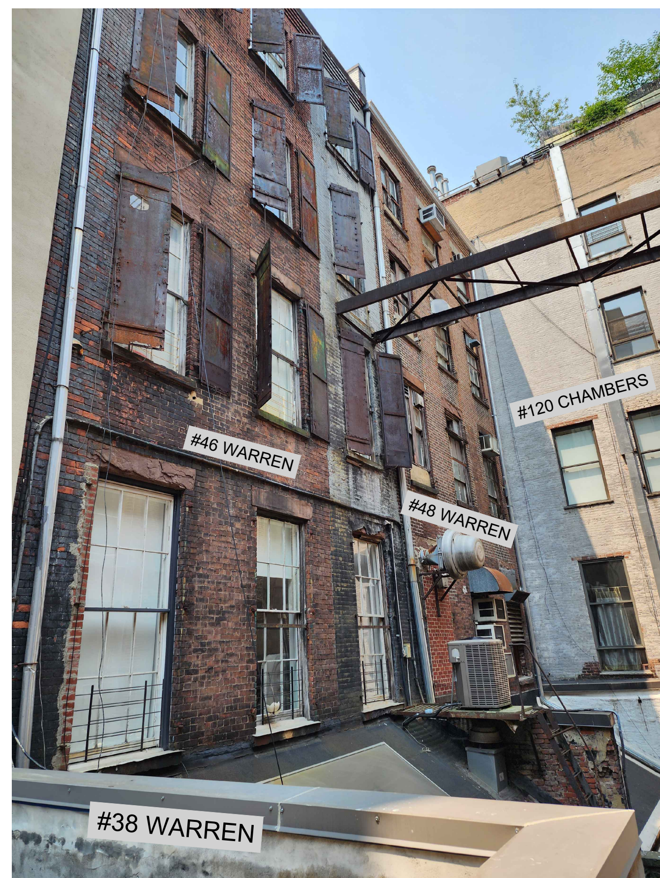
5 EXISTING NEIGHBOR'S REAR FACADES
