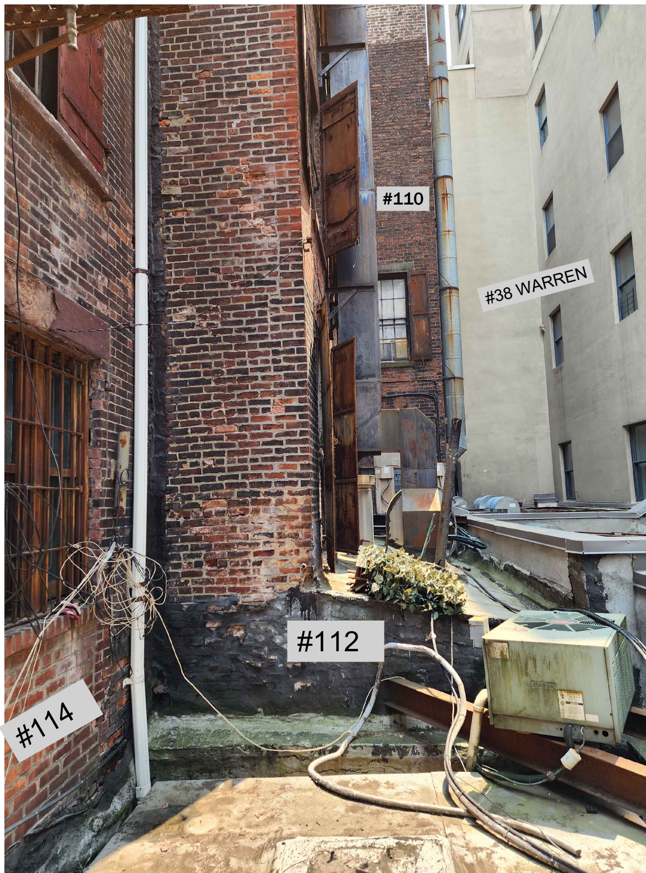
3 EXISTING REAR FACADE
