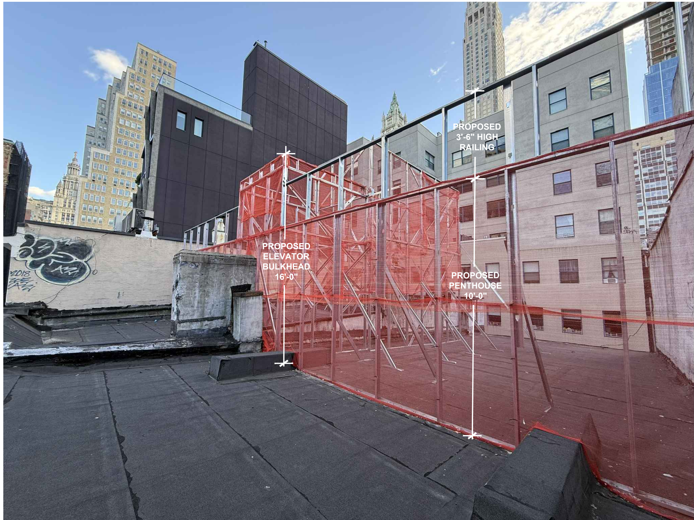
1 VIEW FROM FRONT OF ROOF - WITH MOCKUP
