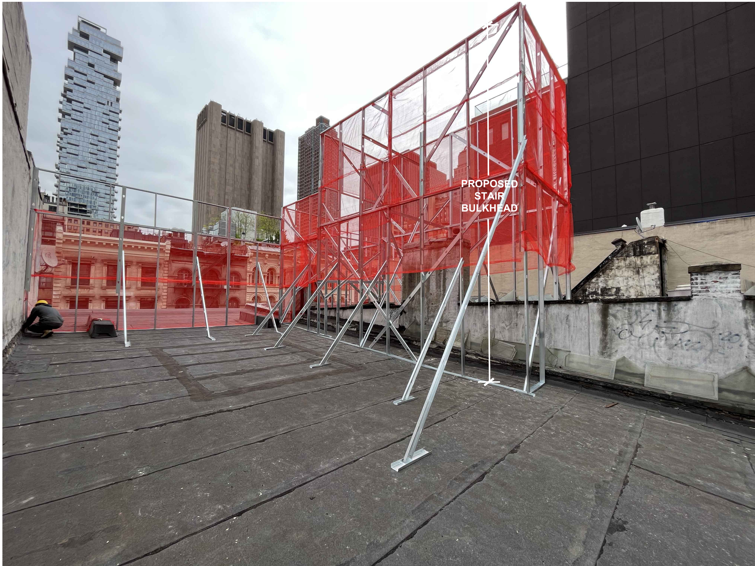
4 VIEW FROM BACK OF ROOF - WITH MOCKUP
