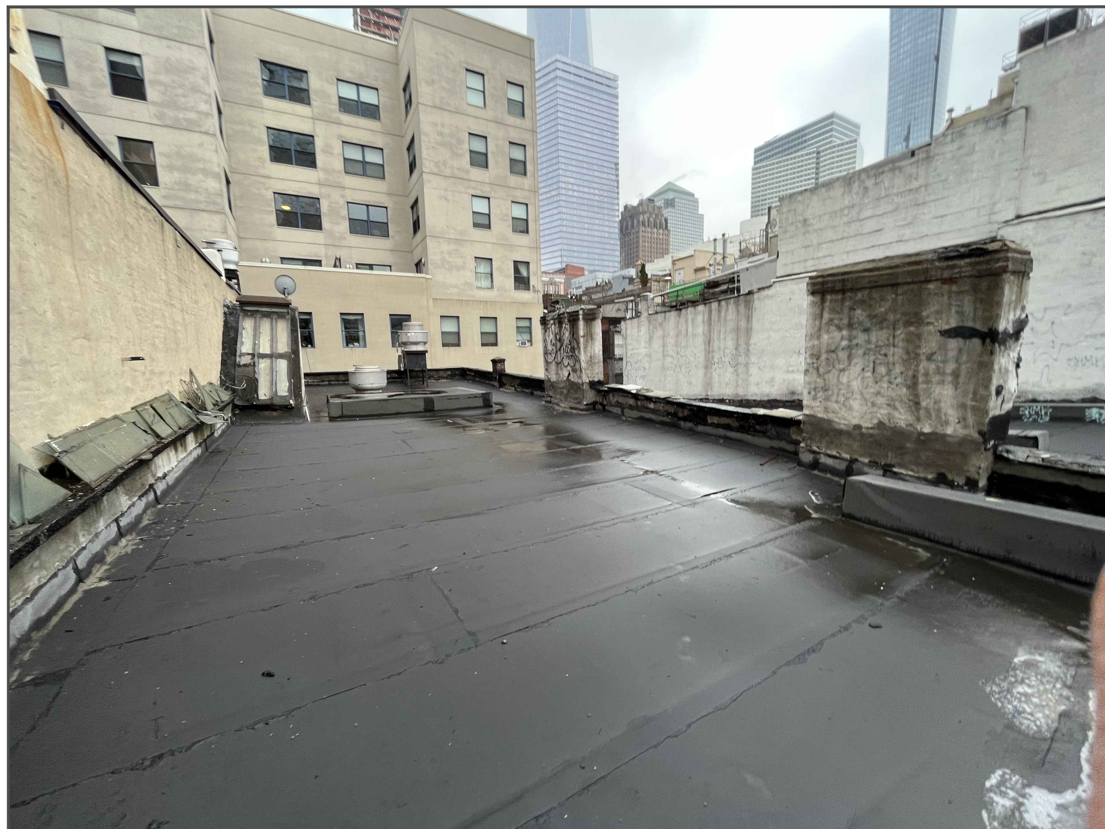
5 EXISTING ROOF OF 112 CHAMBERS ST
