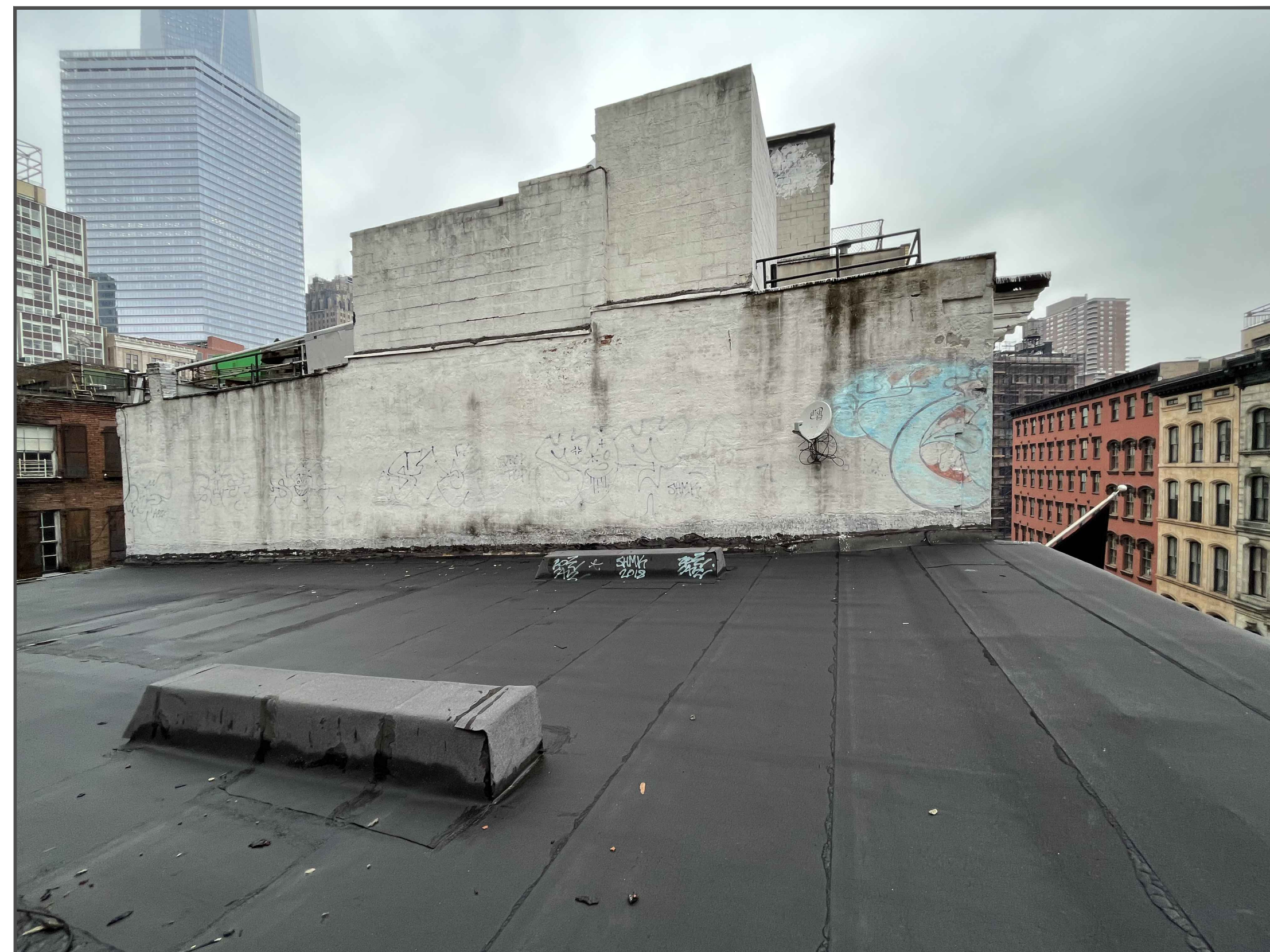
6 EXISTING ROOF OF 114 CHAMBERS ST
