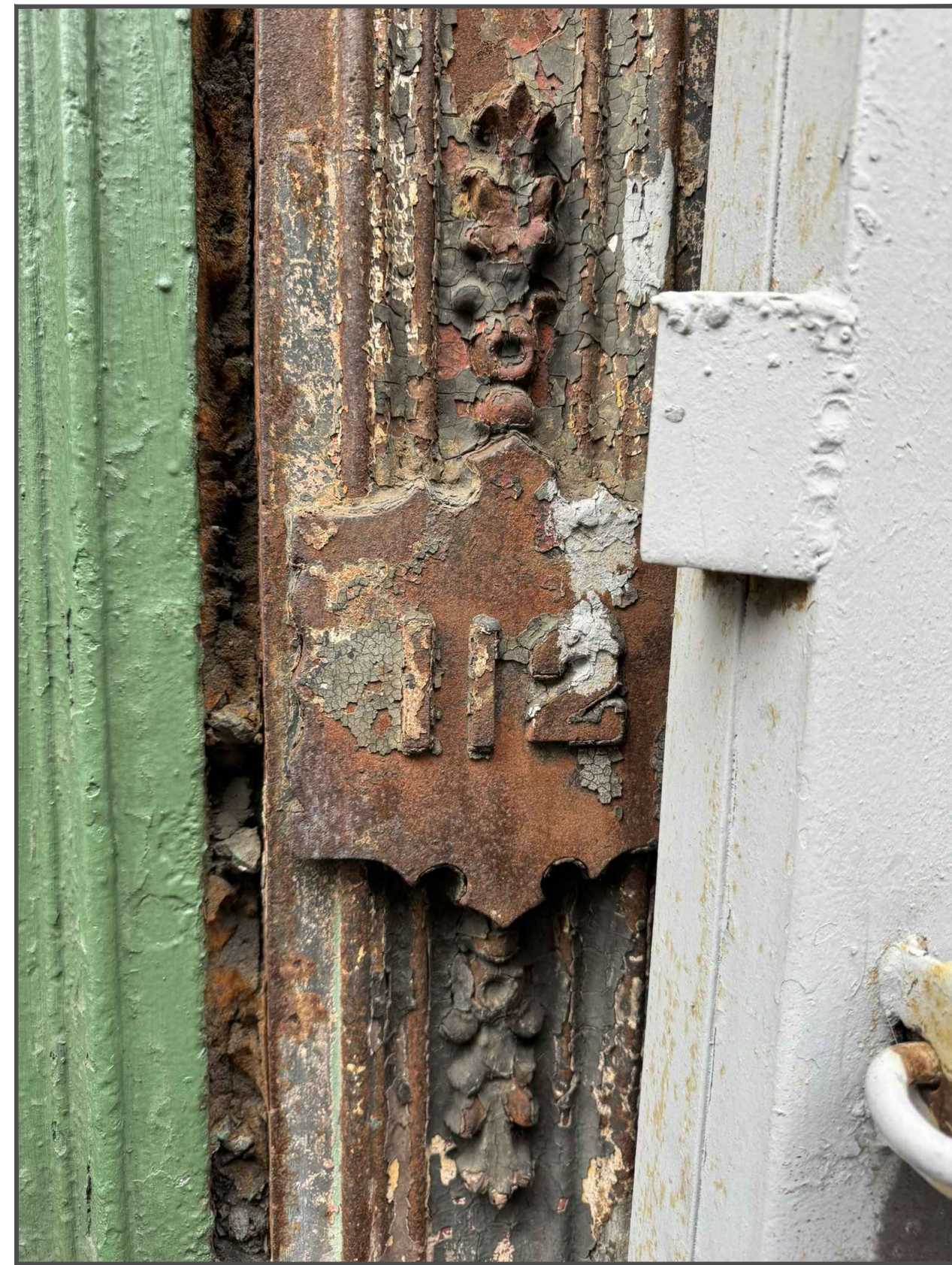
3 CAST IRON DETAIL AT 112 CHAMBERS ST
