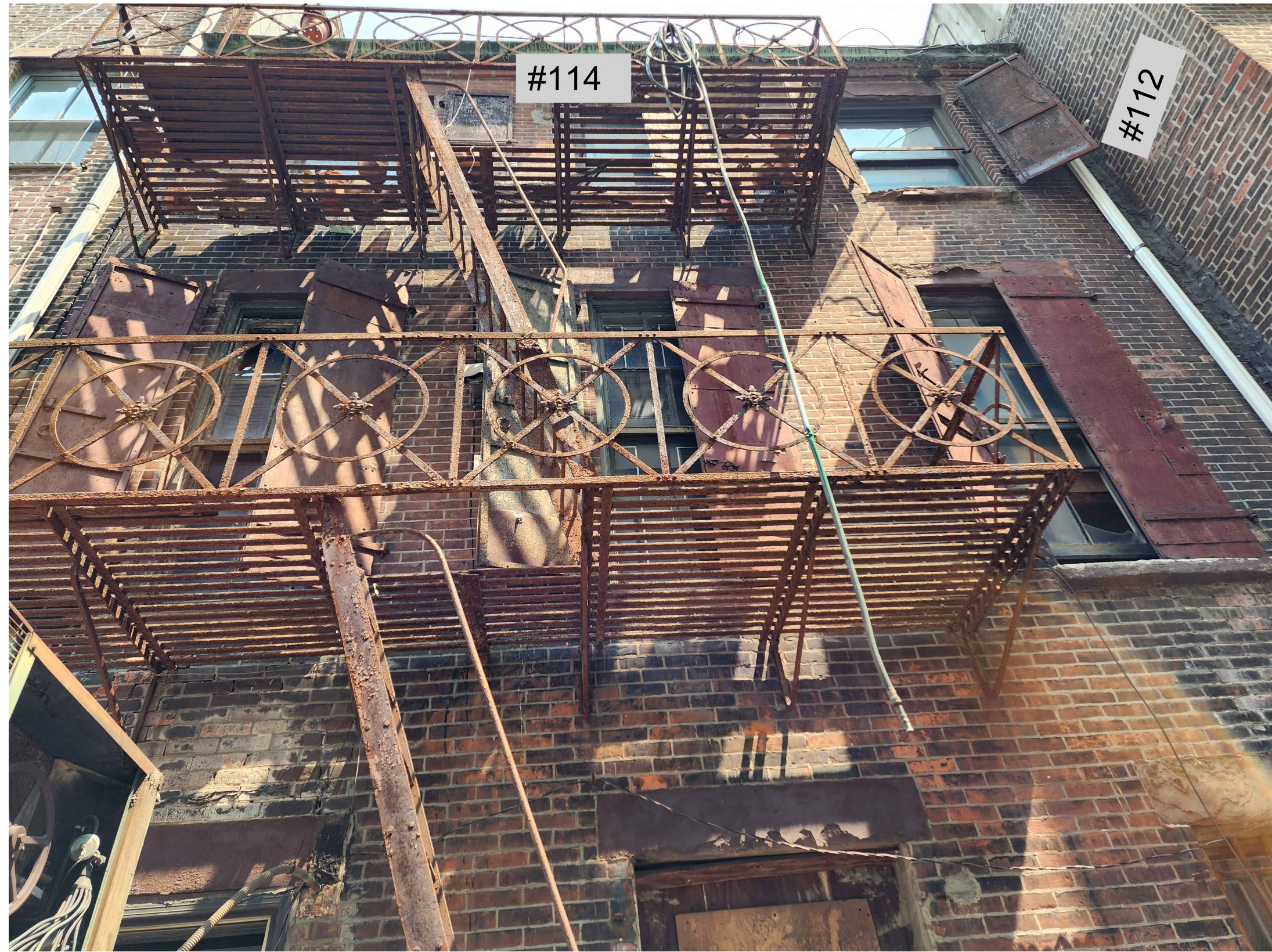
1 EXISTING REAR FACADE
