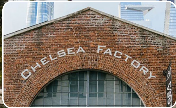
WEST 26TH STREET FACADE LPC-APPROVED PAINTED SIGN
