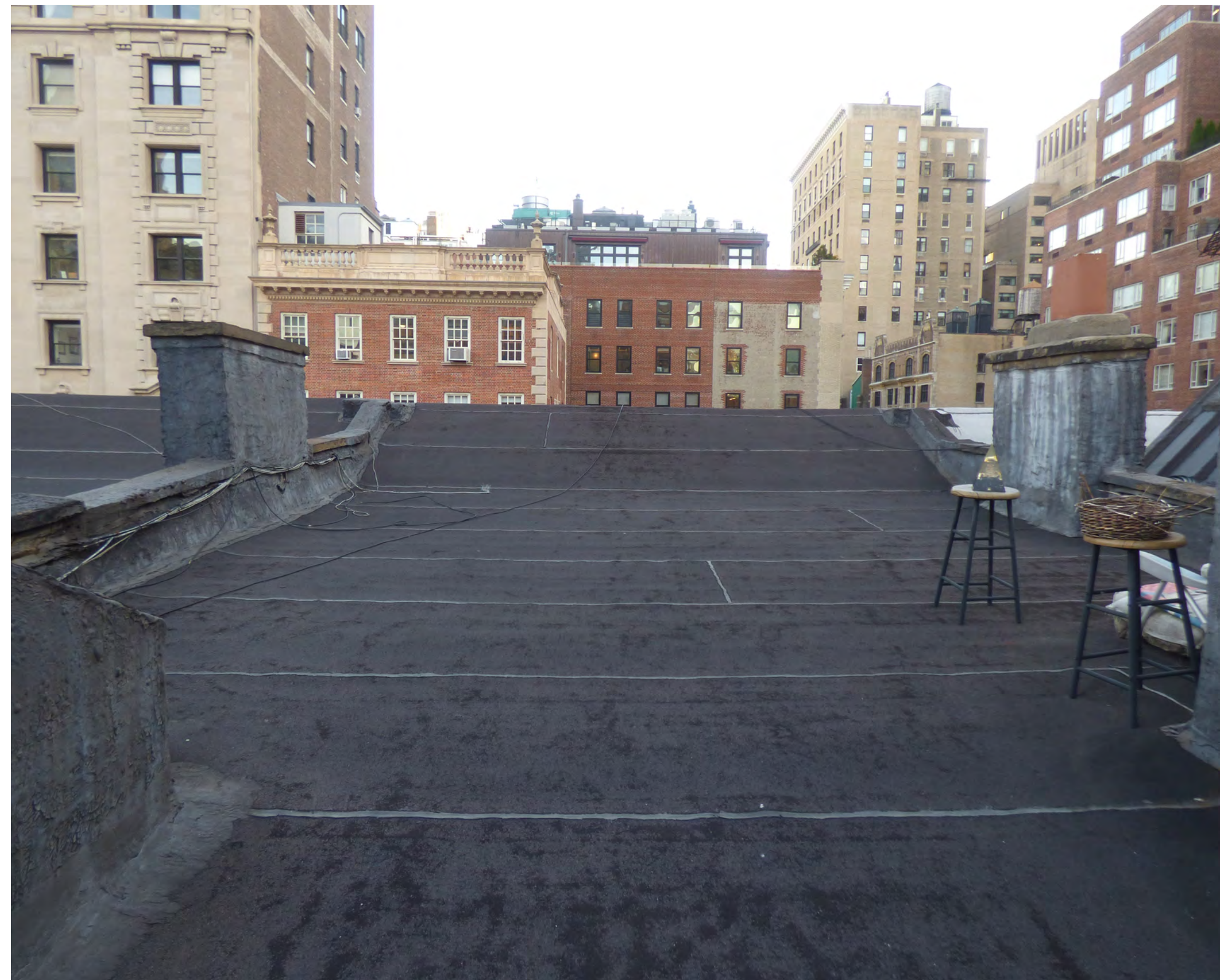
View of the roof looking east.
