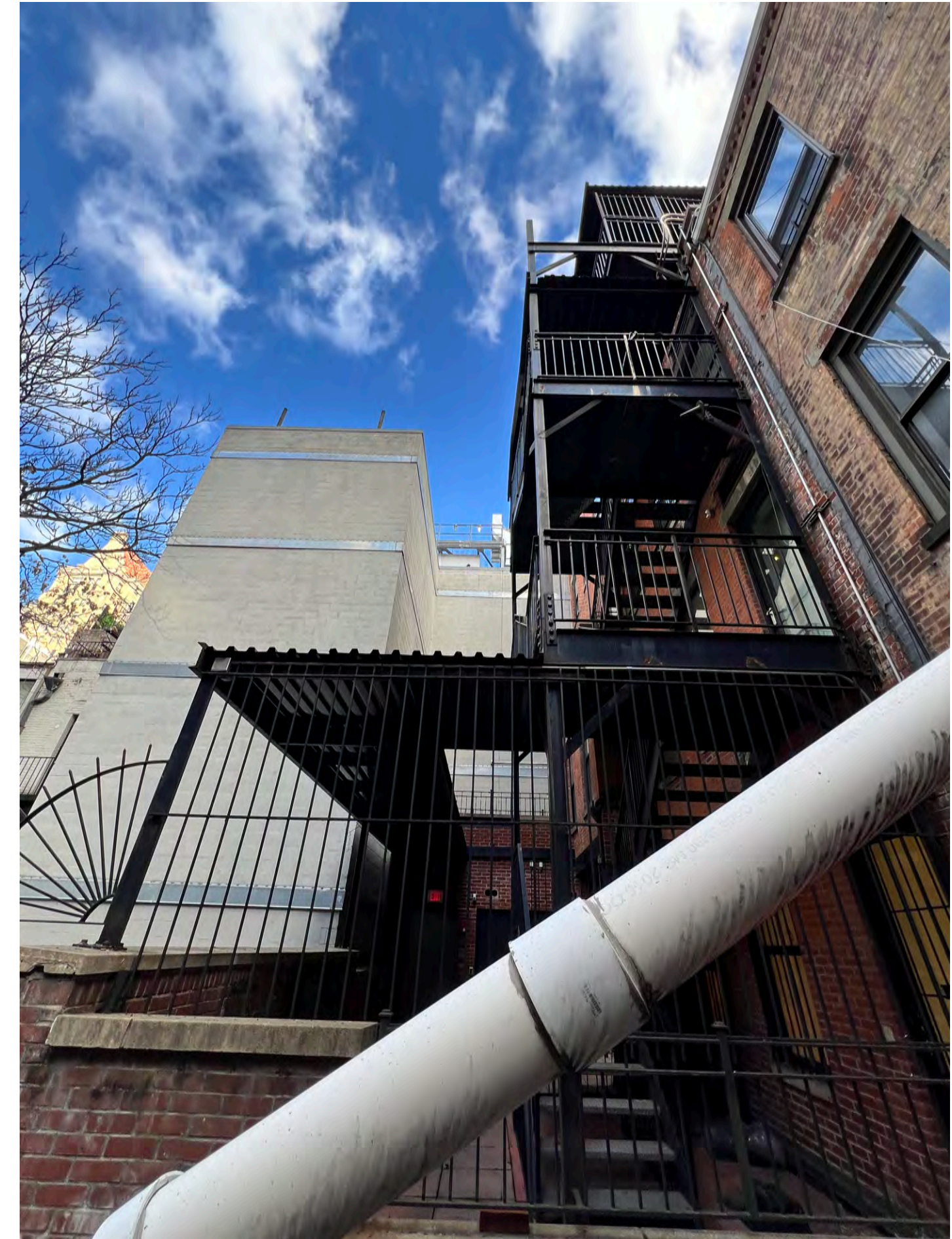
View of the rear yard (694 Madison Avenue)
