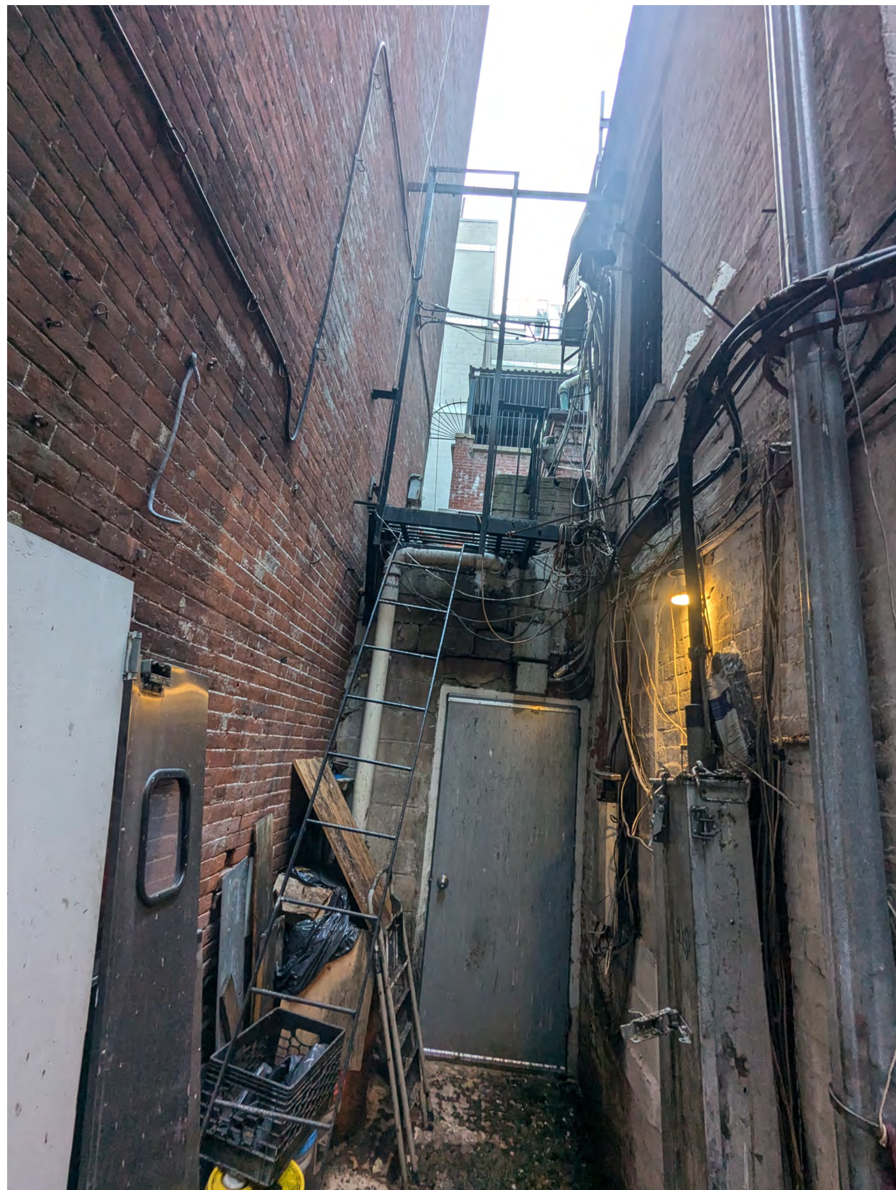
View looking north from the rear yard (towards 696-698 Madison Avenue)
