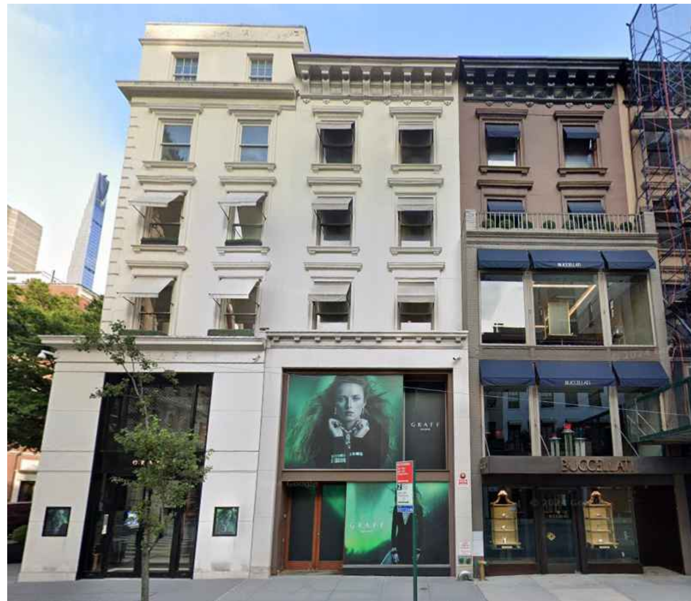
CONDITION @ 710-714 MADISON AVE. 3 NTS
