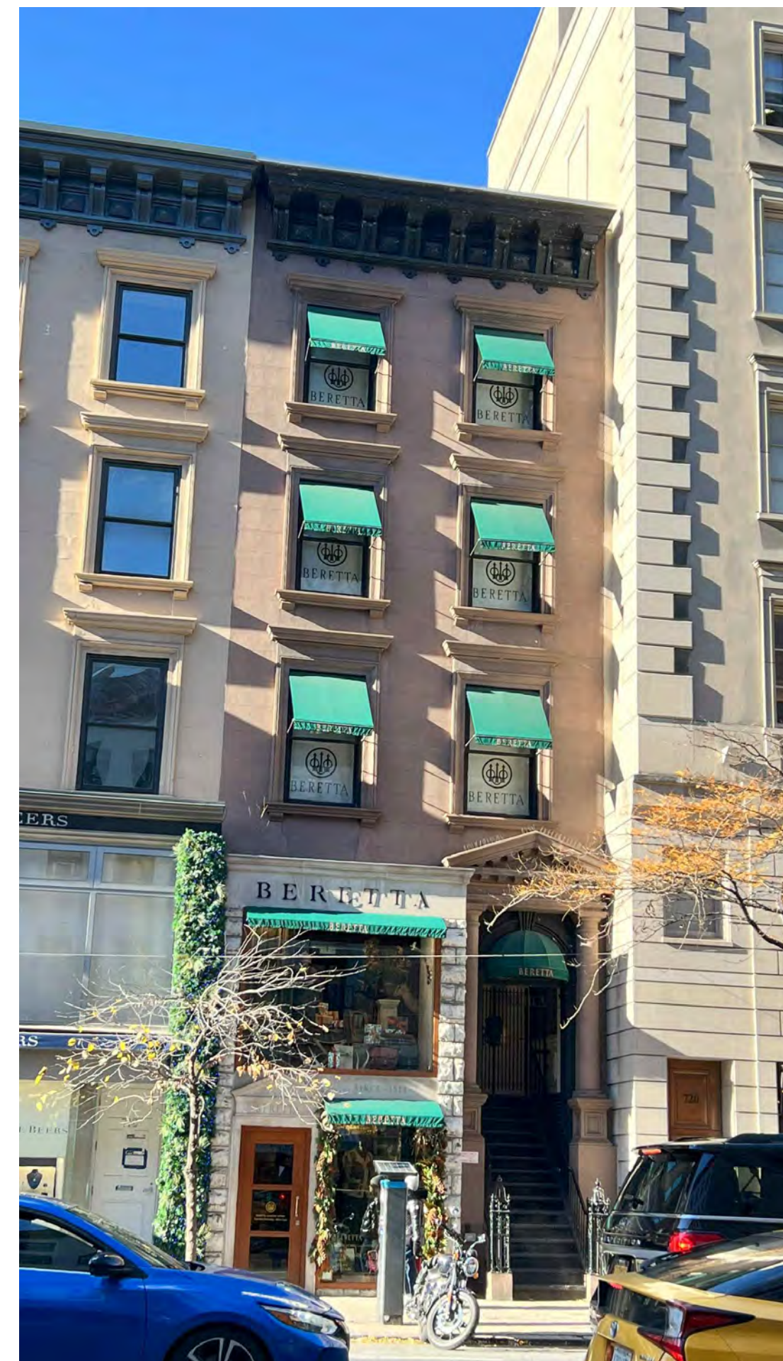
CONDITION @ 718 MADISON AVE. 1 NTS
