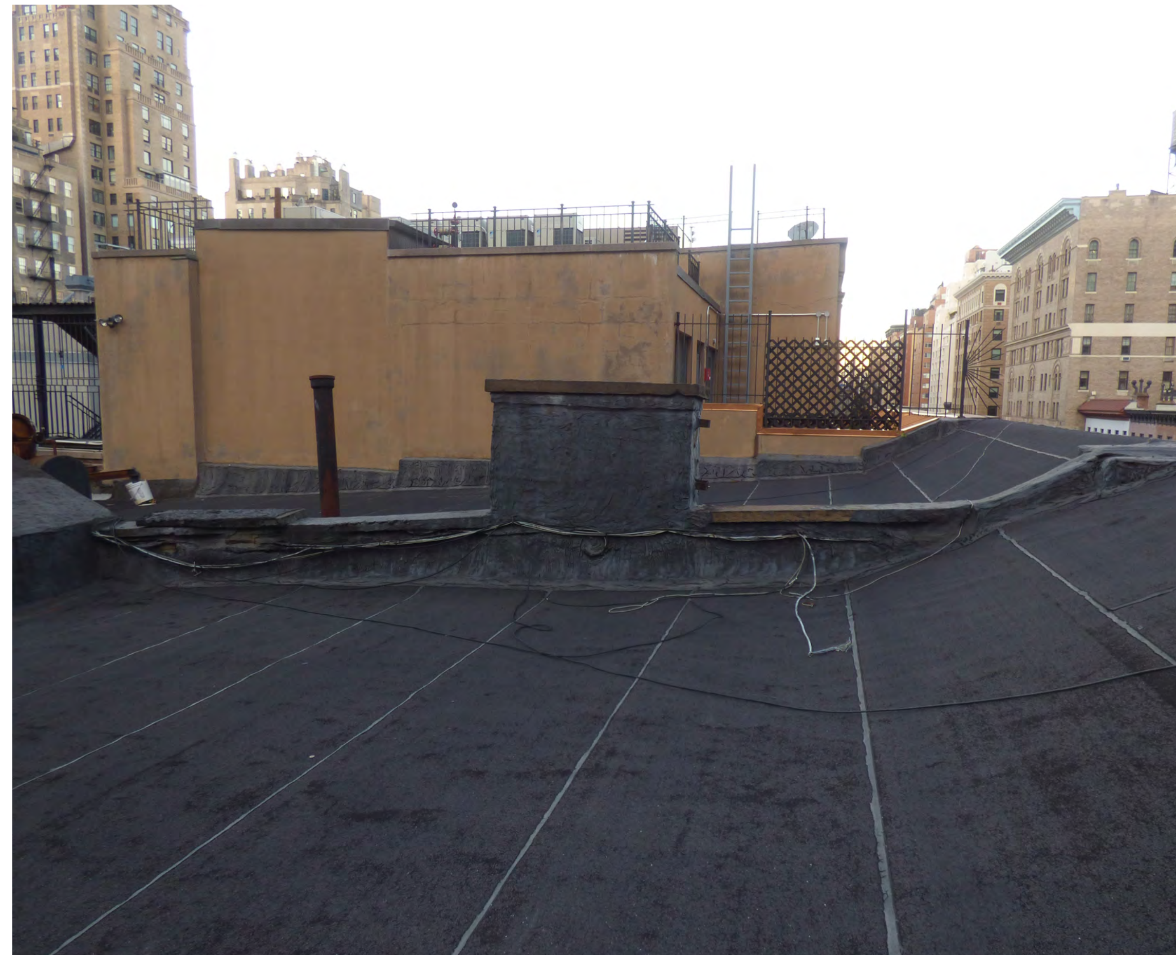
View of the roof looking north.
