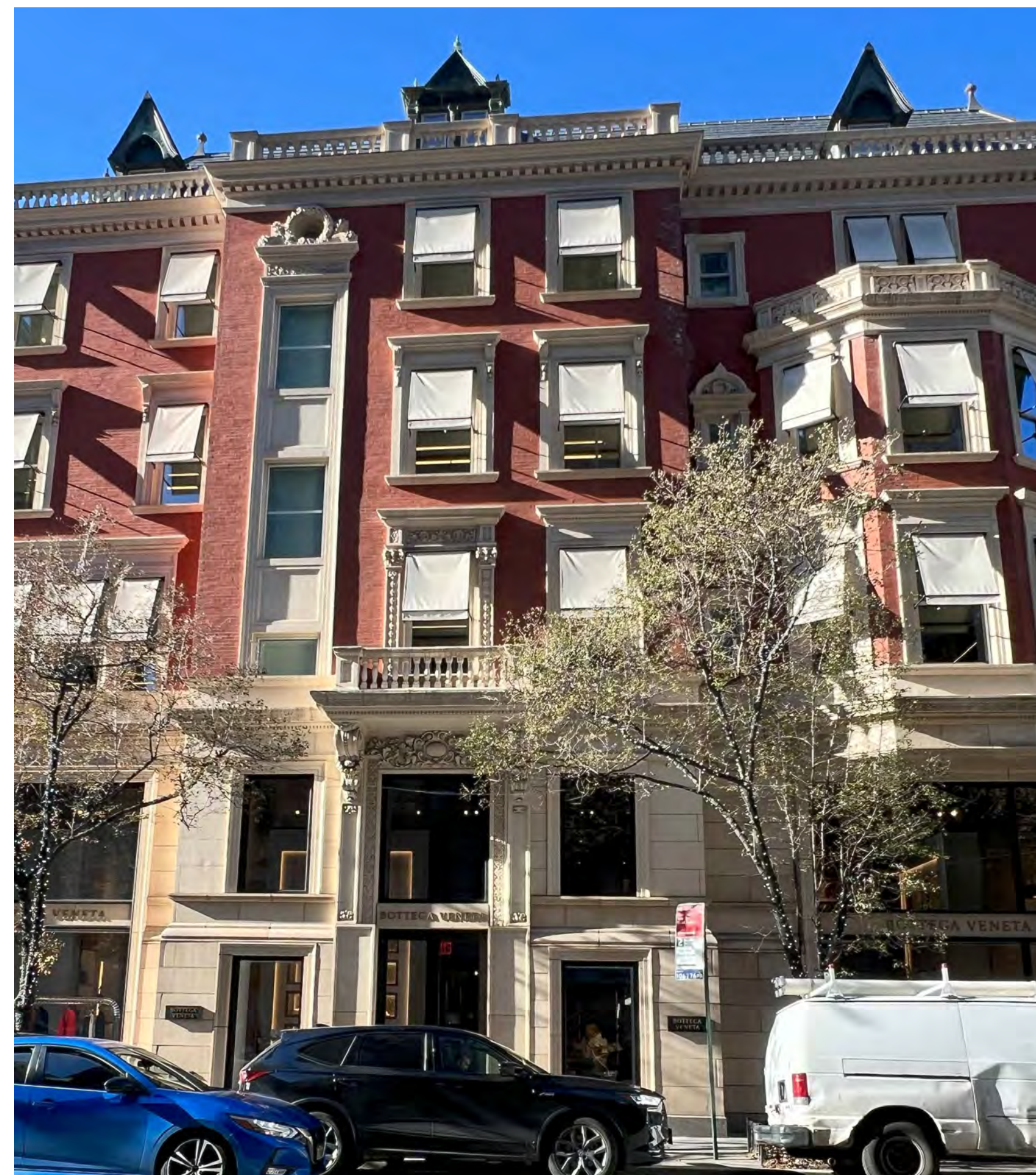
CONDITION @ 740 MADISON AVE. 3 NTS
