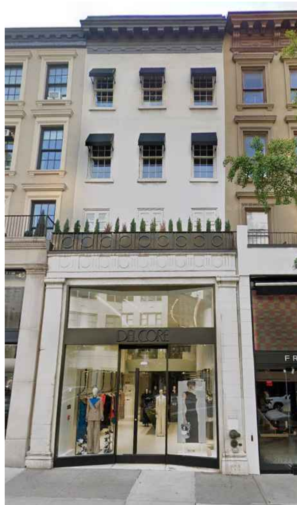
CONDITION @ 789 MADISON AVE. 3 NTS
