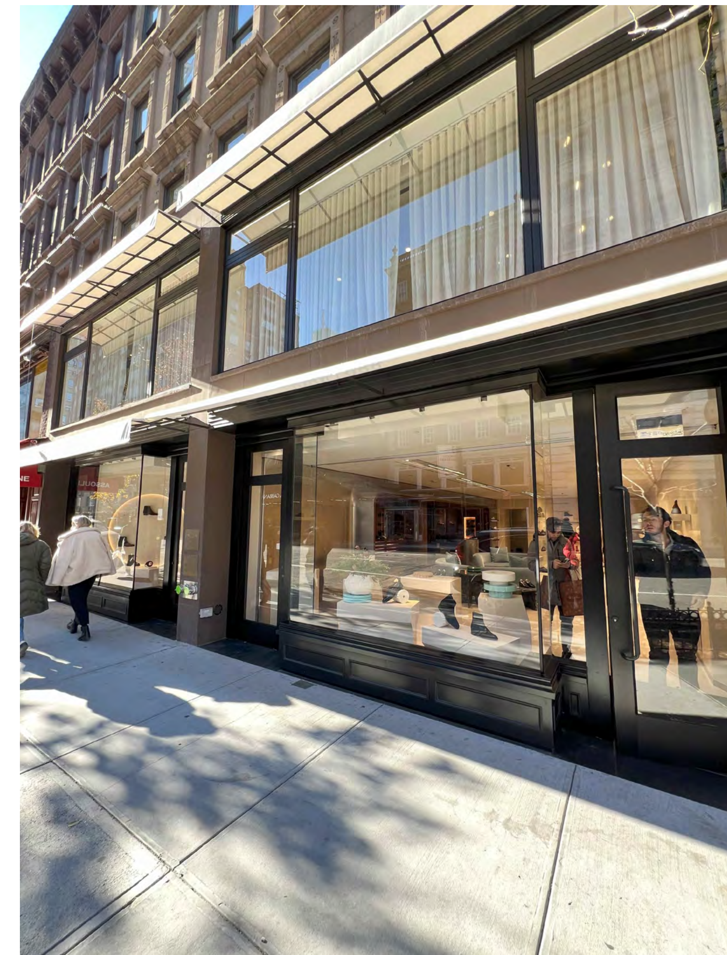
CONDITION @ 700 MADISON AVE. 1 NTS
