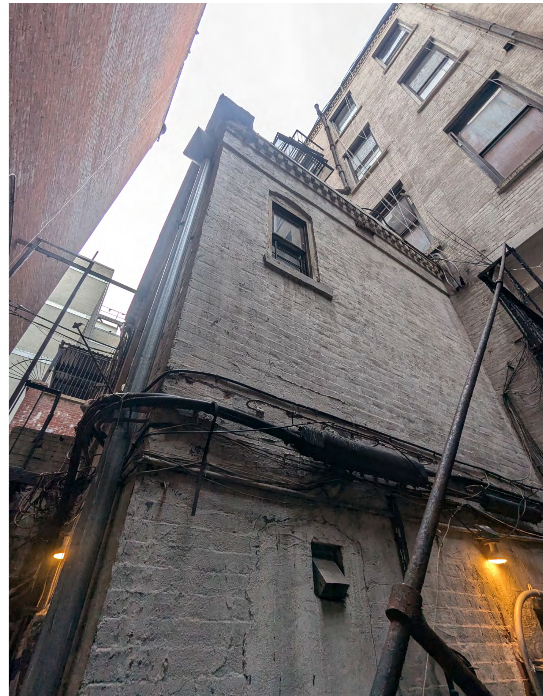
View of the rear yard (694 Madison Avenue)
