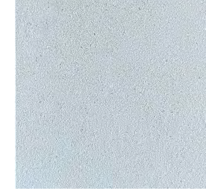
NEW GRAY PORTLAND STONE, JORDANS BASEBED, STONE SIGN SPANDREL.
