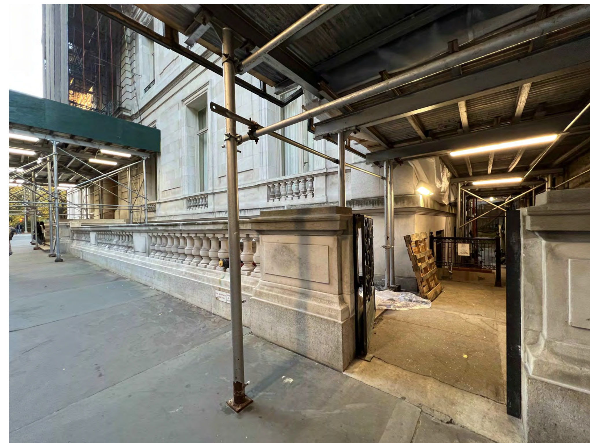
11 EXISTING EAST 78TH STREET VIEW FROM SIDEWALK NTS
