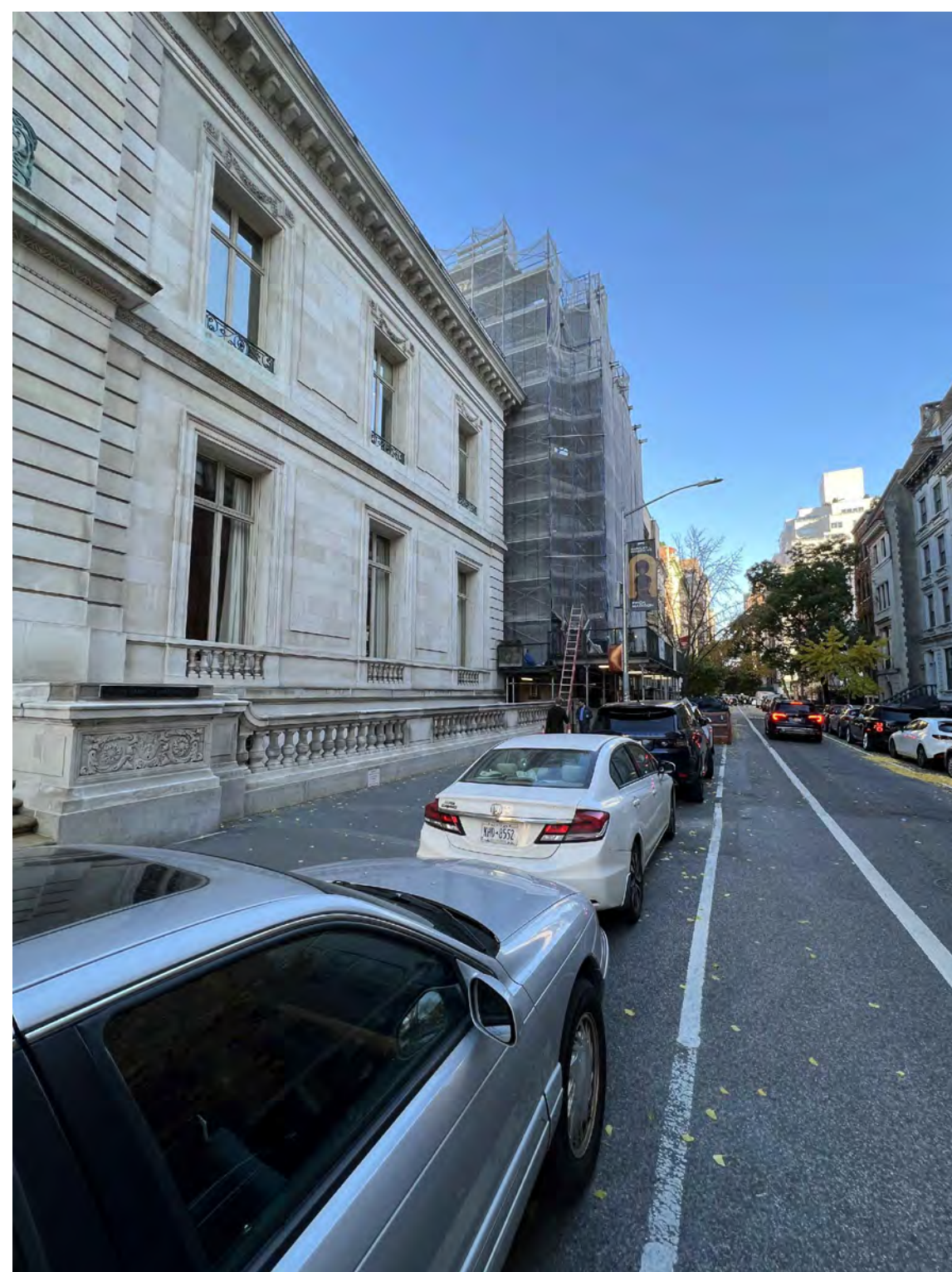
12 EXISTING EAST 78TH STREET VIEW FROM SIDEWALK NTS
