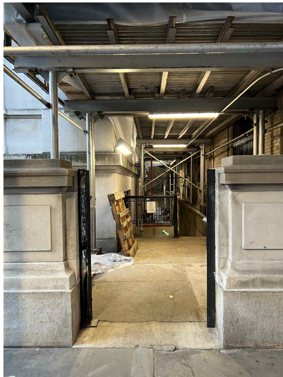
20 EXISTING EAST 78TH STREET VIEW FROM SIDEWALK NTS
