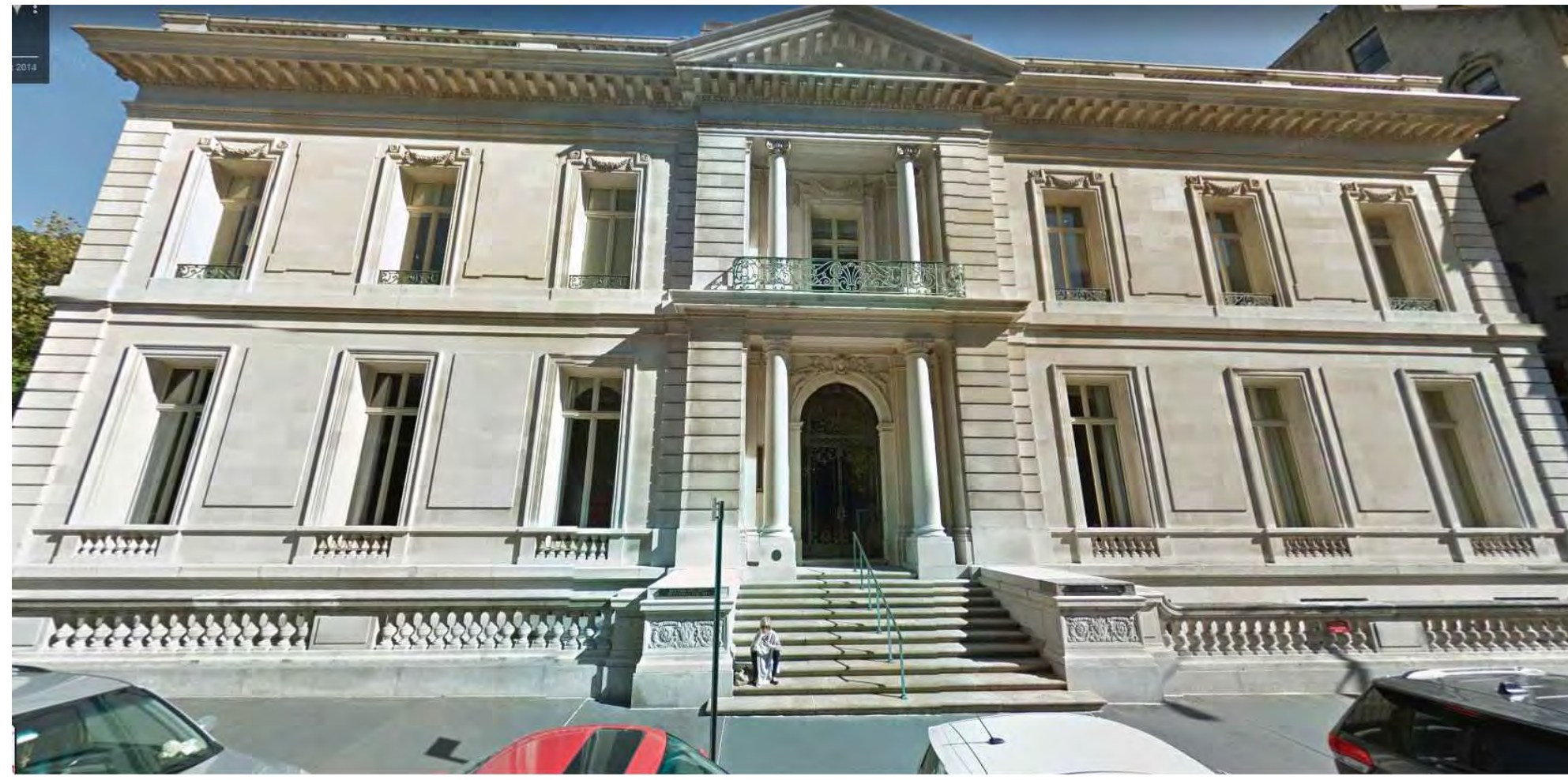
32 EXISTING NORTHERN VIEW OF FRONT FACADE NTS
