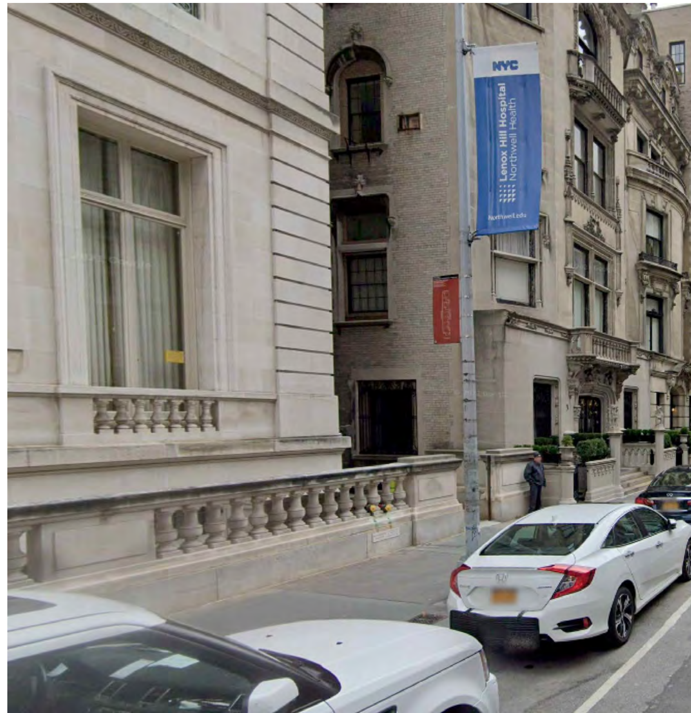
22 EAST 78TH GOOGLE STREET VIEW NTS (LPC REQUEST FOR NO SCAFFOLDING VISIBLE)
