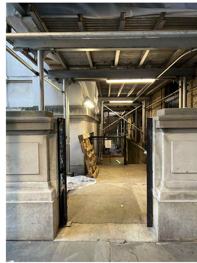
33 EXISTING VIEW FROM SIDEWALK NTS
