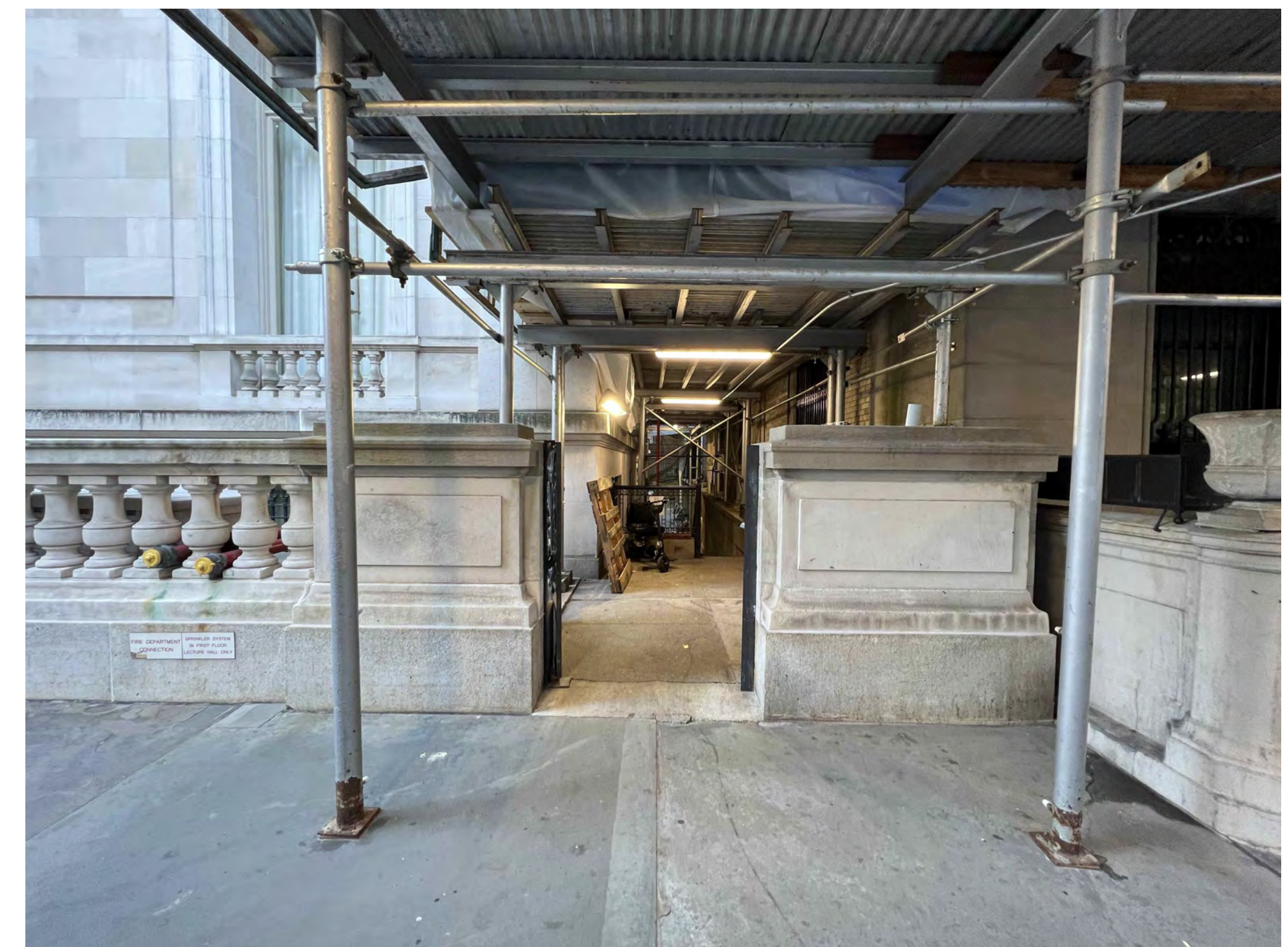
10 EXISTING EAST 78TH STREET VIEW FROM SIDEWALK NTS
