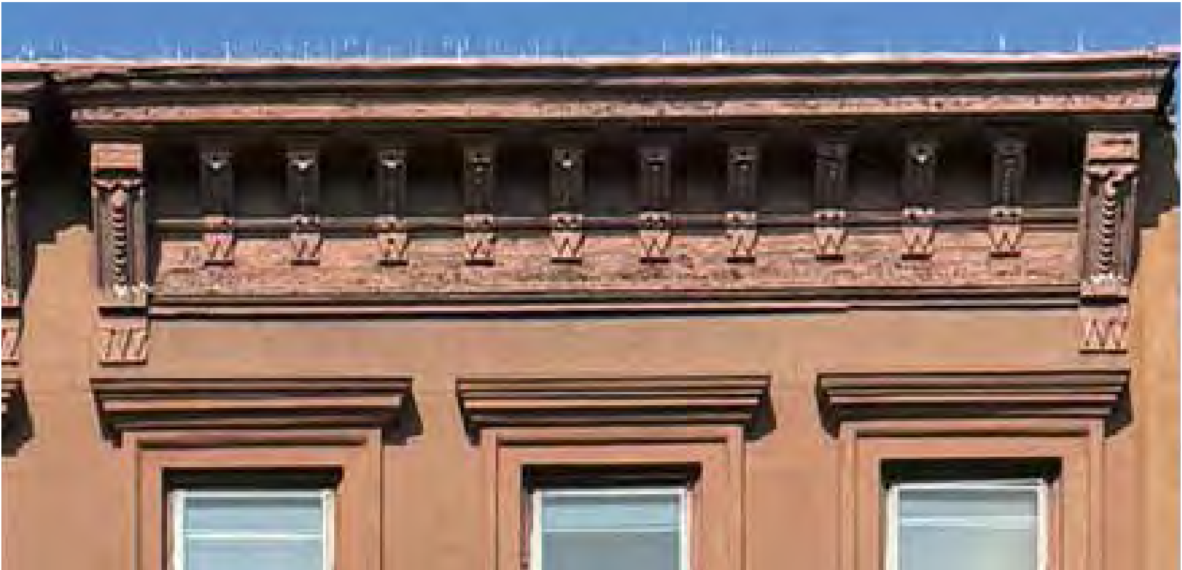
REFERENCE CORNICE: 30 7TH AVE CORNICE
