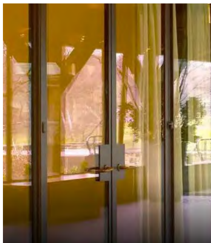
#4 HOPE'S - LANDMARK 175 STOREFRONT DOORS WITH SIDELIGHTS STEEL INSULATED WINDOWS PAINTED GREEN COLOR TO MATCH DECO BUILDING
