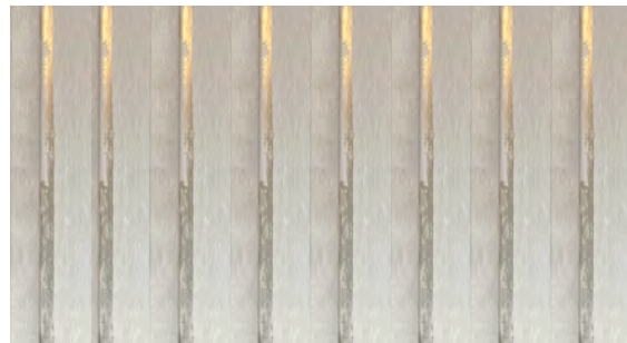
#3 ZINC SPANDREL PANELS FOLDED TO ALLUDE TO ORIGINAL RIBBED SPANDREL PANELS ON 23RD STREET
