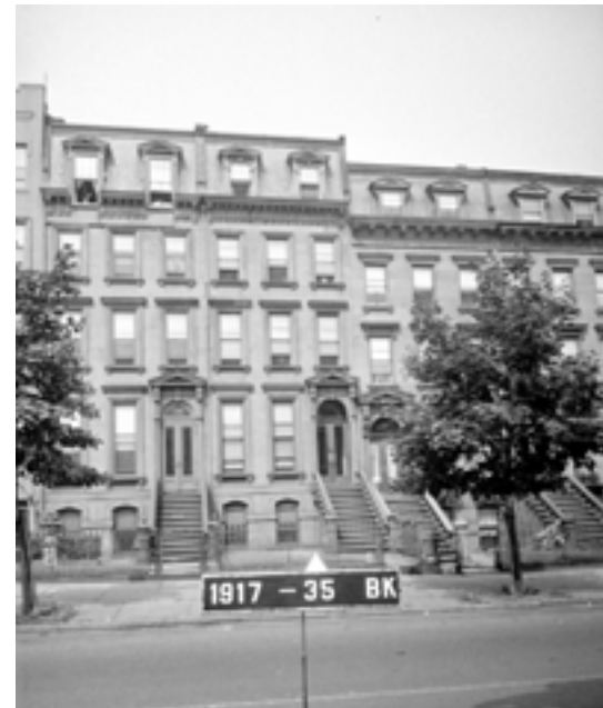
240 WASHINGTON AVENUE - ROWHOUSE
