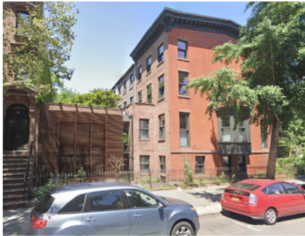
228 WASHINGTON AVENUE (APPROVED AND COMPLETED CLINTON HILL LANDMARKS)
