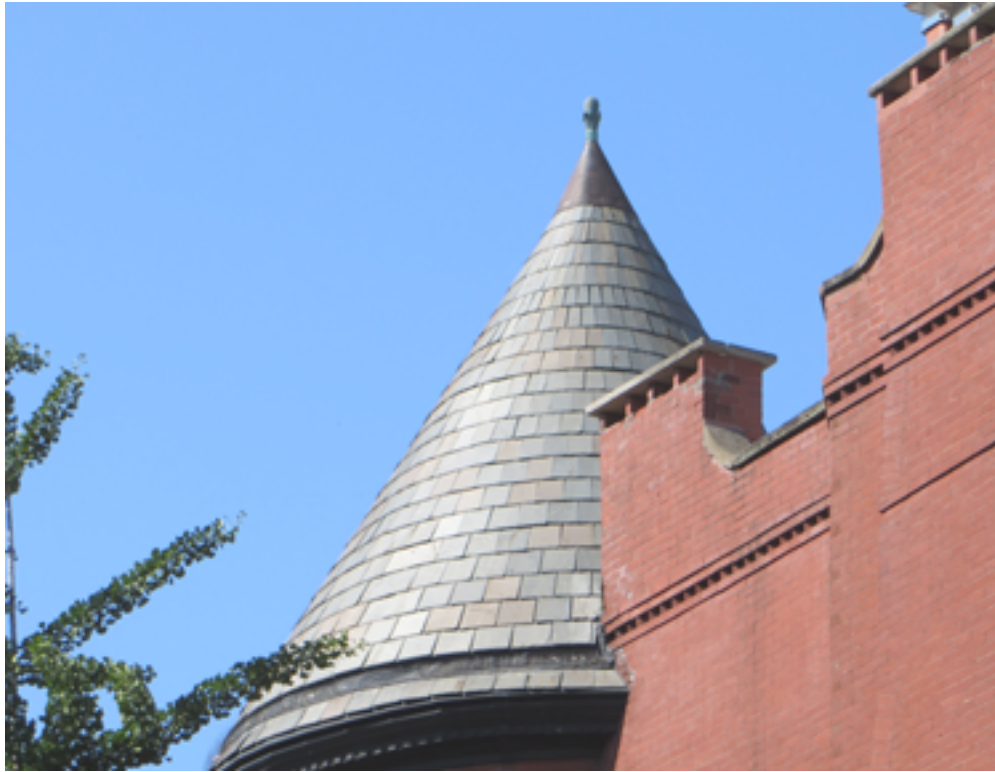
SLATE TILE SHINGLED ROOFING ( 289 DEKALB AVE )
