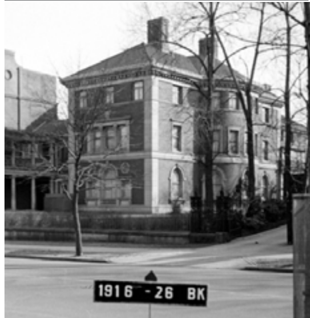
229 CLINTON AVENUE - MANSION
