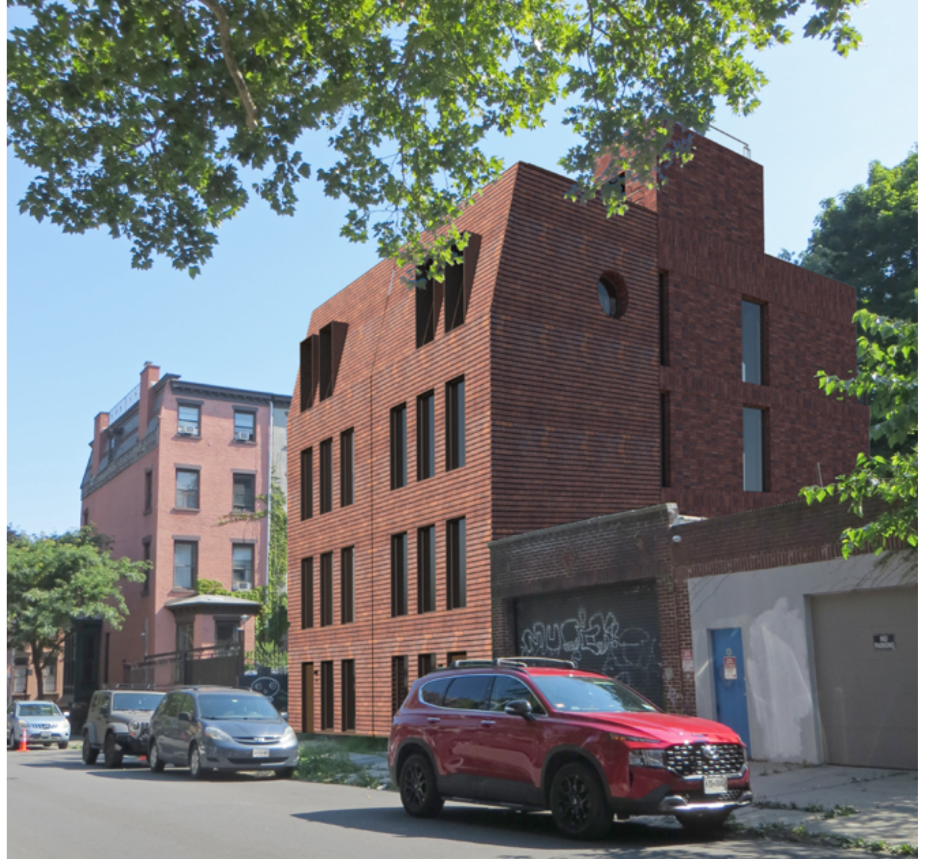
VIEW B LOOKING NORTHEAST
