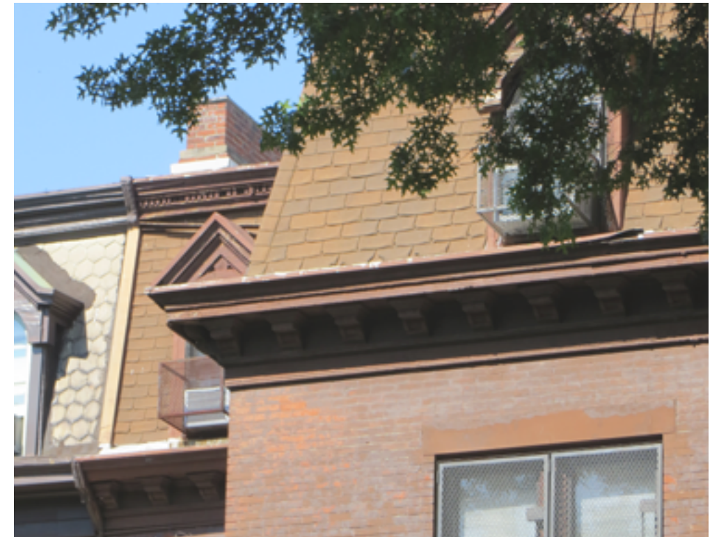
FACADE COLORATION ( 252 WAVERLY AVENUE )
