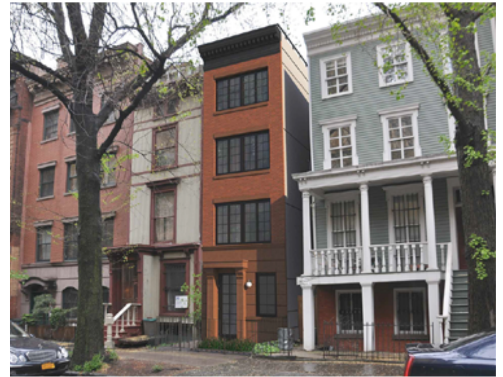
39 SOUTH ELLIOT PLACE (APPROVED & UNDER CONSTRUCTION FORT GREENE LANDMARKS)
