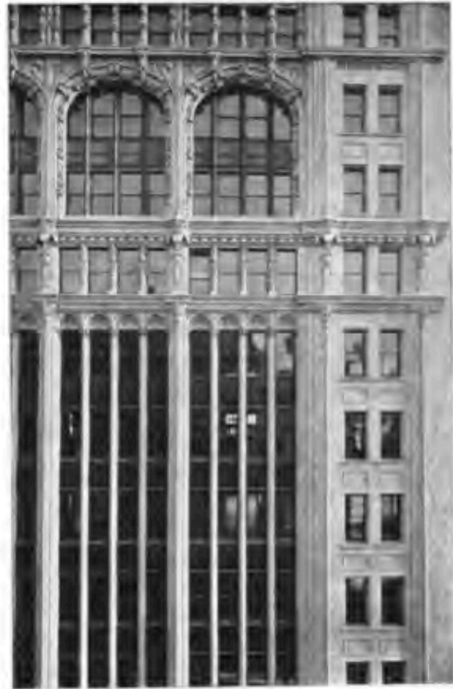
DETAIL of terra cotta facade, Emmett Building, Madison Avenue and 29th Street, New York City. J. Stewart Barney and Stockton B. Coll, Architects.
