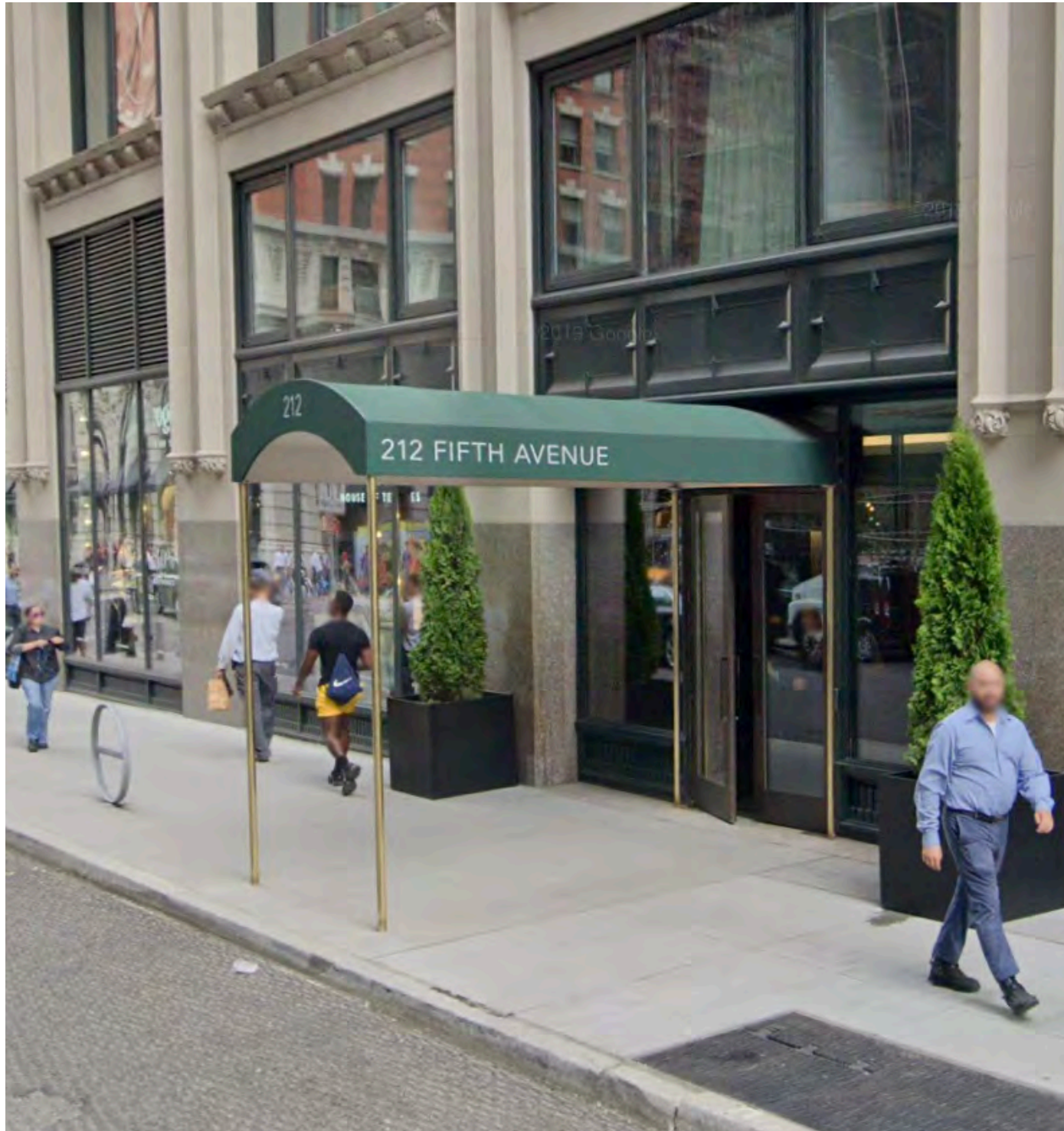
212 Fifth Avenue (Schwartz & Gross, 1913) in the Madison Square North HD. Canopy approved by LPC in 2015.
