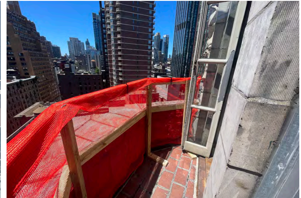
Guardrail at 16th Fl. SW Corner
