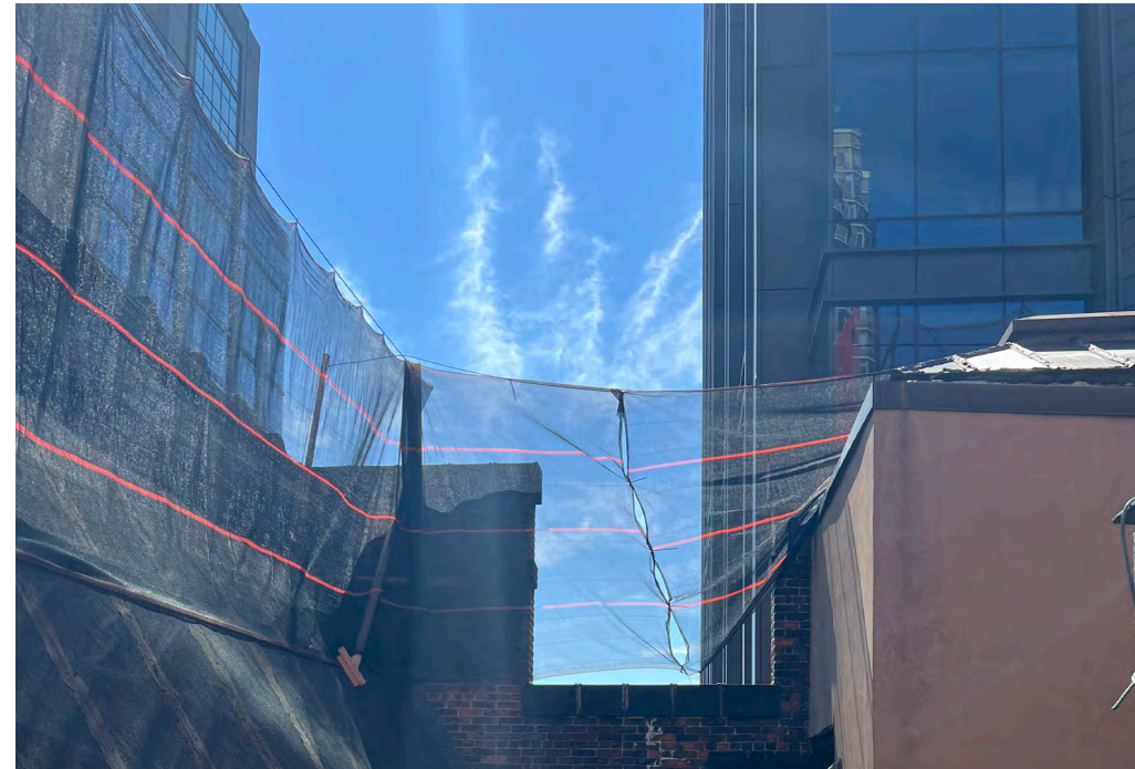
Guardrail at East
