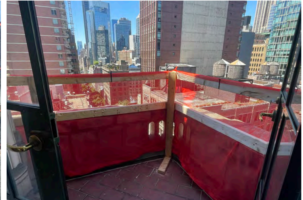
Guardrail at 16th Fl. NW Corner
