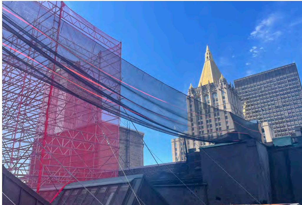
Guardrail at West
